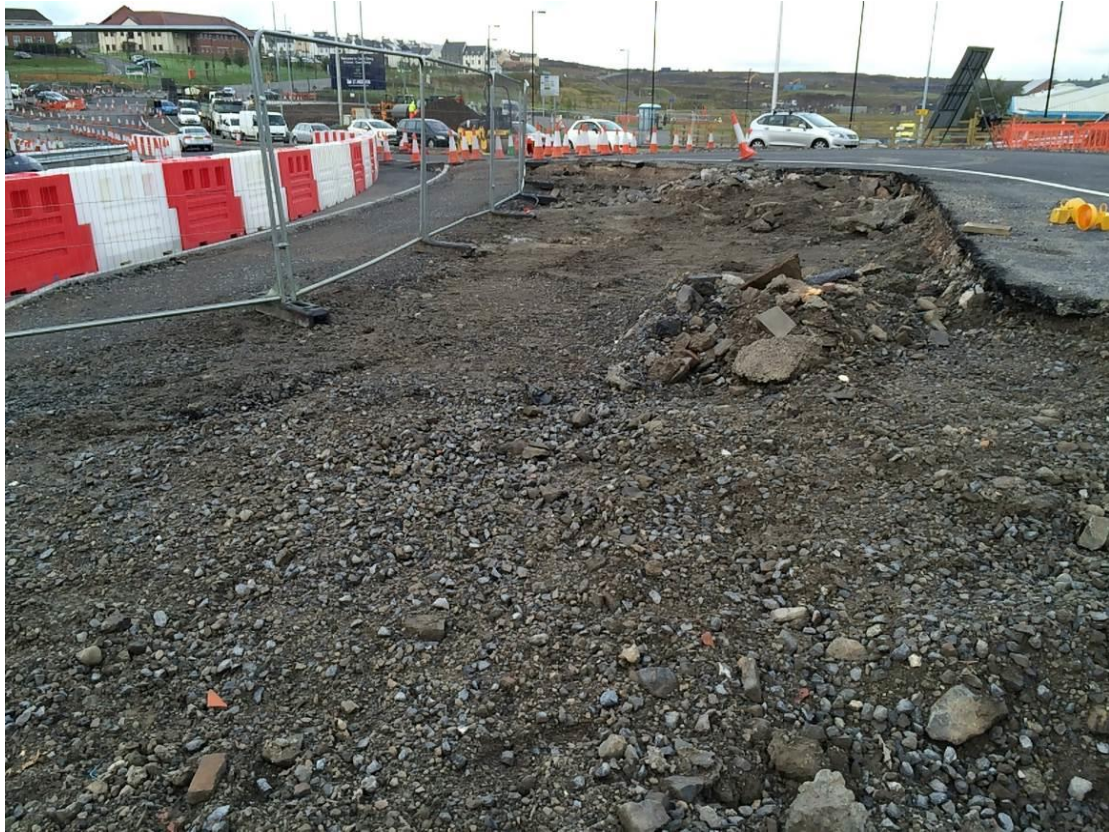
Photograph 11 – Looking southwest towards the Coed Darcy Village junction.
