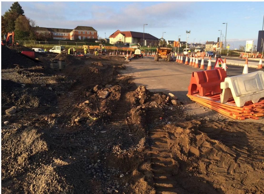
Photograph 12 – Looking southwest towards the Coed Darcy Village junction.
