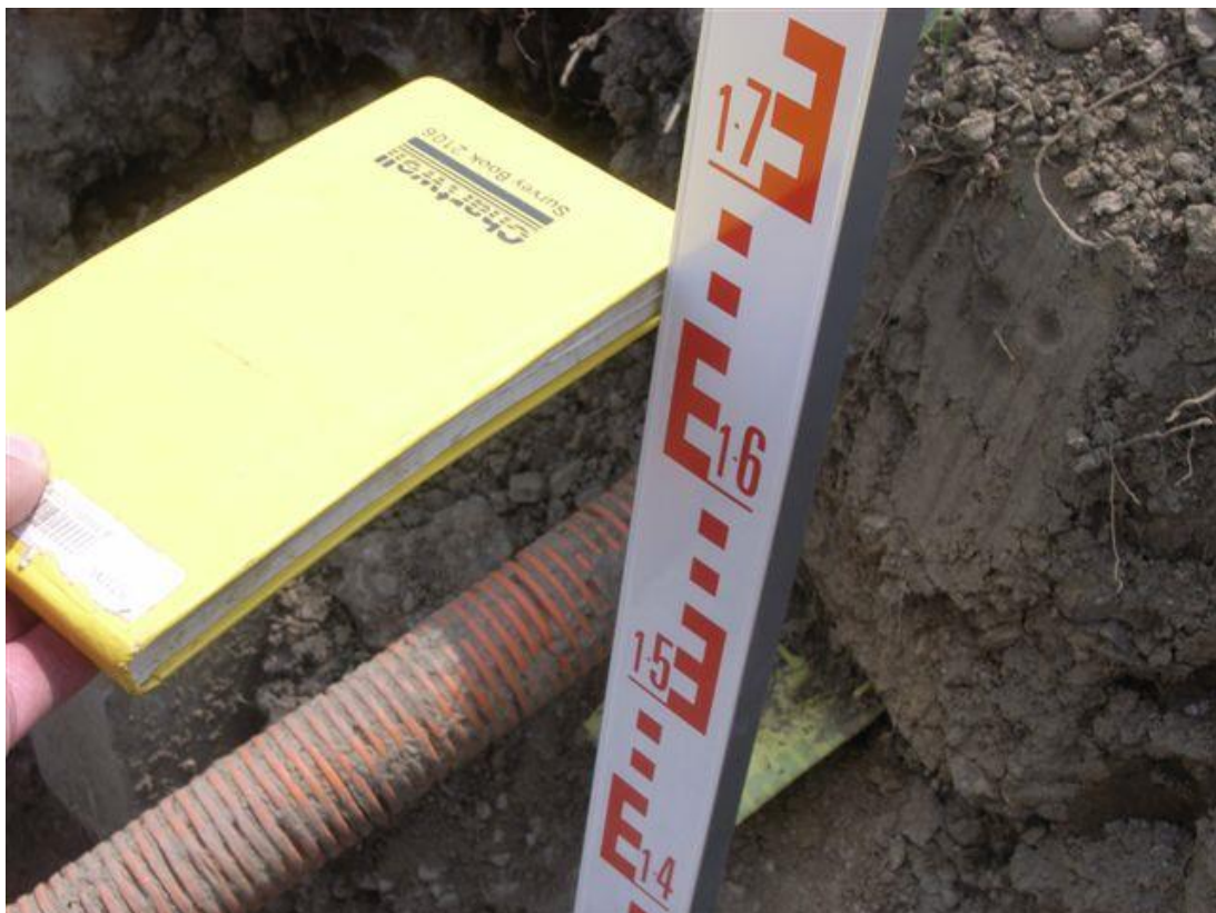
Photograph 4: Depth to recorded gas main
