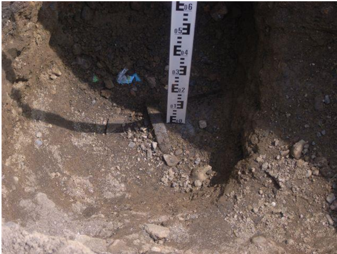
Photograph 7: Base of open trench
