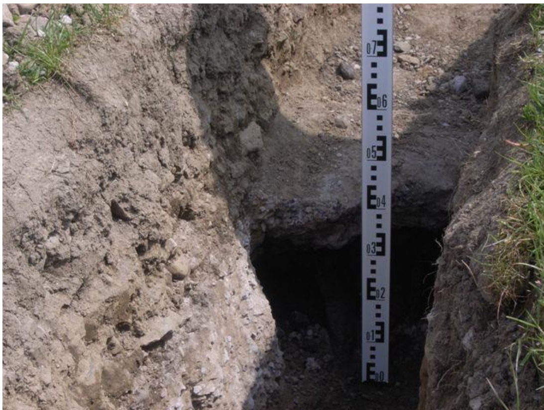
Photograph 10: Depth to base of excavations near to main
