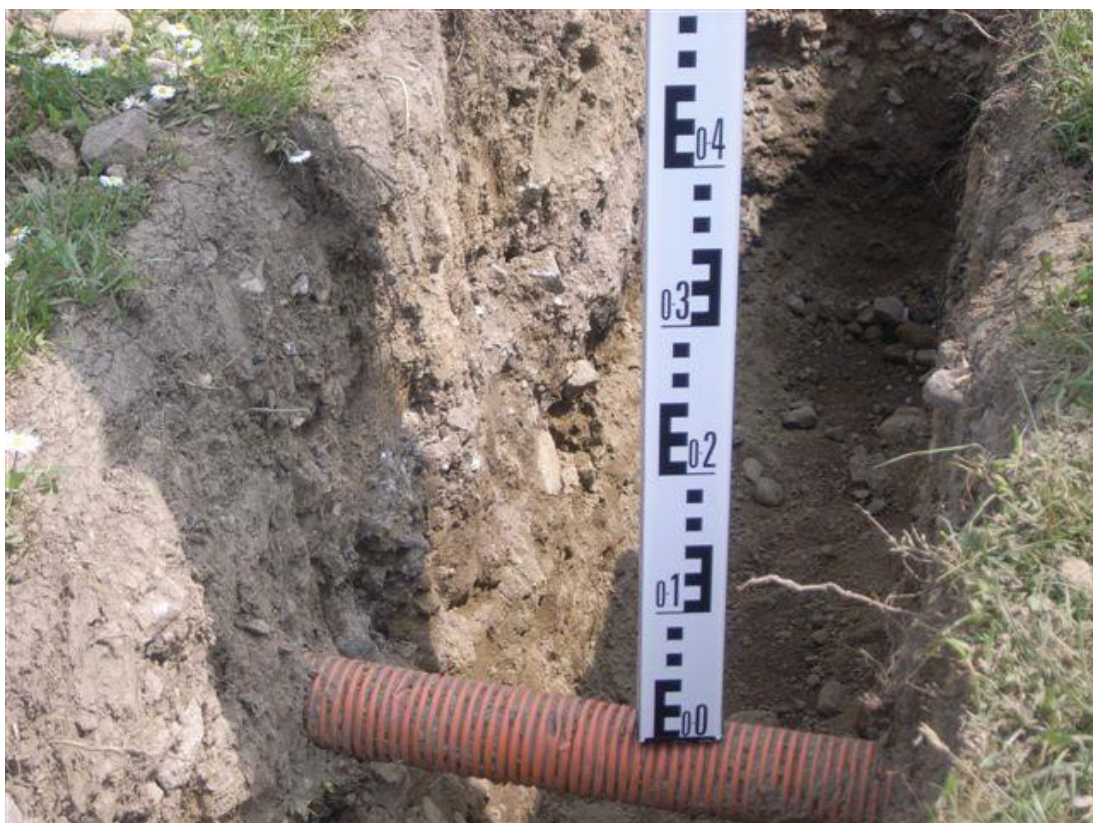
Photograph 8: Depth of identified street lighting
