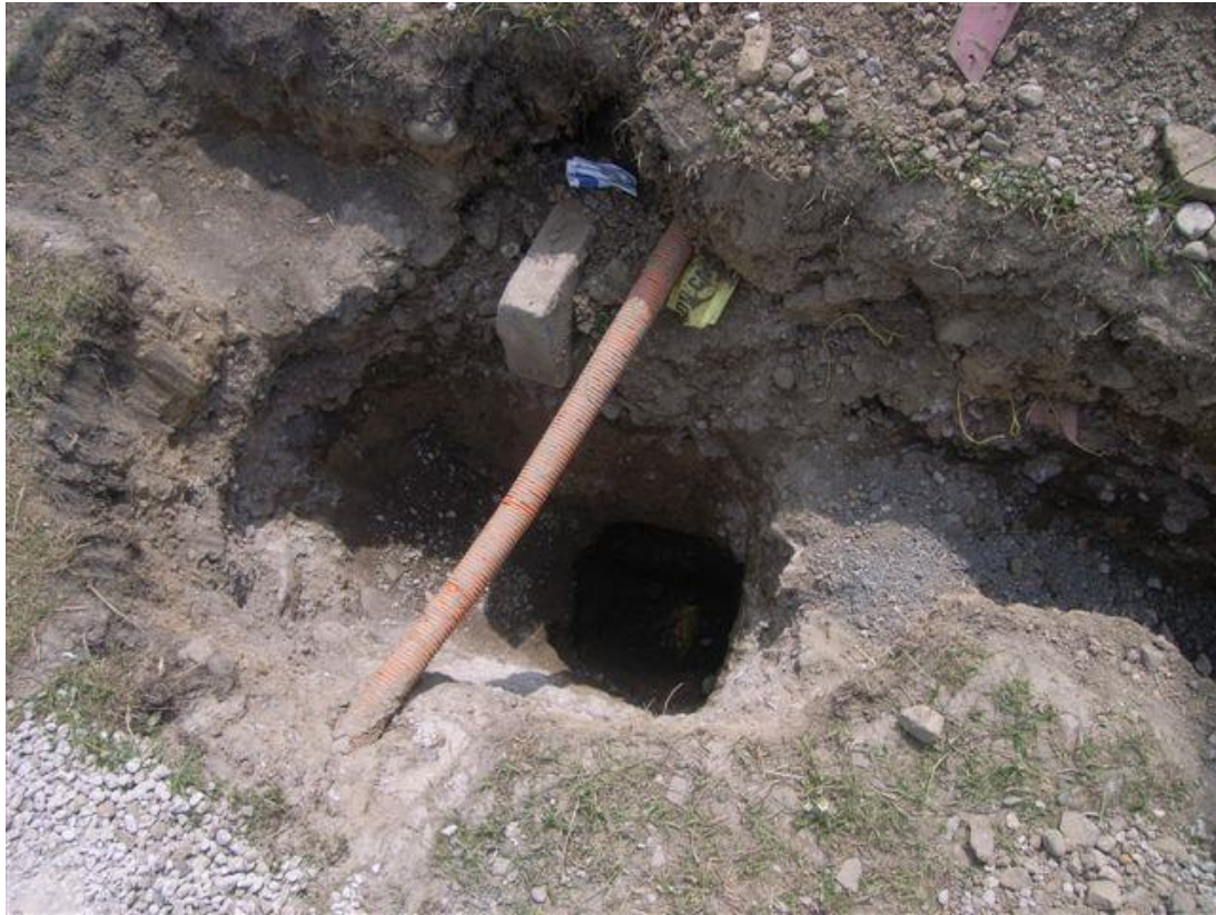
Photograph 1 : Street lighting with gas main underneath
