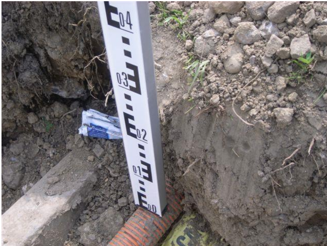
Photograph 5: Depth to street lighting
