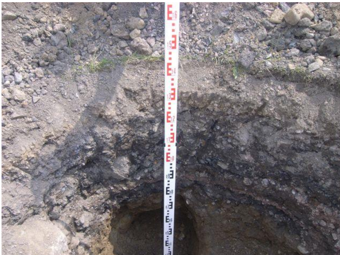
Photograph 6: Cast iron main
