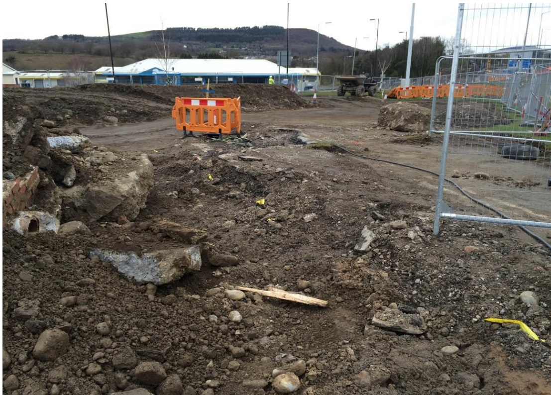
Photograph 4 – Looking northwest towards Darcy Business park.
