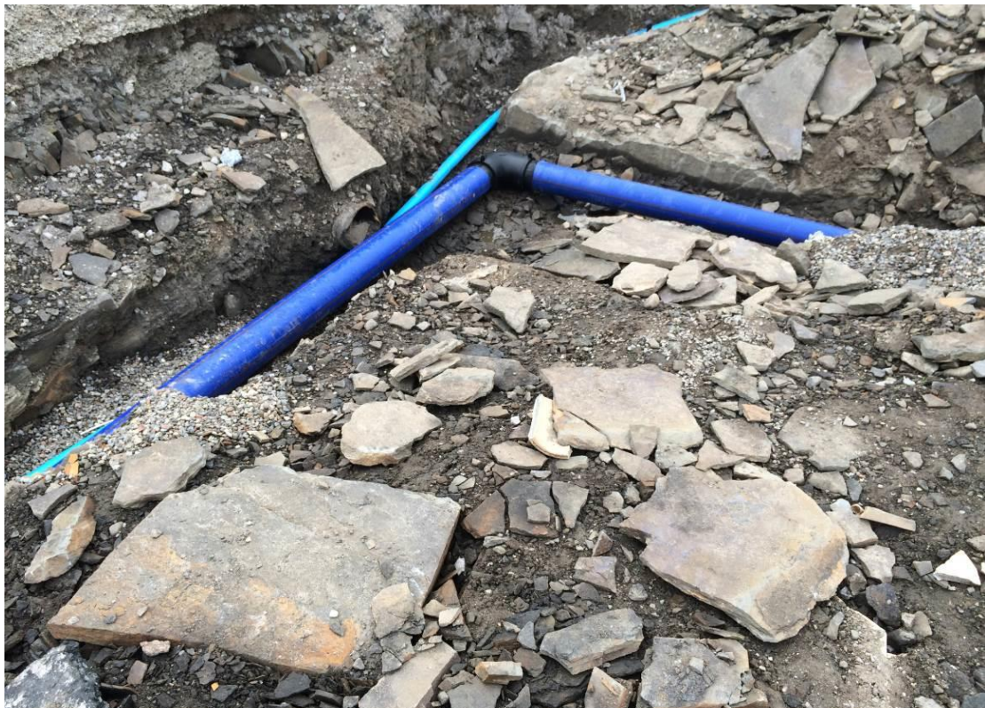
Photograph 8 – Looking at the newly installed water main, note the shallow depth to bedrock.
