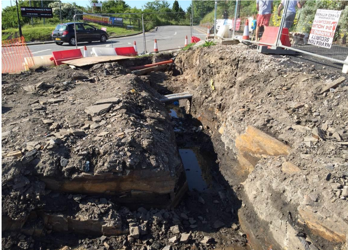
Photograph 7 – Looking southeast along the B4290, note the shallow depth to bedrock.
