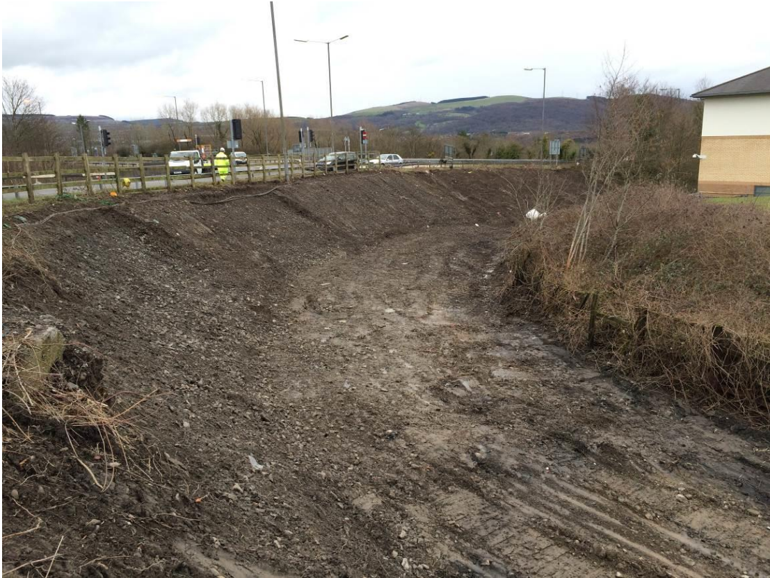
Photograph 1 – Looking east over bank improvement ground works.
