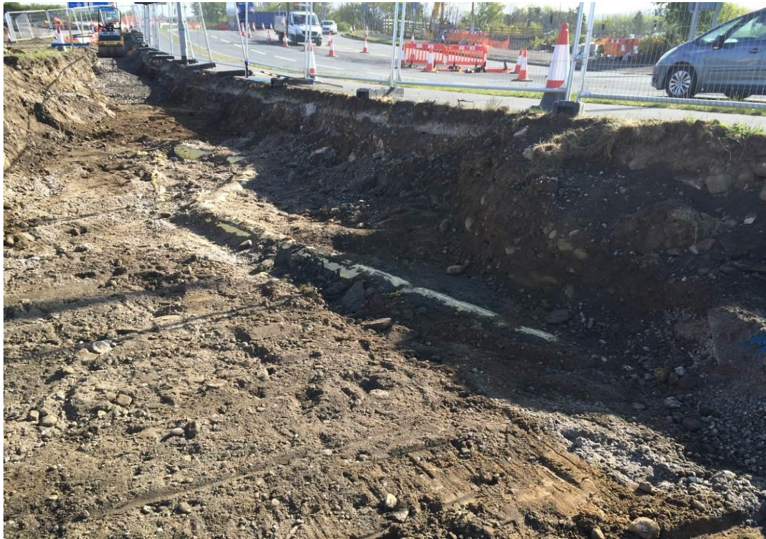
Photograph 5 – Looking northeast towards the motorway island.
