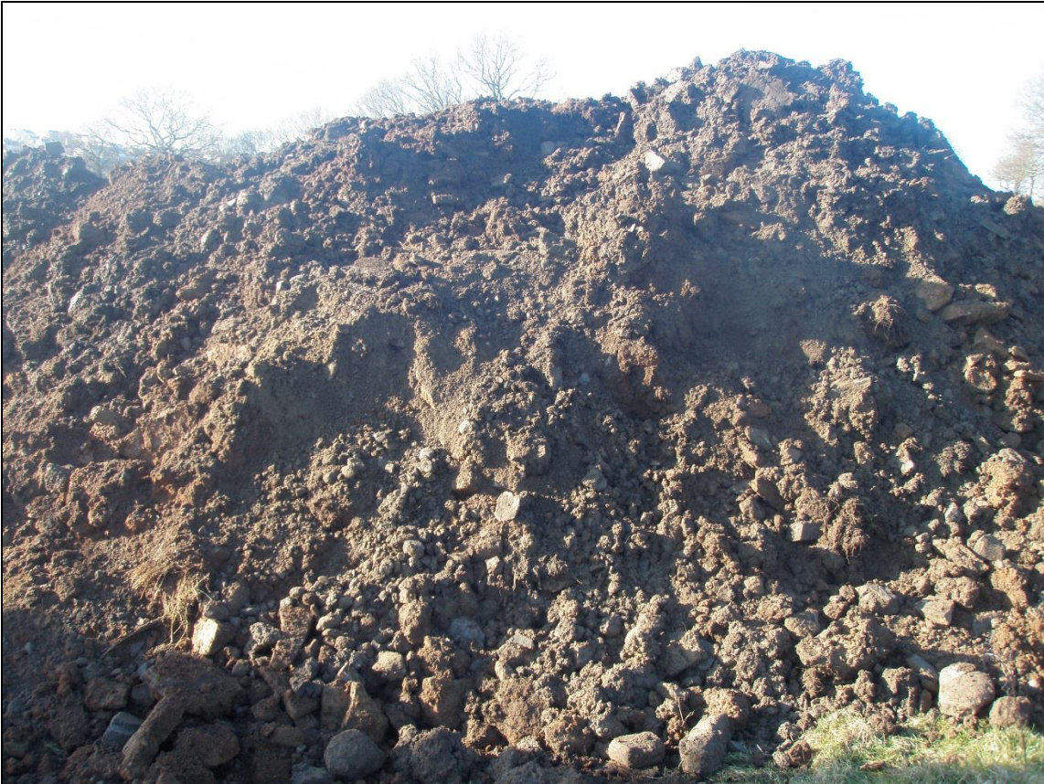
NSE31A Arisings from excavation. No visual or olfactory evidence of contamination
