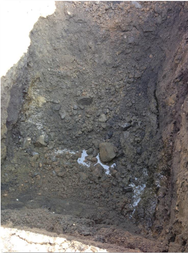
Photograph 7 NSW628- investigation into free product identified during ground investigation. No free product observed and no hydrocarbon sheen present on water seepage within excavation.
