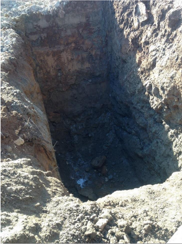
Photograph 5 NSW378 – excavation to remove recorded RBSL failure at 4.5m.
