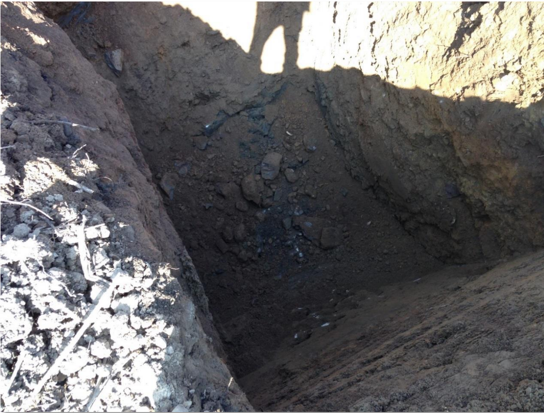
Photograph 3 NSW269 – investigation into oil ingress observed during ground investigation. No free product encountered,
