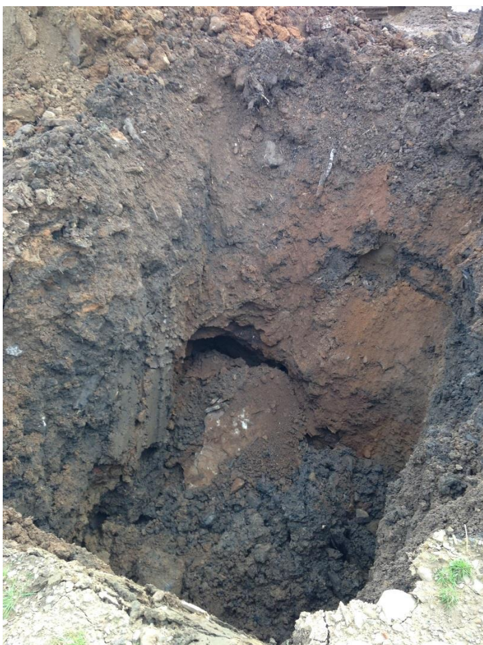
Photograph 2 NSW238 – investigation into observed oozing black liquid during ground investigation. Material assigned maximum VO score of 3,3, no oozing black liquid observed,
