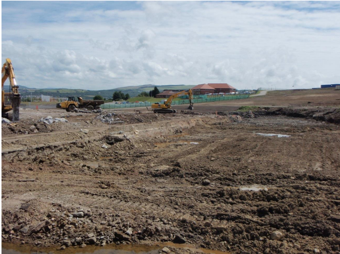
Photograph 15: Removal of existing roadway to the south of the former DIME Plant
