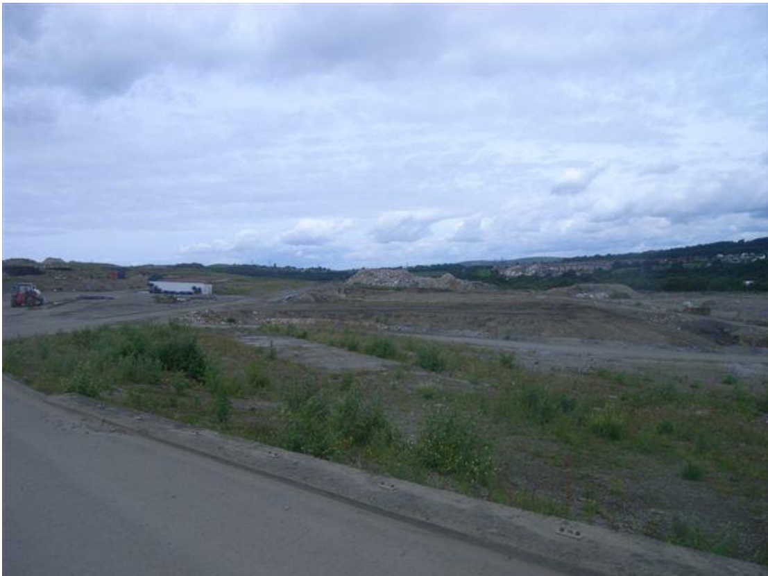
Photograph 8: Former central substation and bath house (June 2011)
