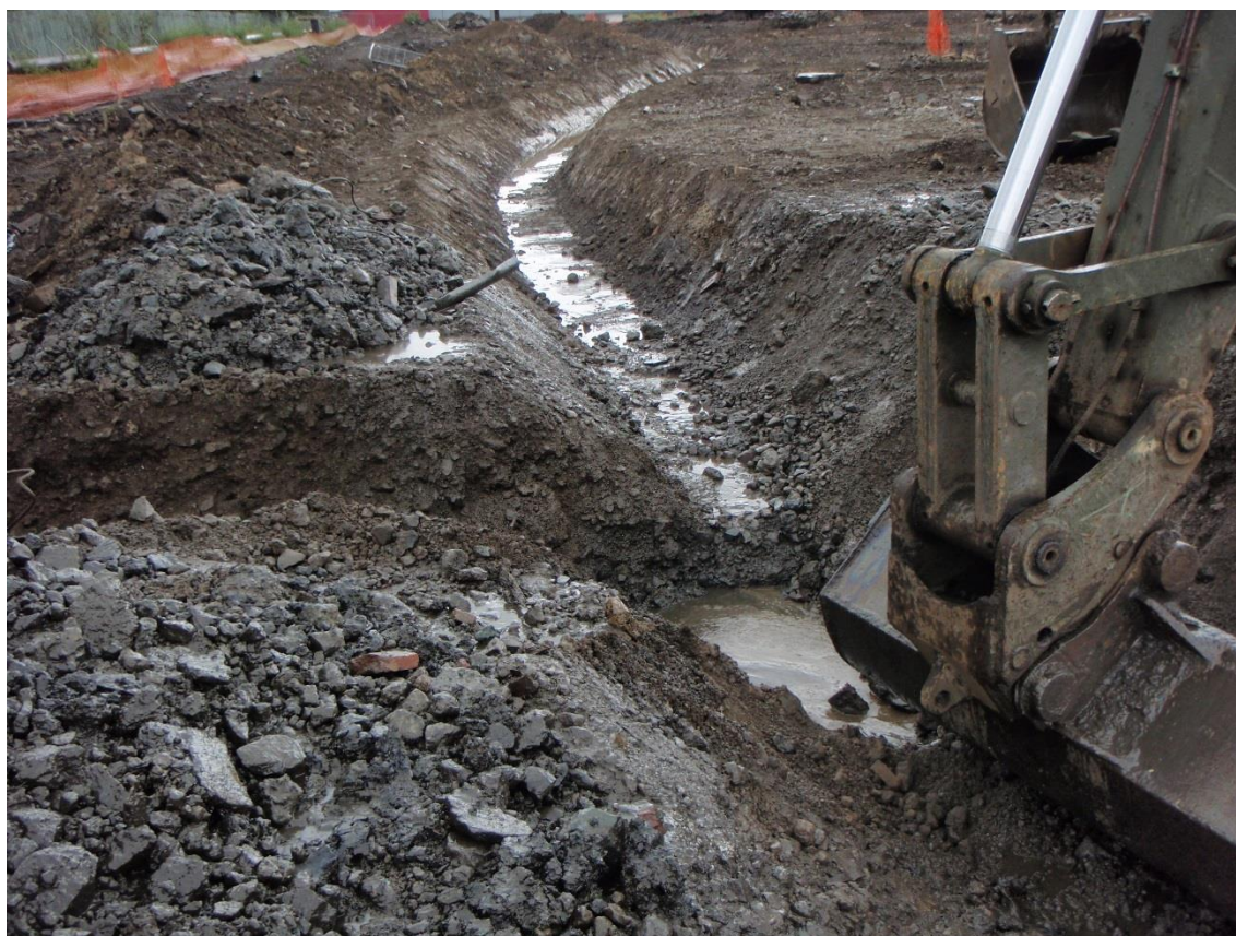
Photograph 11: Installation of new drainage ditch during hardstanding removal
