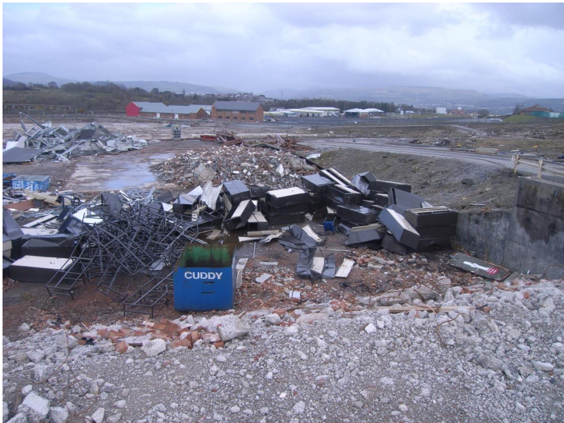
Photograph 6: New bath house demolition (March 2010)
