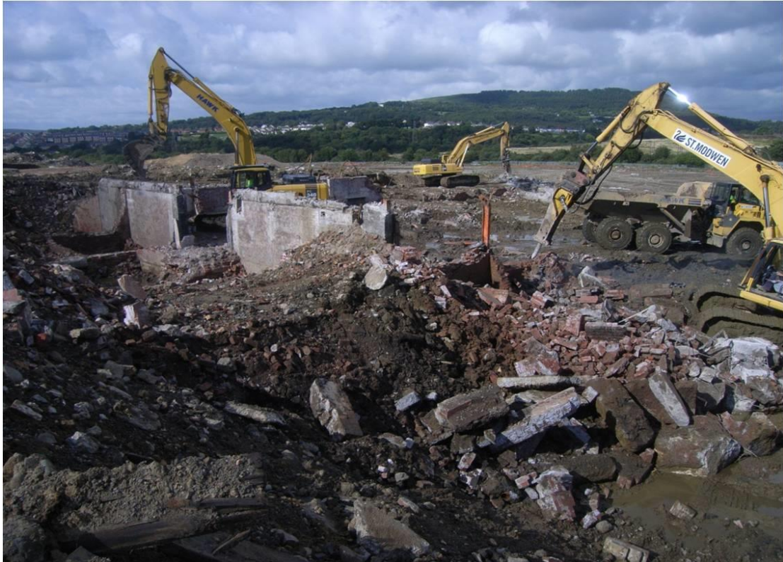
Photograph 7: New bath house and central substation foundation removal (August 2010)
