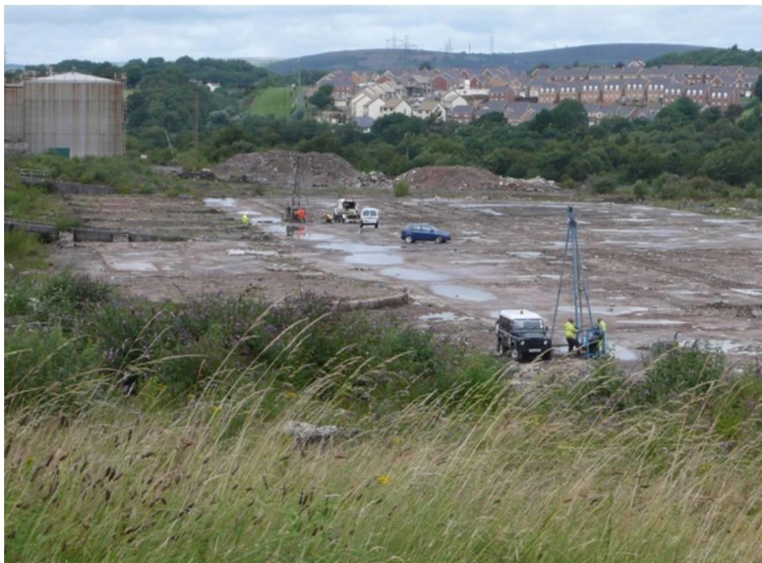
Photograph 2: Preliminary Ground investigations (July 2009)
