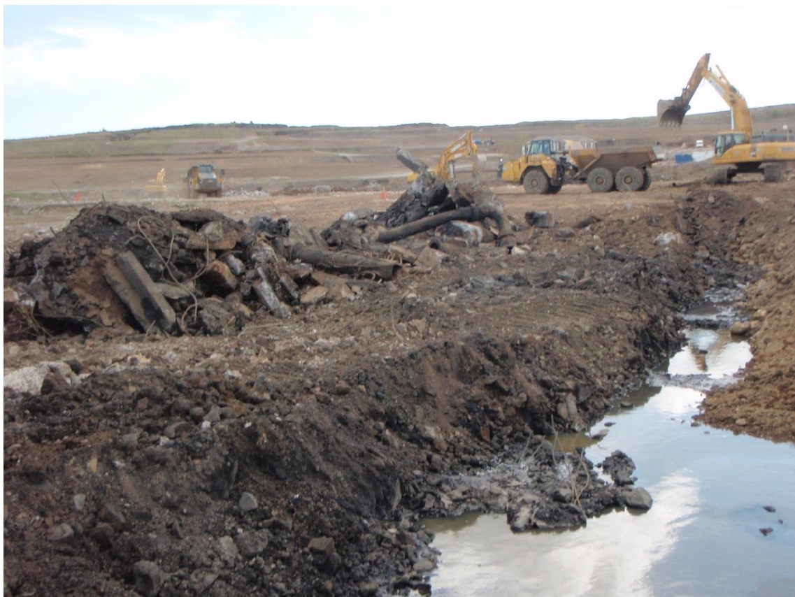
Photograph 14: Removal of identified pipework/relict infrastructure etc
