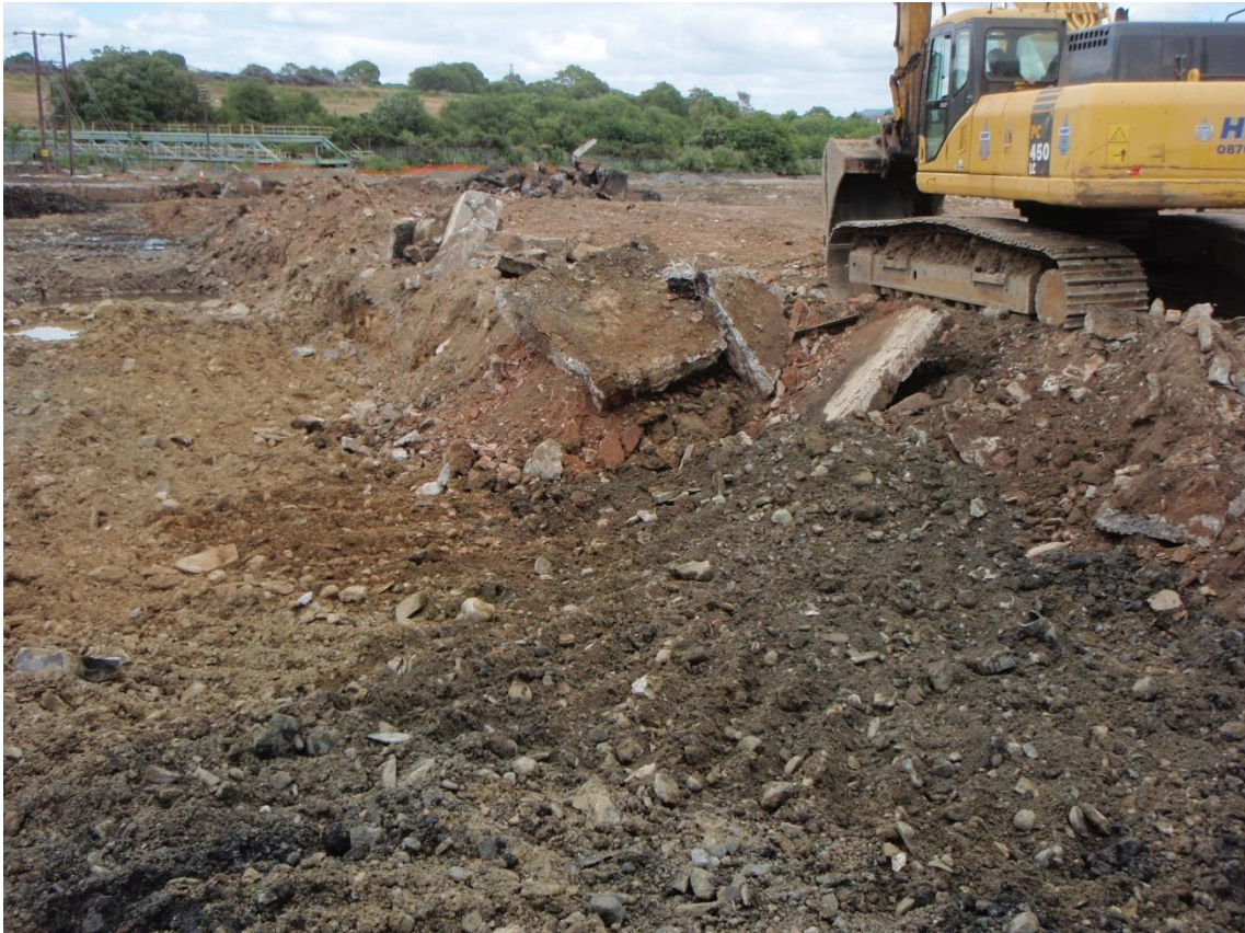
Photograph 13: Shallow (1m) turnover and structures removal
