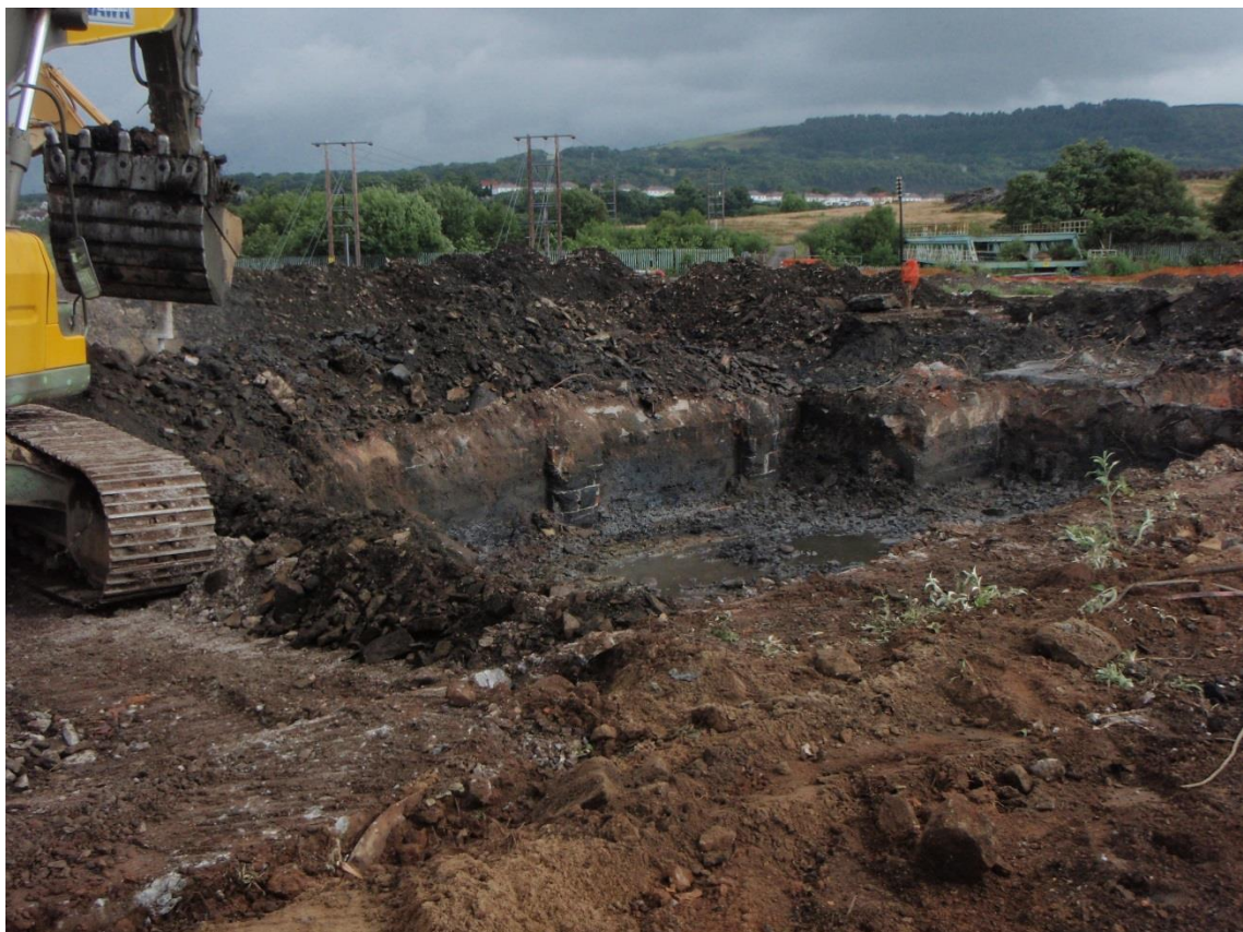
Photograph 16: Removal of existing below ground structures during the works
