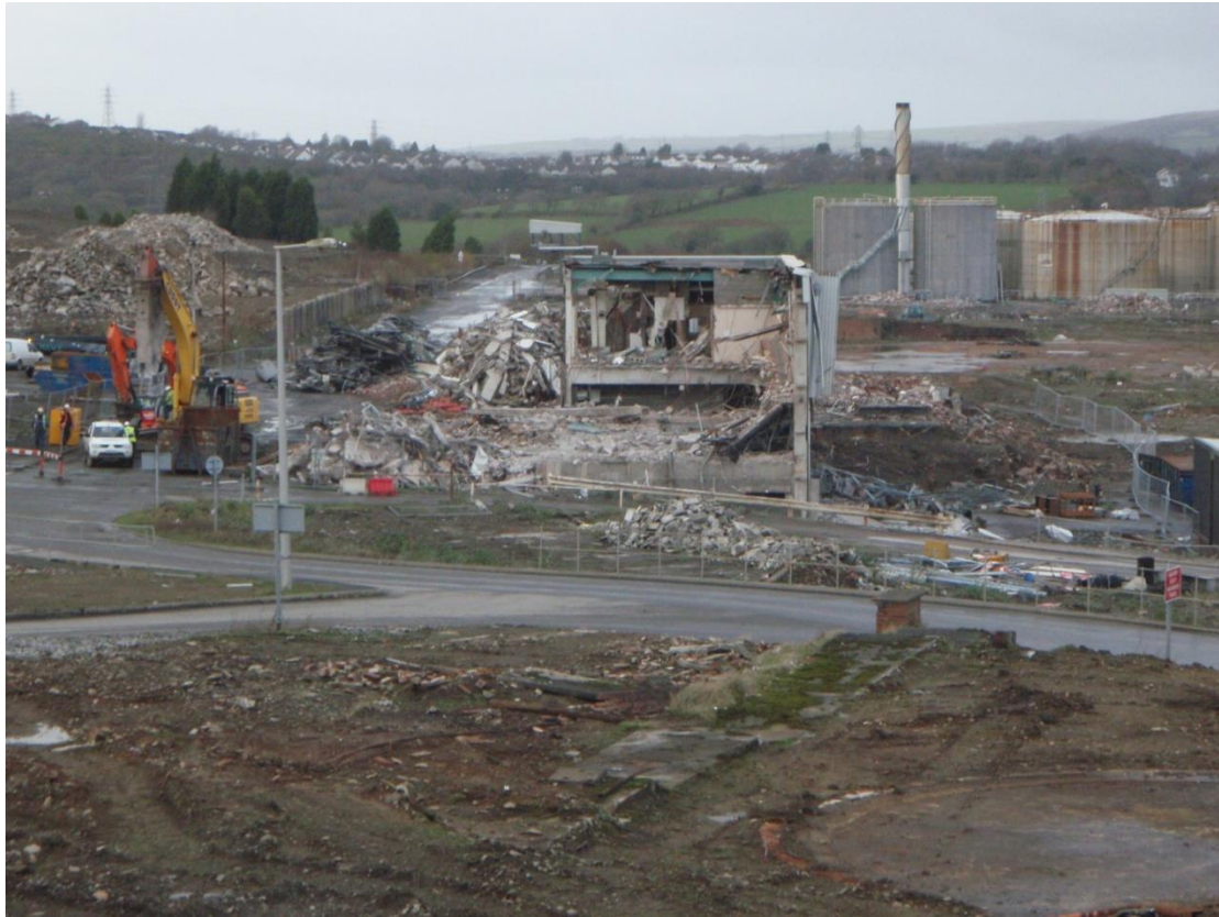
Photograph 5: Central substation demolition (December 2009)
