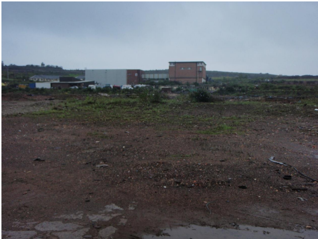
Photograph 4: Central substation and New bath house (2008)
