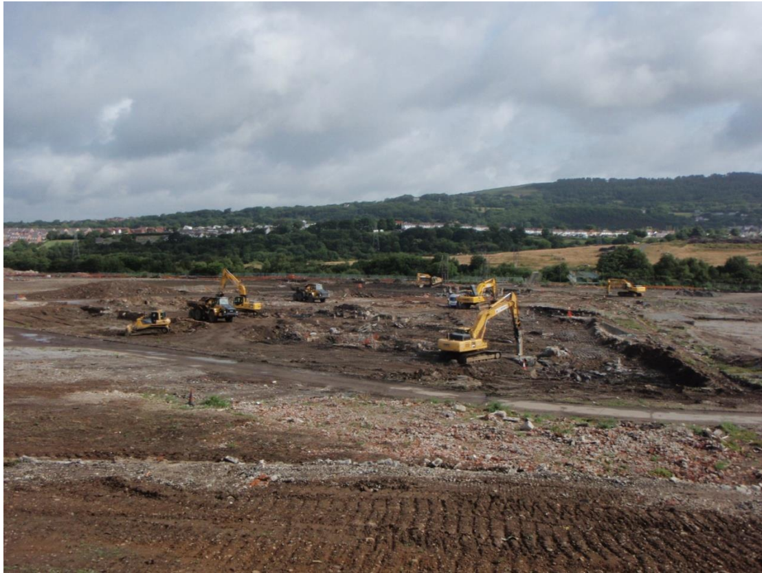
Photograph 3: DiME hardstanding removal July 2010
