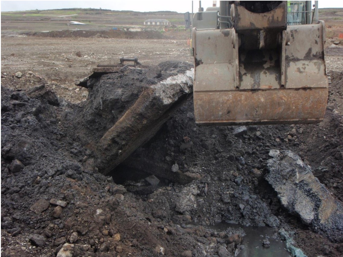
Photograph 9: Shallow turnover during hardstanding and drainage removal
