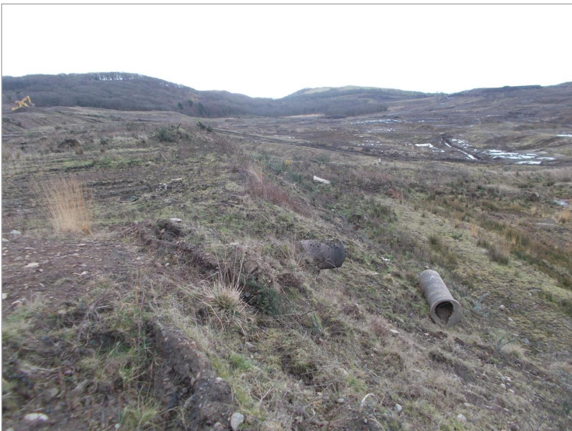
14) Drainage outfall pipe on southern tank farm
