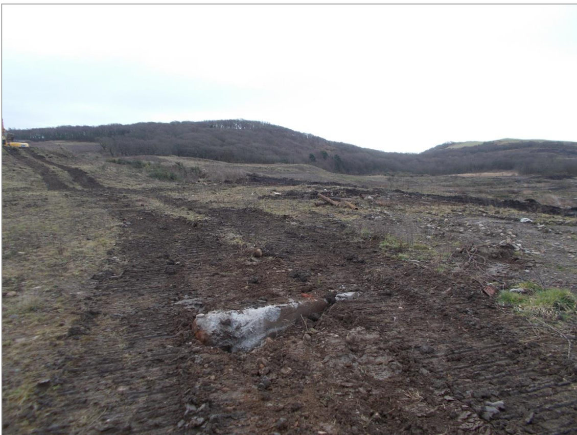
16) Residual concrete on southern tank farm
