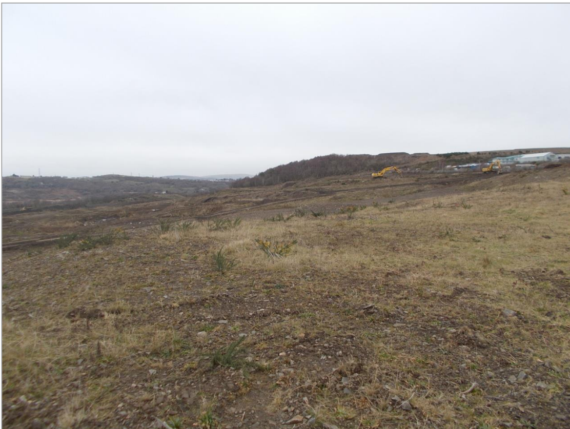
20) View north towards upper terrace
