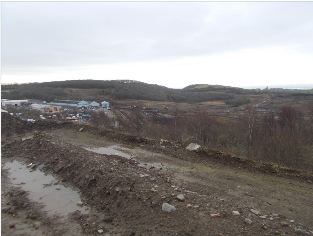
4) Looking south from upper terrace
