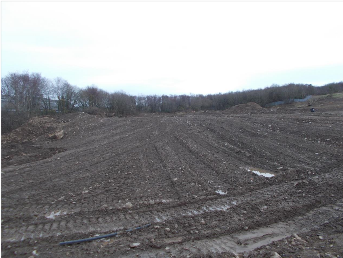
19) View east from main site road
