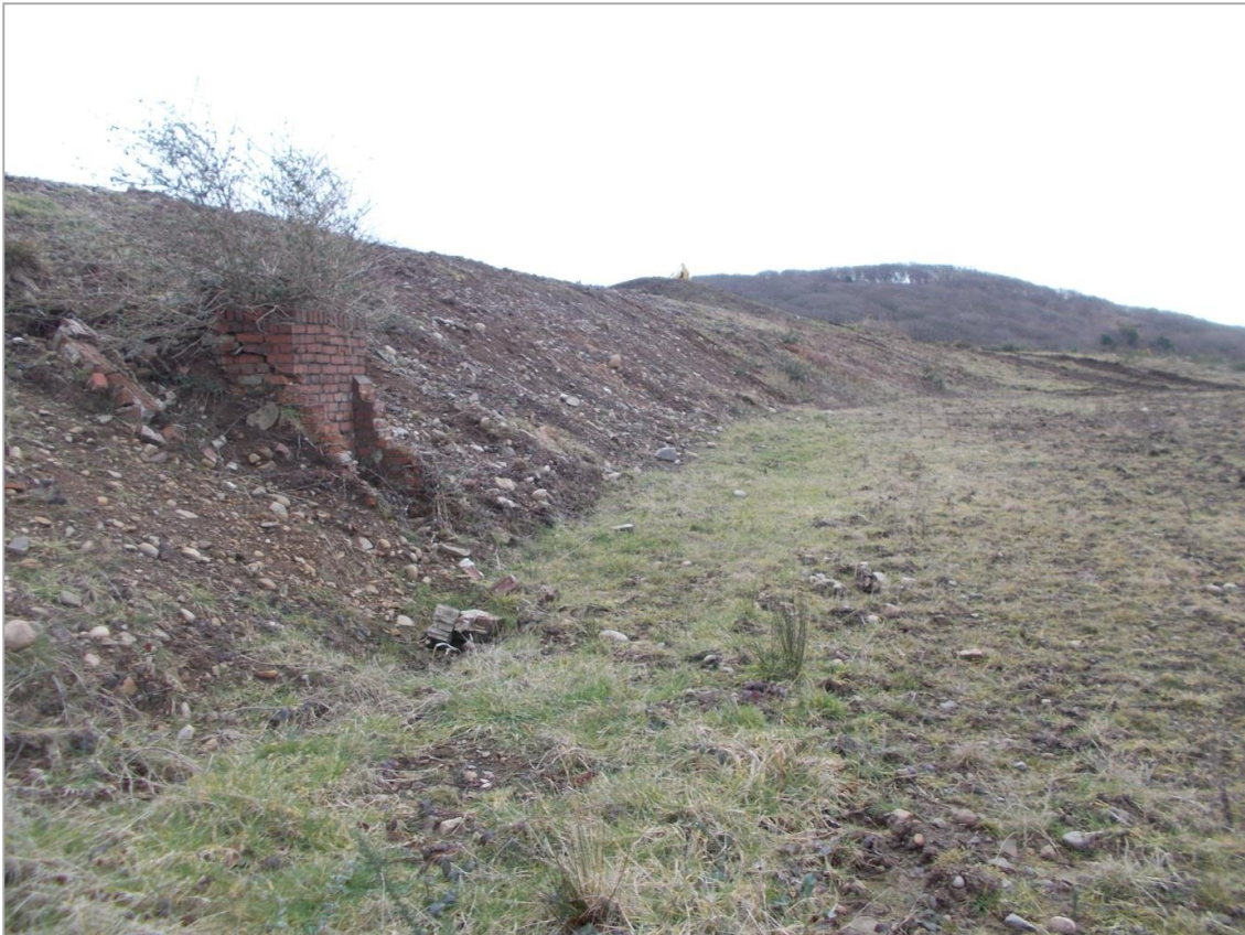
15) Brick structure on southern tank farm
