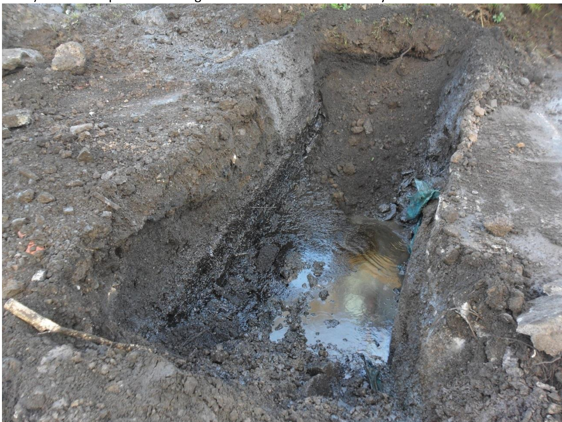
2) The southern edge of Zone D Separator.
