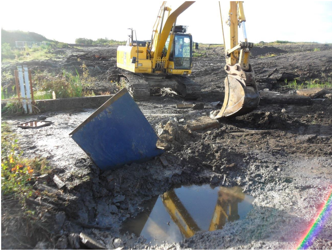
9) Backfill of the excavation around the separator following product removal
