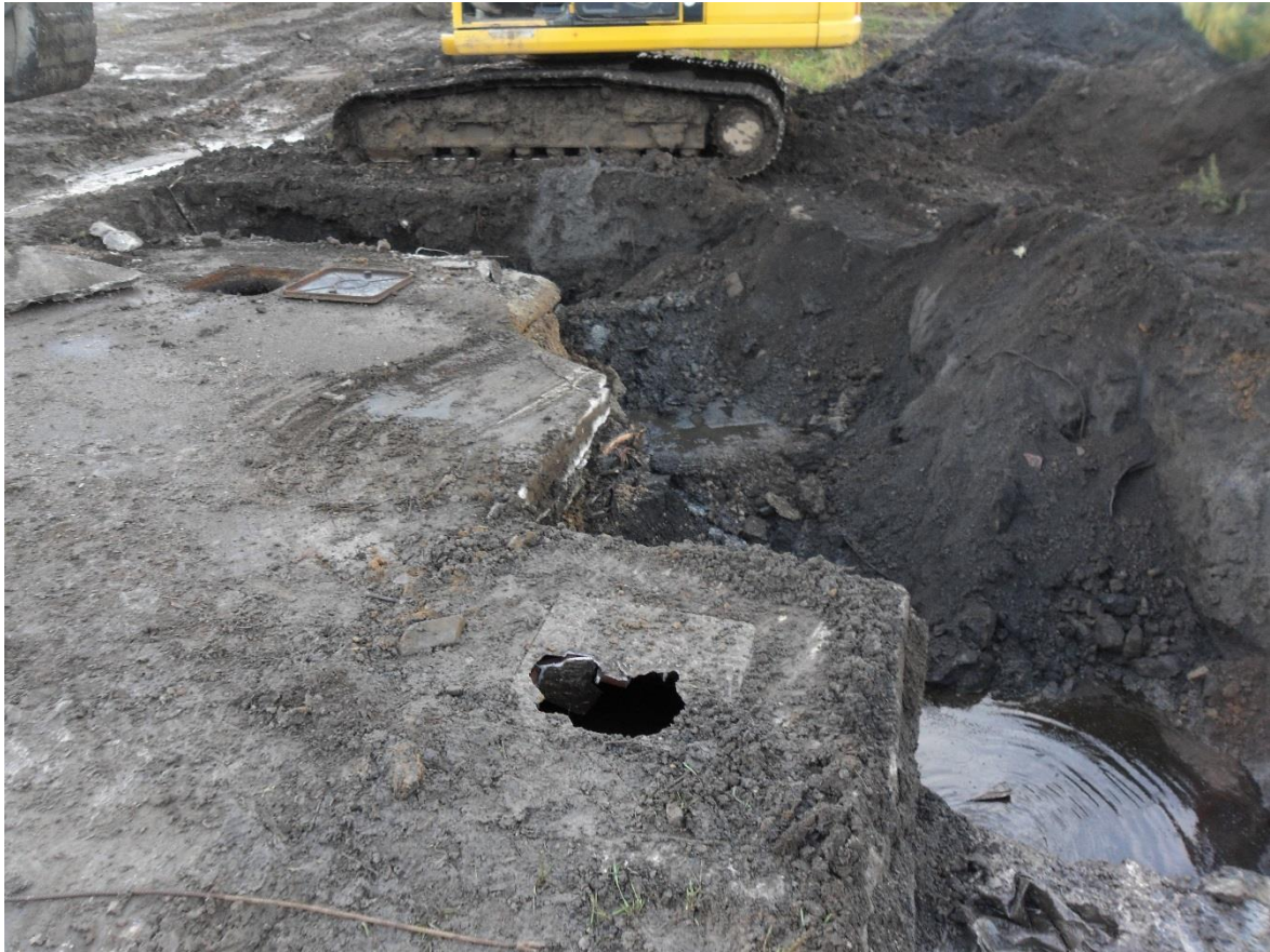
3) Exposing the side of the separator
