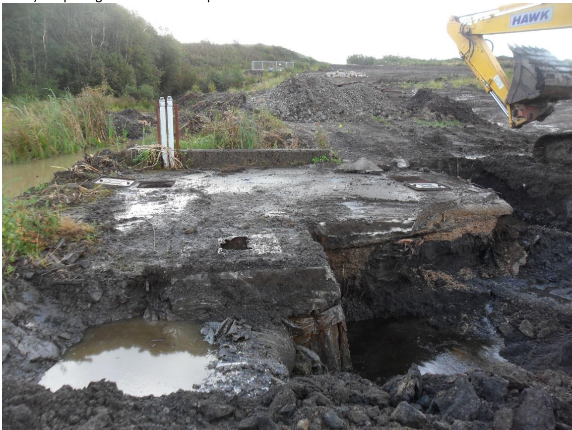
4) Exposing the side of the separator
