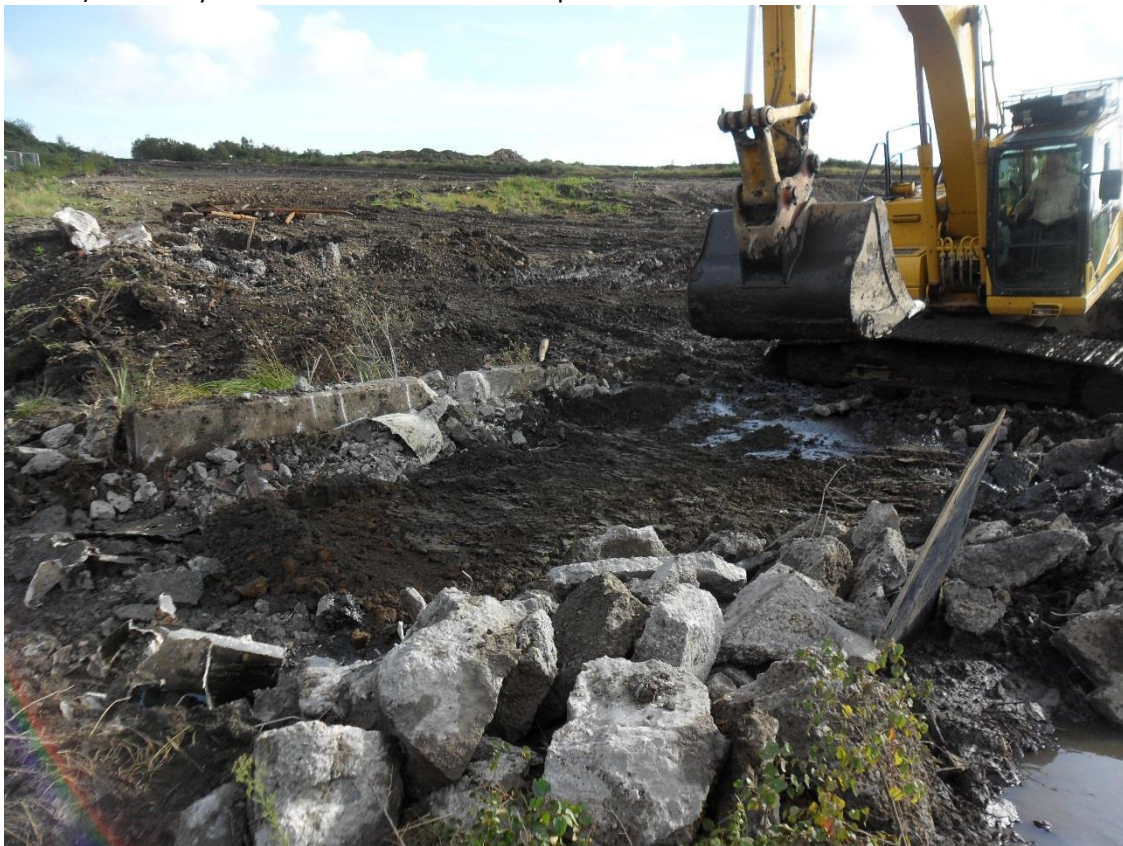
14) Backfilling of the separator following the removal of material and oily water.
