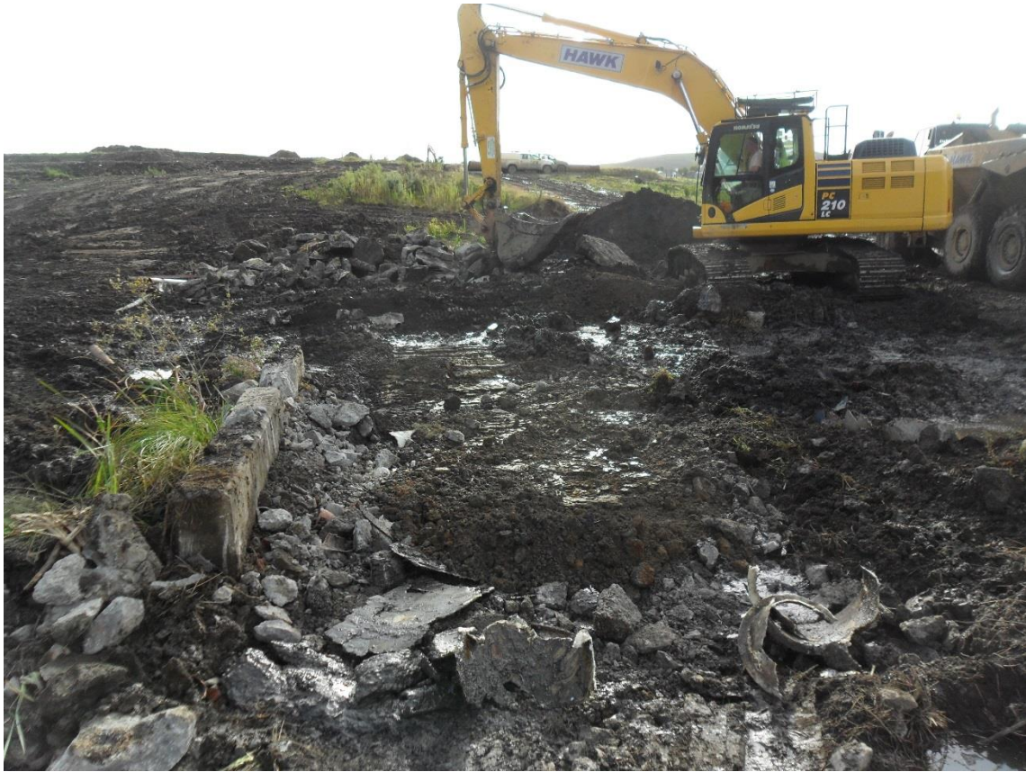
15) Backfilling of the separator following the removal of material and oily water.
