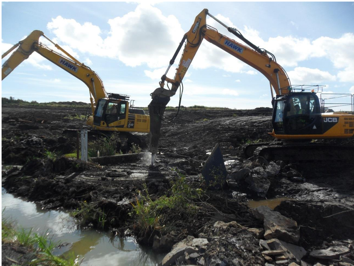
10) Commencement of breaking the top off the separator.
