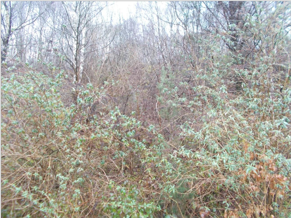
23) Pipe work supports upslope of service road (blocked by trees)
