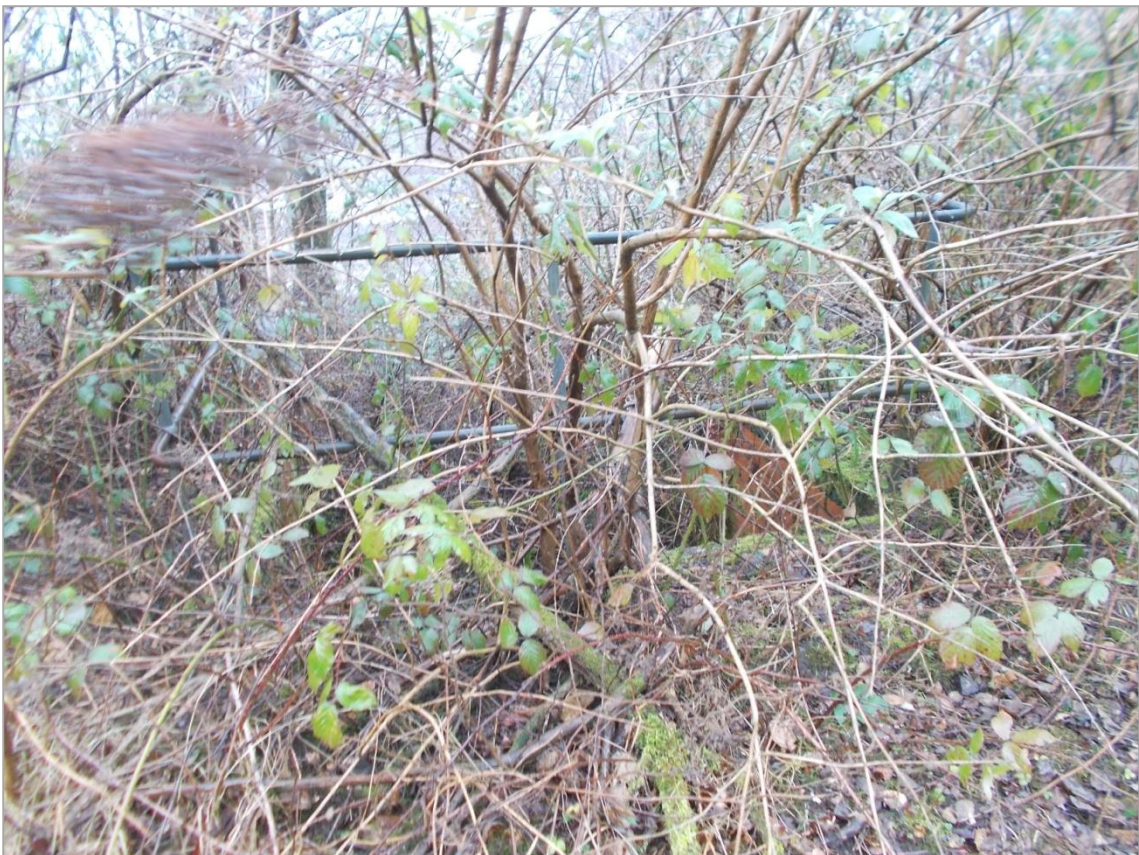
22) Pipe outfall located on service road
