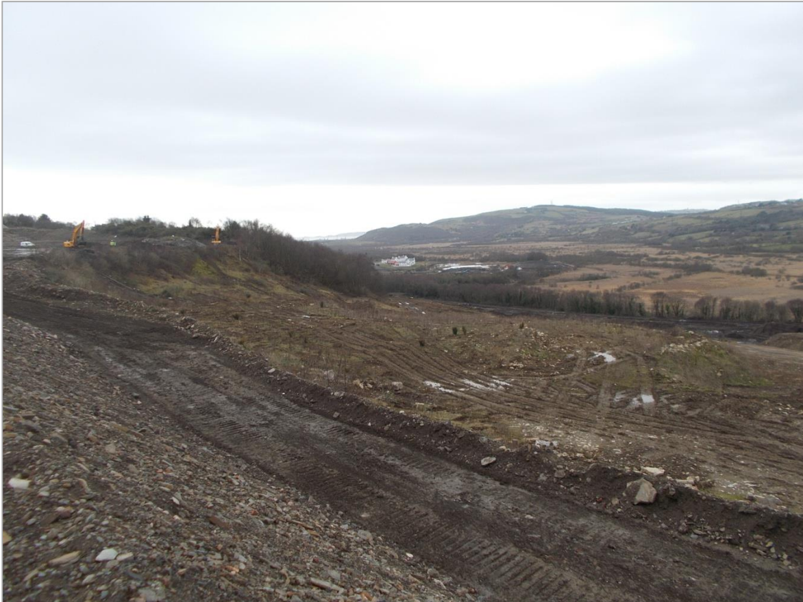
16) Looking south across stockpile area
