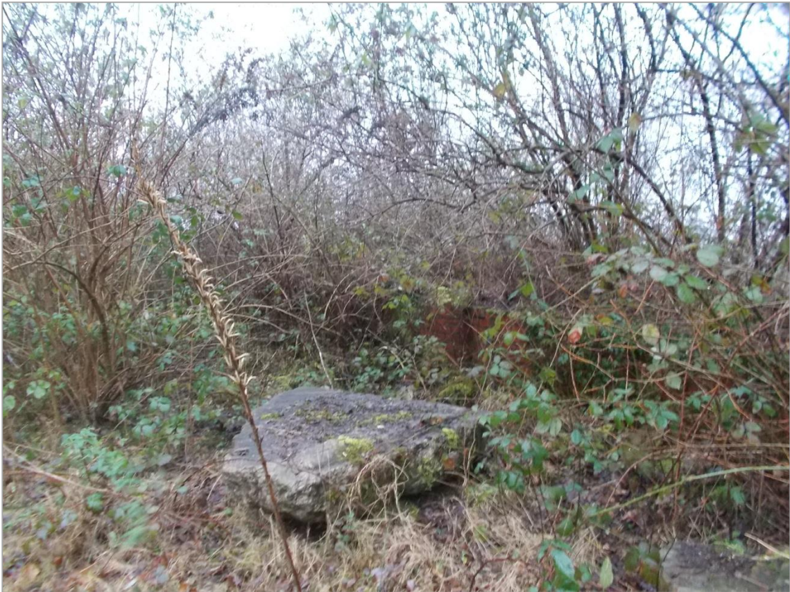
21) Brick structure located on the service road
