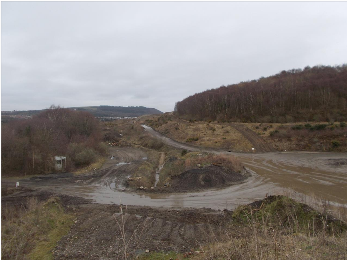
9) Taken from stockpile looking north along main site road
