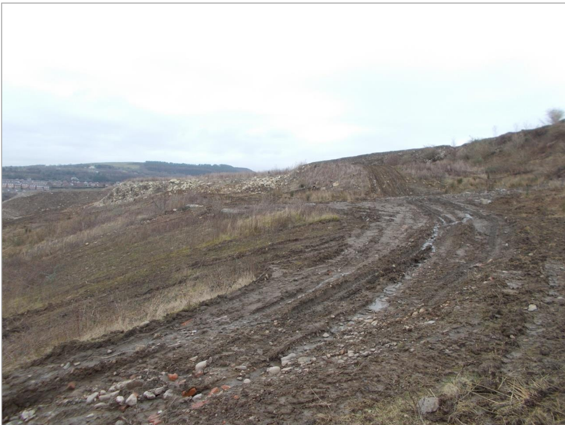
14) Looking north across former import stockpile area
