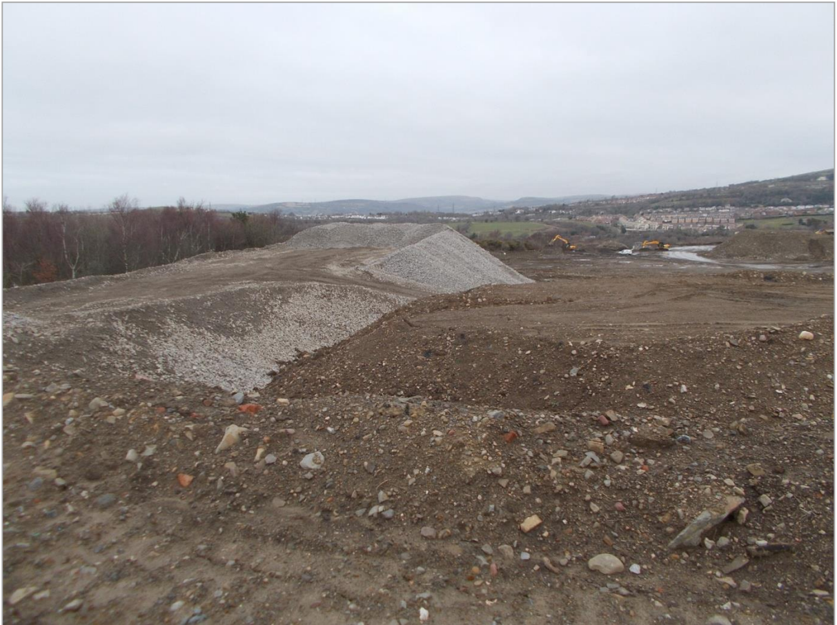
29) View across upper terrace
