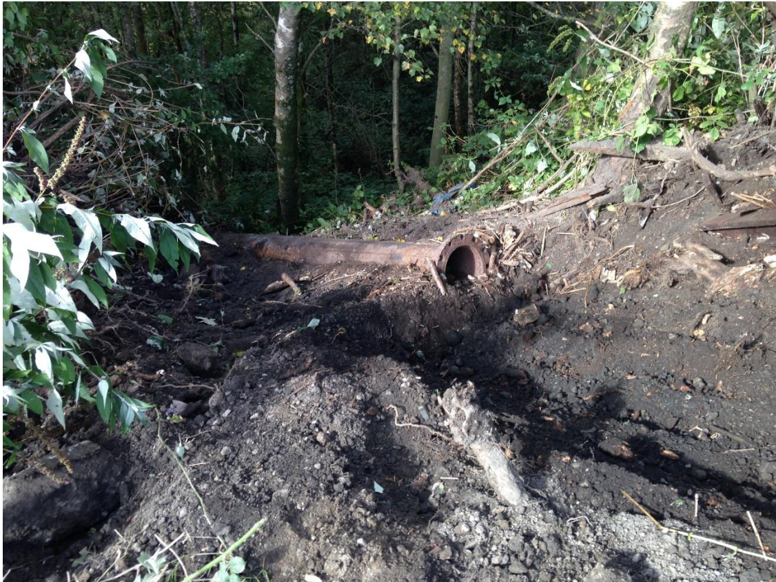
1) Pipe 1 – northern most pipe exposed and removed. Viewing north west
