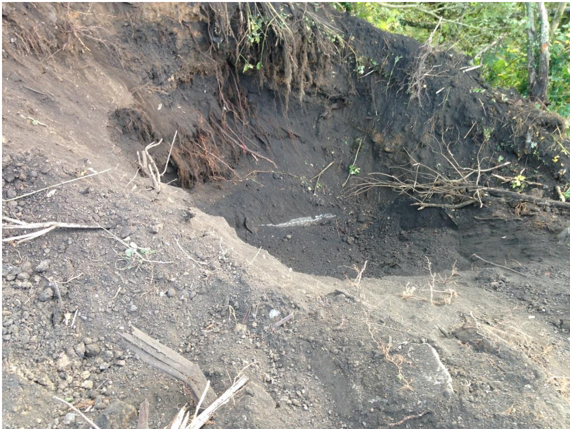
4) Pipe 2 - Southern most pipe exposed and removed. Viewing south west
