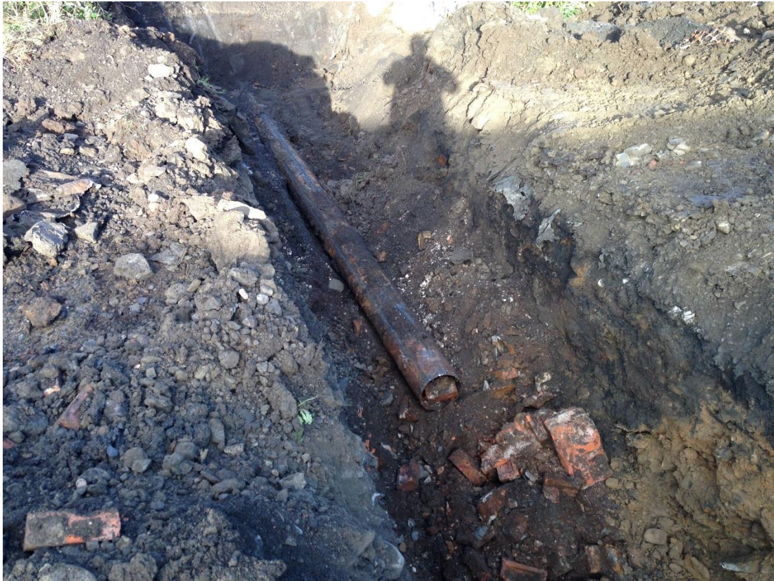
5) Pipe 2 – length of pipe located under the haul road removed
