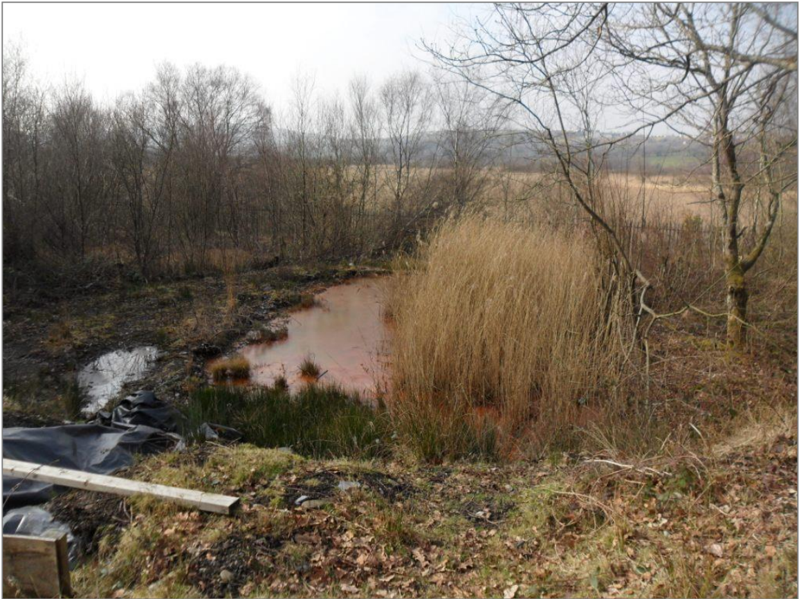
Photograph 15: Reedbed fed by the discharge of the interception trench. Note the ochreous water.
