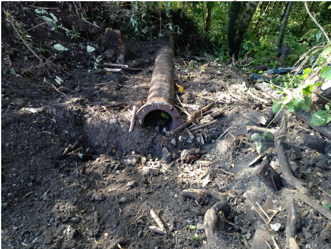
2) Pipe 1 - northern most pipe exposed and removed
