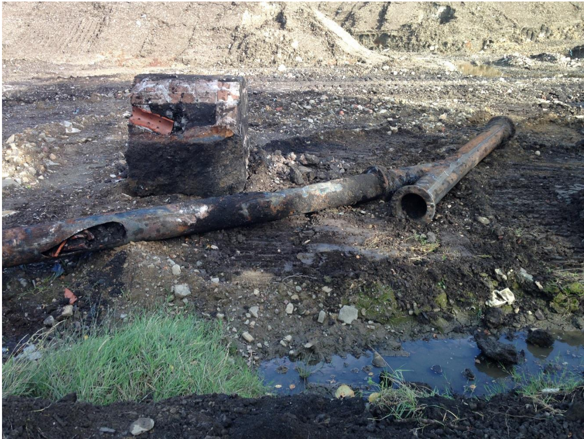
9) Pipe 3 – Sections removed.
