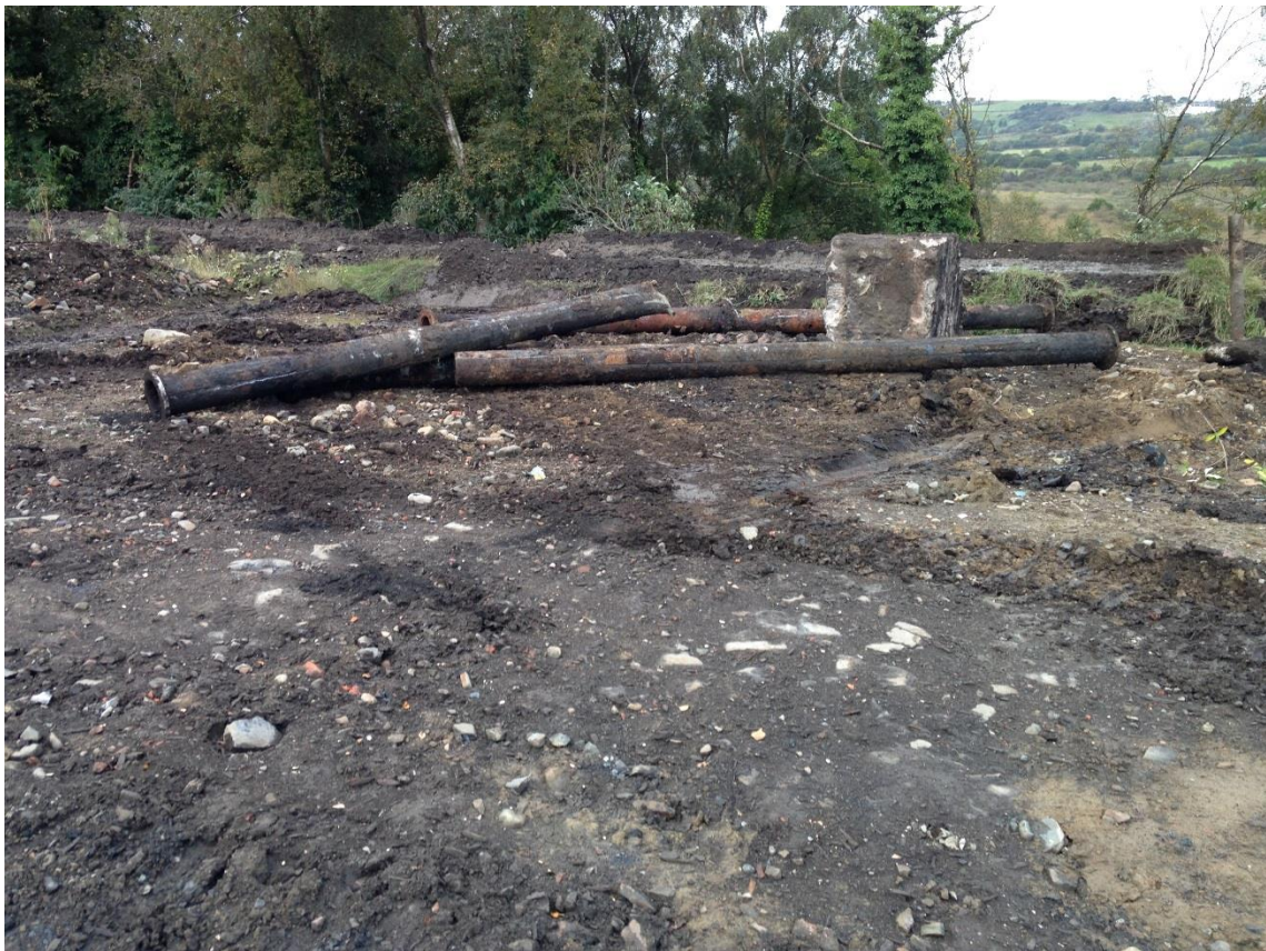
6) Pipe 2 sections removed
