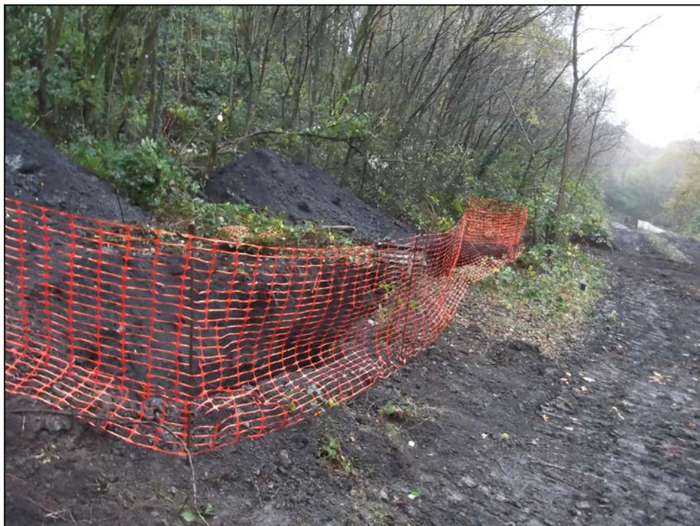
Photograph 6 – Complete excavation to east and west of Sump 5
