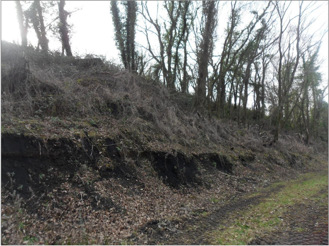
Photograph 31: Track cutting viewing to the south towards the containment area.
