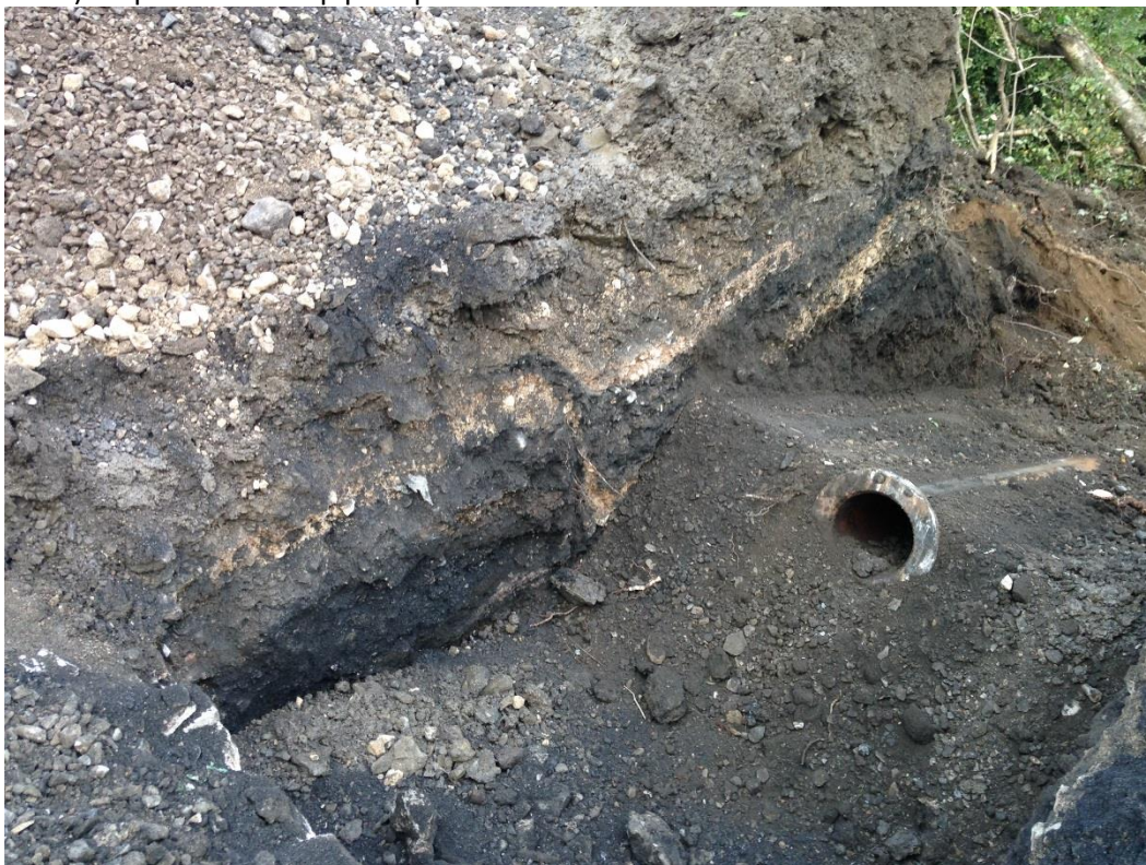
8) Pipe 3 - Middle pipe exposed and removed
