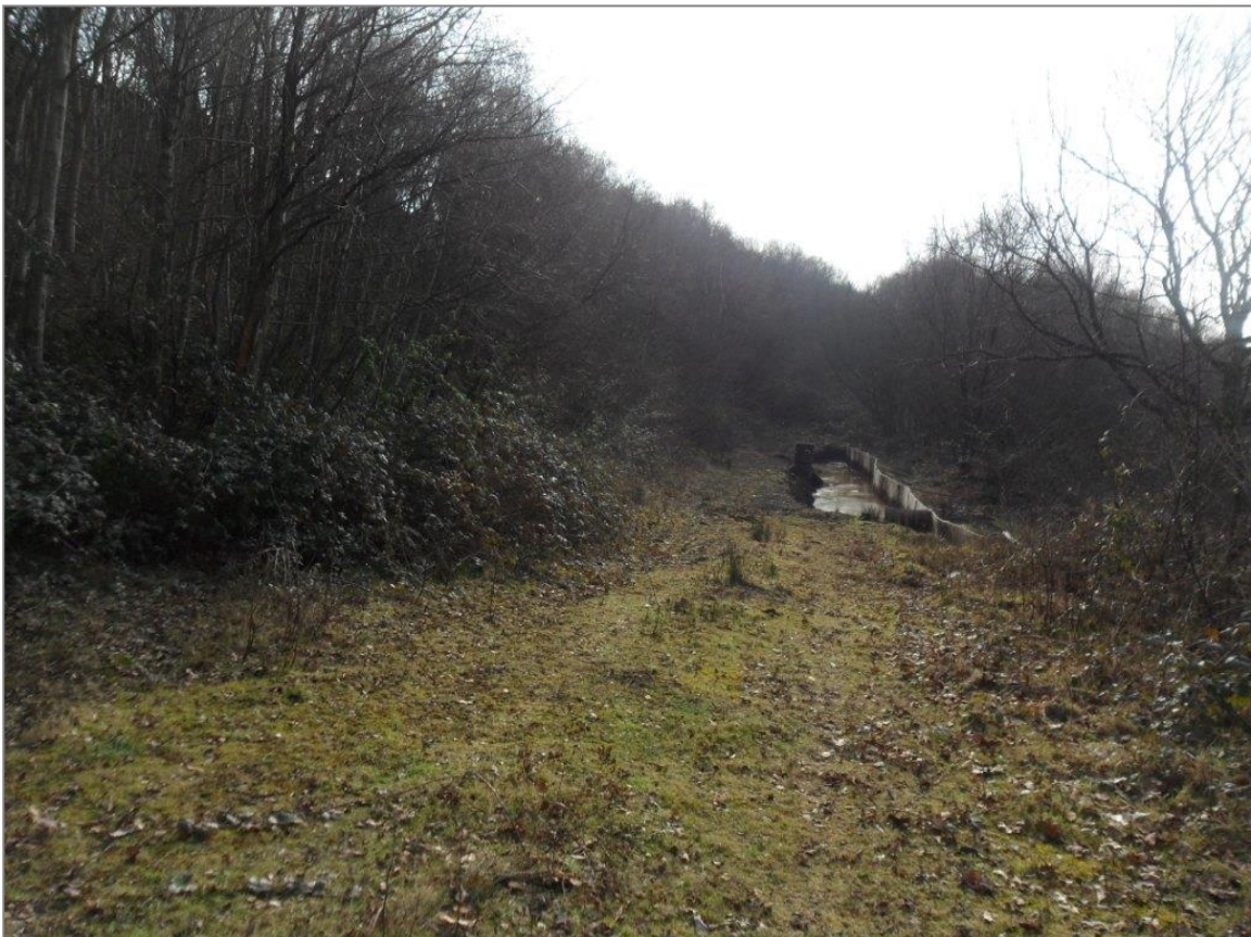
Photograph 14: Grassed track with dense woodland both sides and the interception trench in the background.
