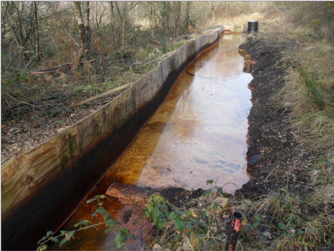
Photograph 17: The western margin interception trench with oil sheen and some free product. Note the 200mm diameter pipe entering the trench.
