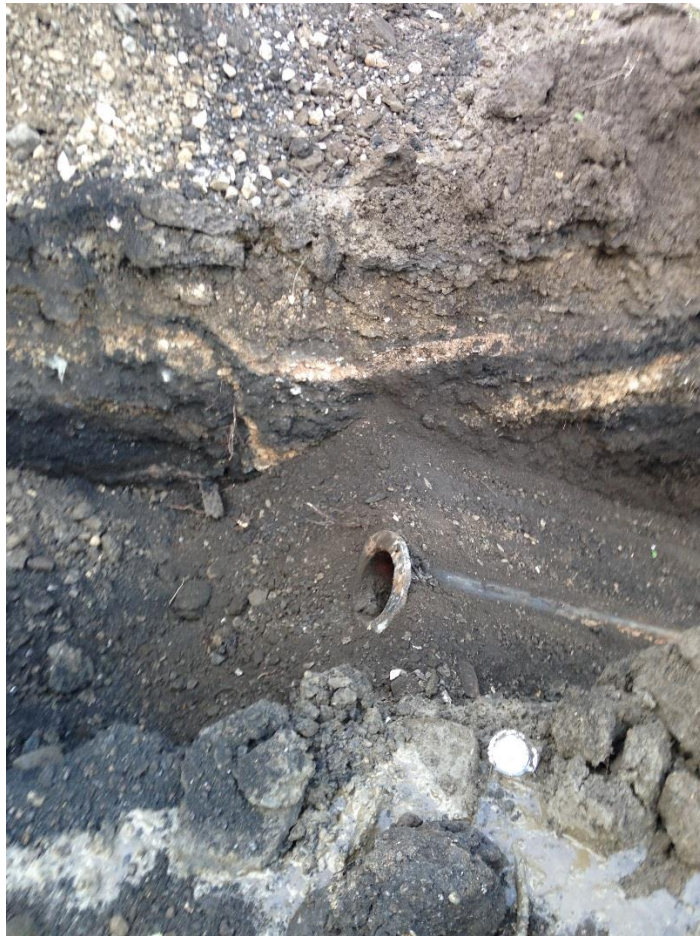
7) Pipe 3 – Middle pipe exposed and removed
