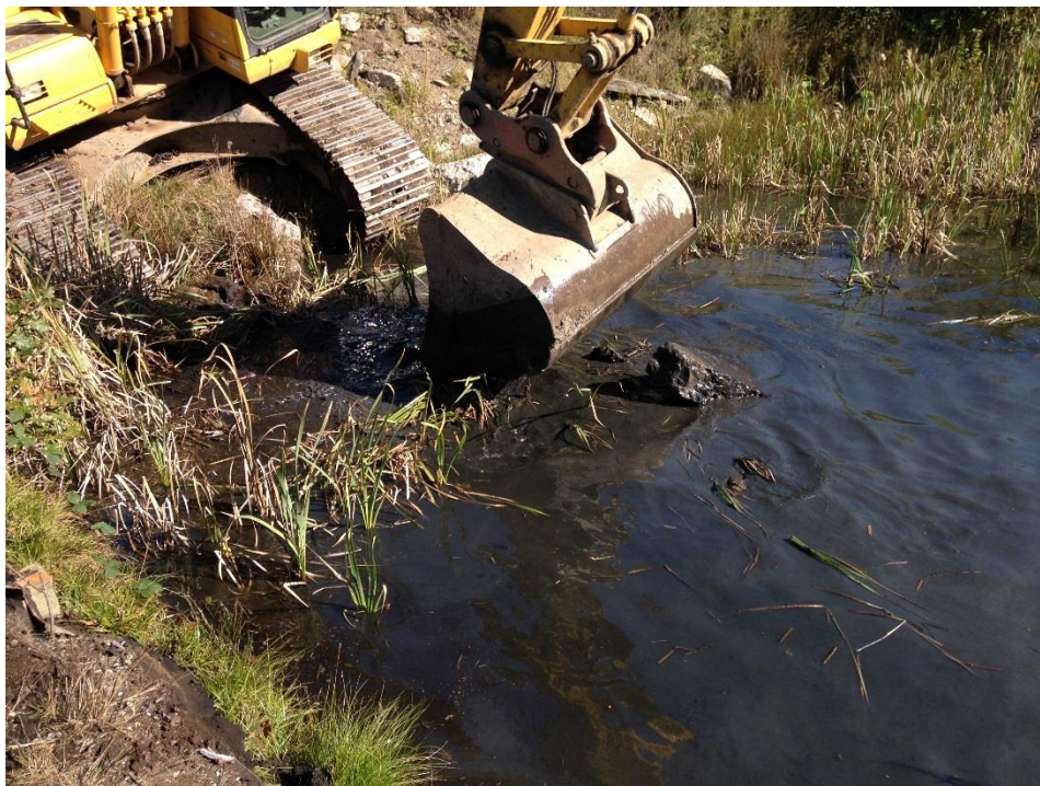
Photo 6 – Excavations stirring waters edge – note lack of release oil or iridescence
