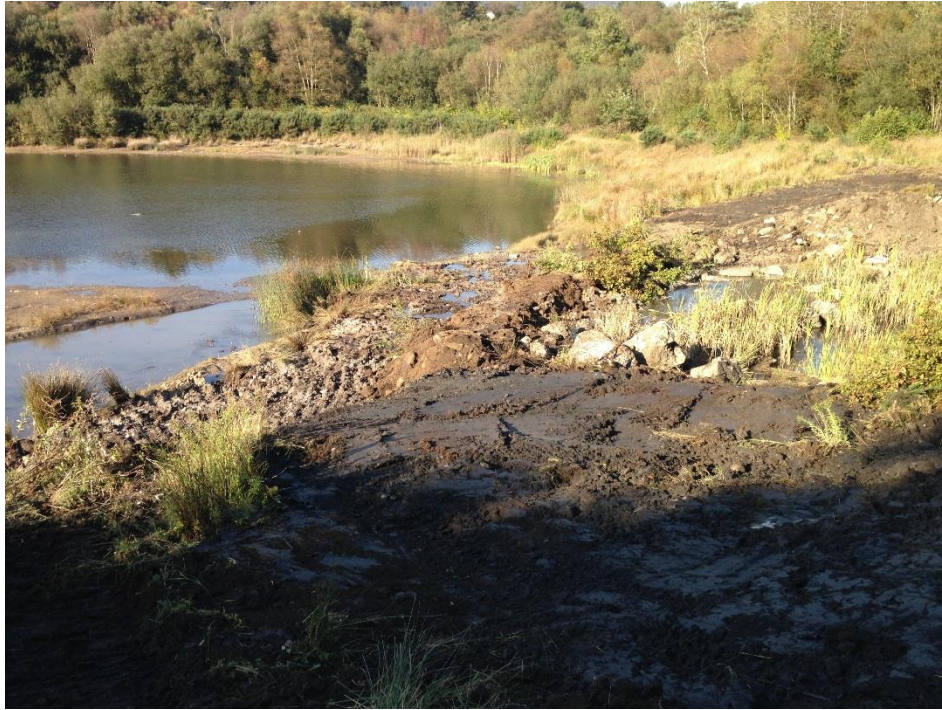
Photo 10 – Works area on completion
