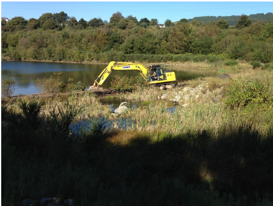
Photo 5 – Excavator positioned and excavating in front of former interceptor wall
