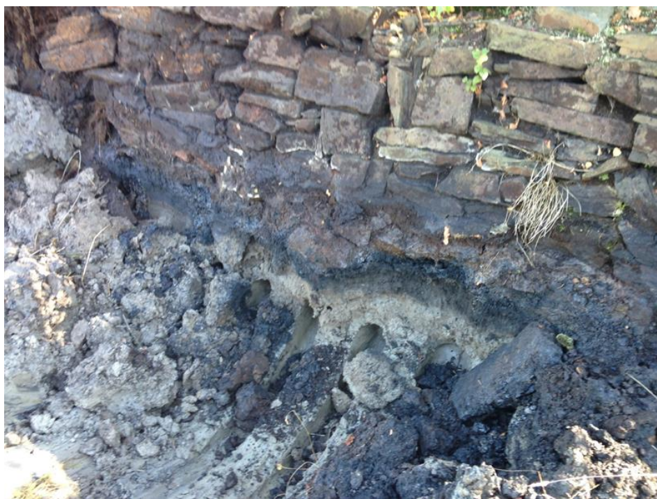
Photo 7 – Excavation adjacent the former interceptor wall, note clean underlying clay and residual oil/water seepage from the base of the interceptor wall (removed during the works)
