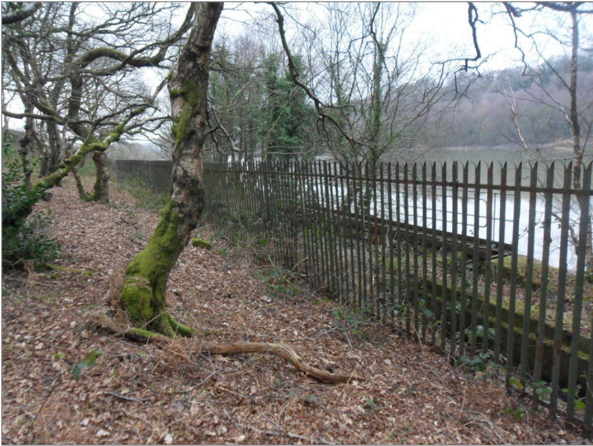
Photograph 11: Palisade fencing restricting access to the NSR.
