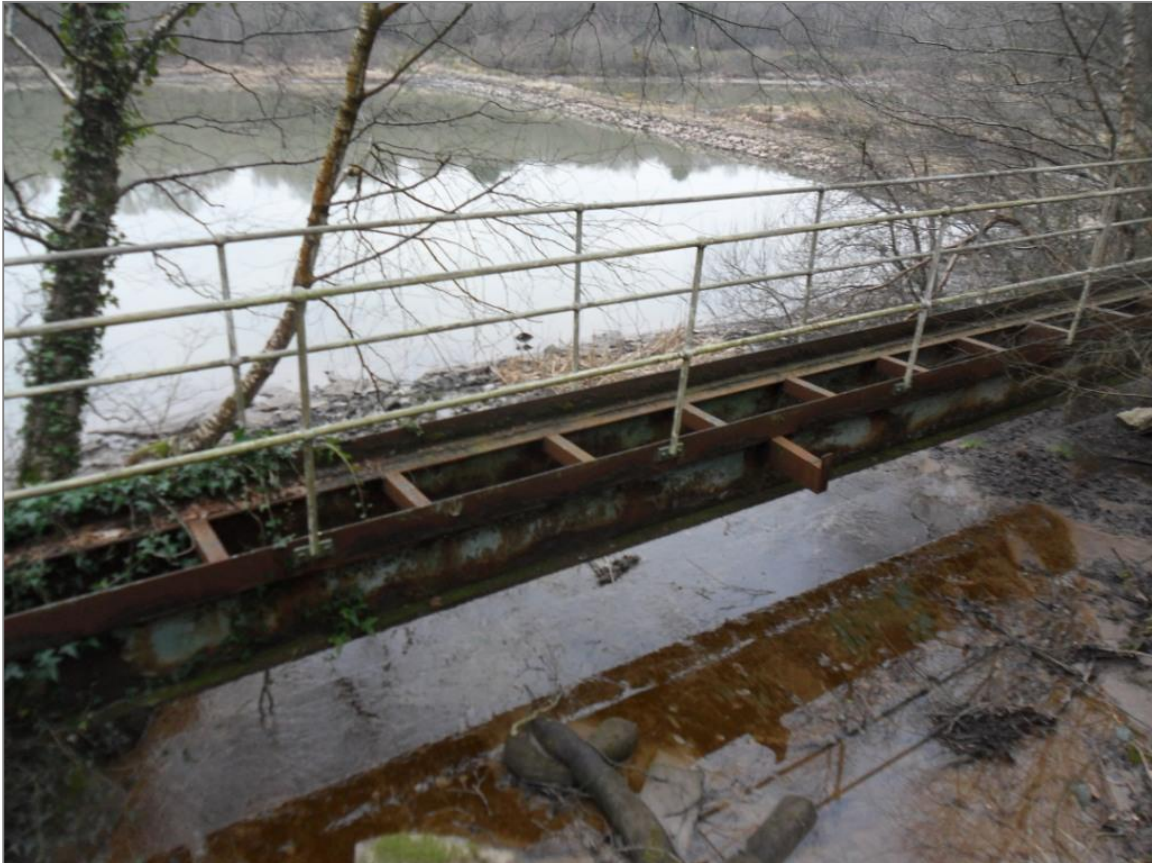
Photograph 12: Former metal foot bridge spanning a spillway where the water originates from the NSR API separators.
