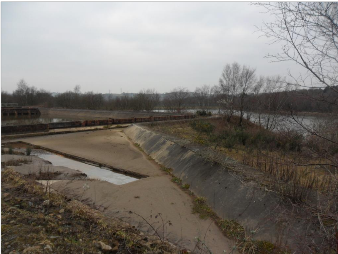
Photograph 24: Concrete channel looking towards the NSR API separators.
