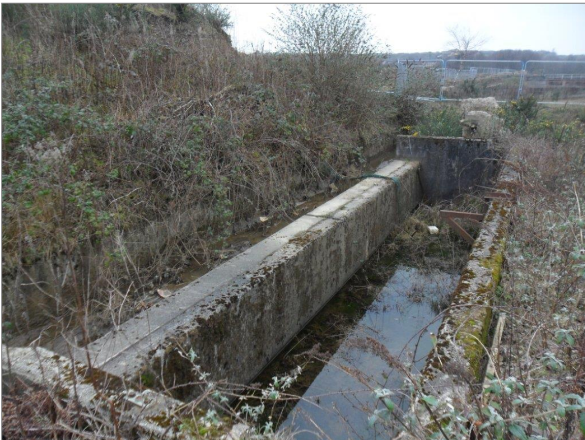
Photograph 22: Concrete structure adjacent to drainage channel.
