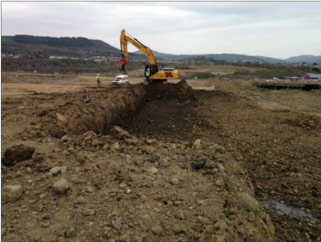
30) Overburden removal on the north west of the site showing indicative pre and post reclamation depth in this area in the south of the site.
