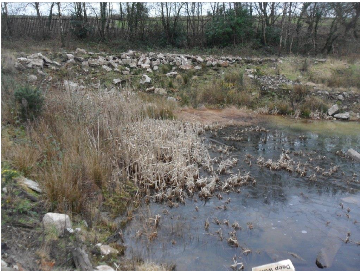
Photograph 8: Open excavation currently flooded in the area of the former east bay oil water separators. Remnant concrete boulders along the edges from the demolition of the former structure.
