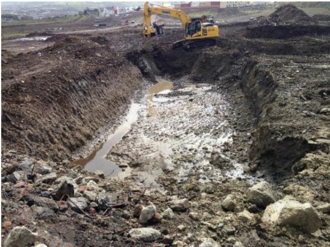
27 ) Commencement of the removal of overburden prior to excavation of material failing visual and olfactory criteria in SW of the site.
