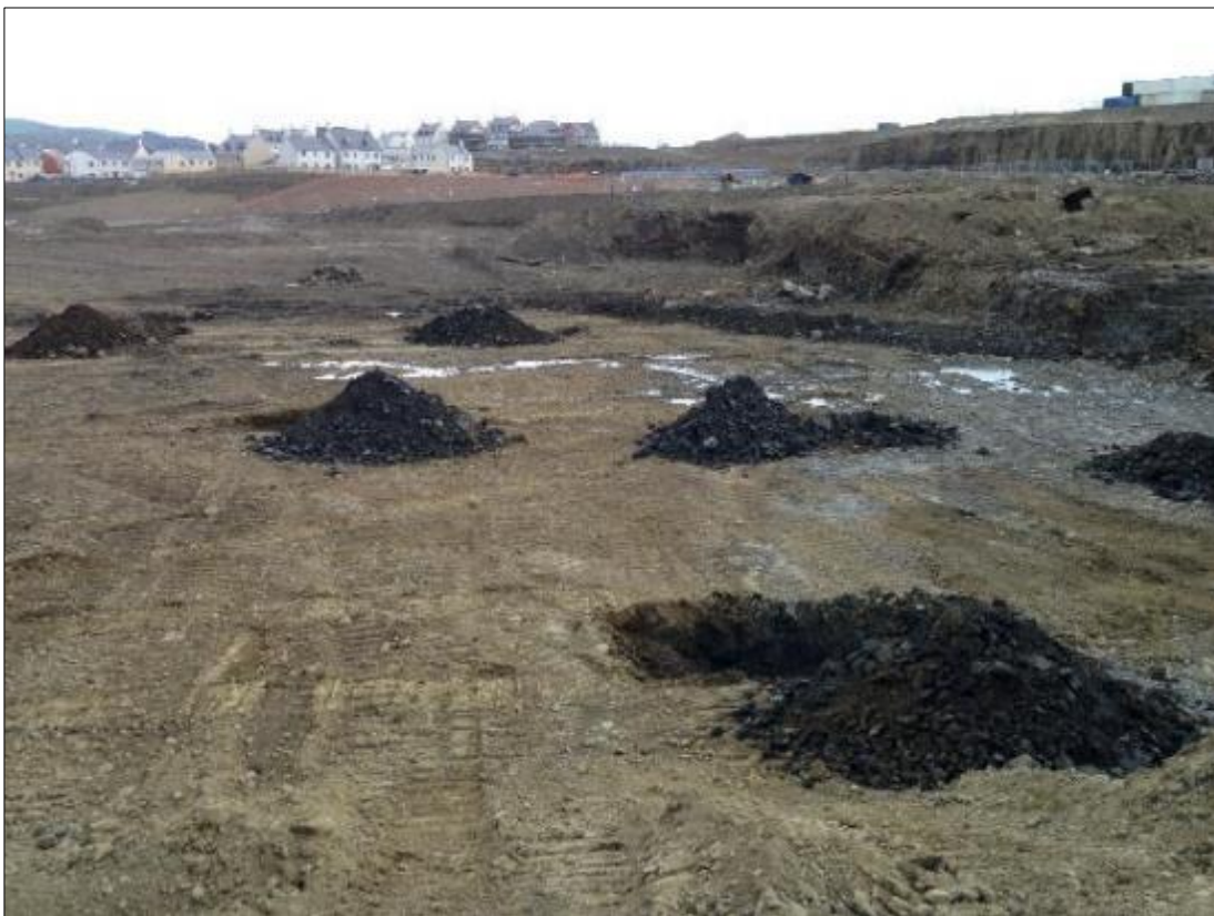
31 ) Visual and olfactory validation pits across the southern pitch area
