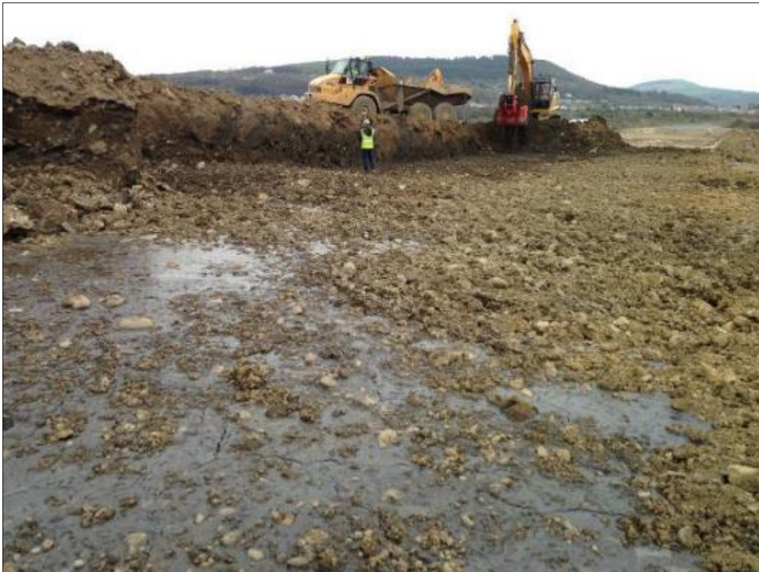
28) Exposure of highly odorous and viscous 'tarry' material prior to removal
