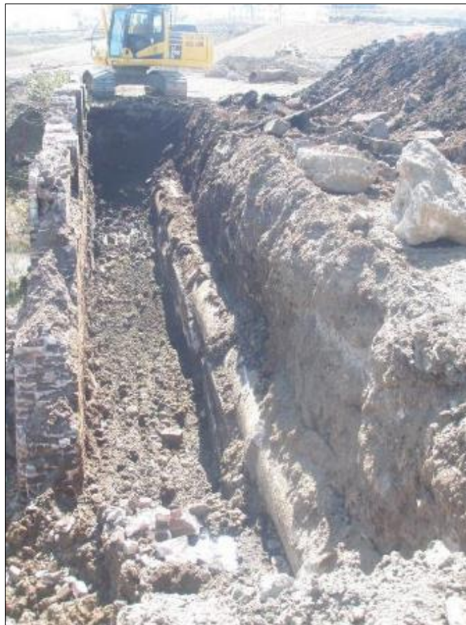
19) Exposure of 400mm concrete pipe section behind brick retaining wall prior to removal – see also photo (18)
