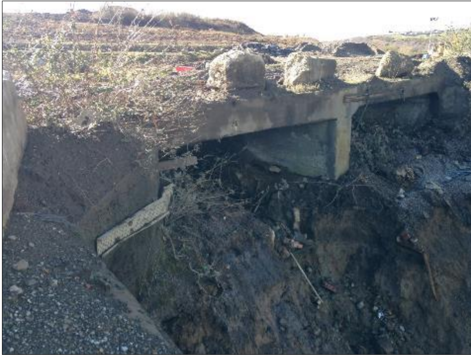
22) Road bridge prior to removal with former pipe track underneath
