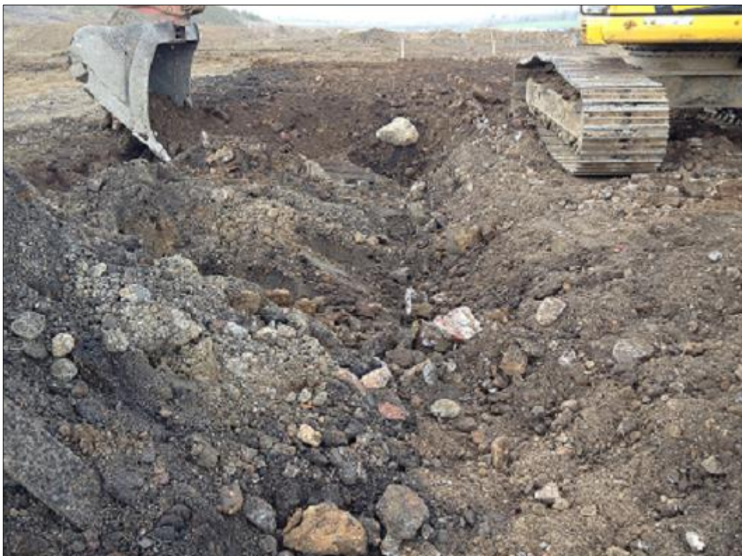
16) SB22 – Following clearance of remnant footing
