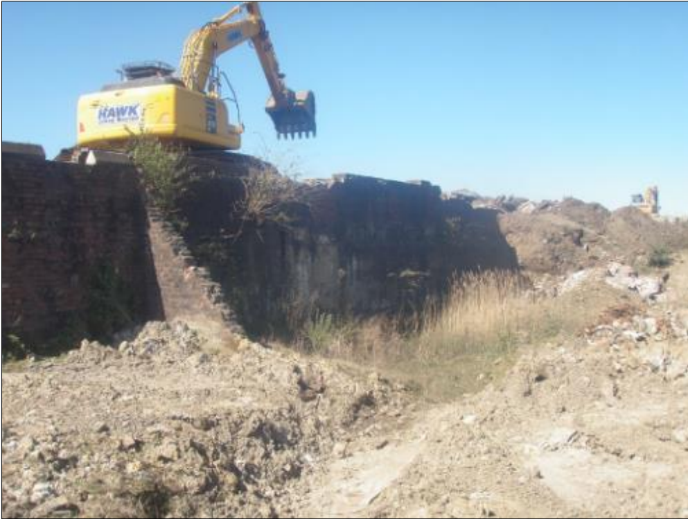
18) Back Retaining wall during demolition – see also photo (19)
