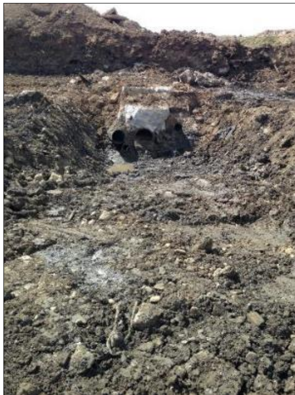
21) Pipe sections below concrete hardstanding – see photo (20)
