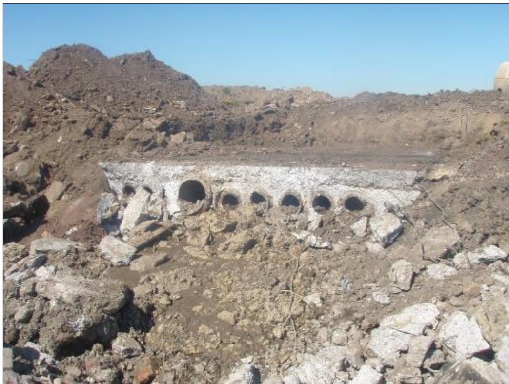
25) Pipe section running beneath hardstanding during removal
