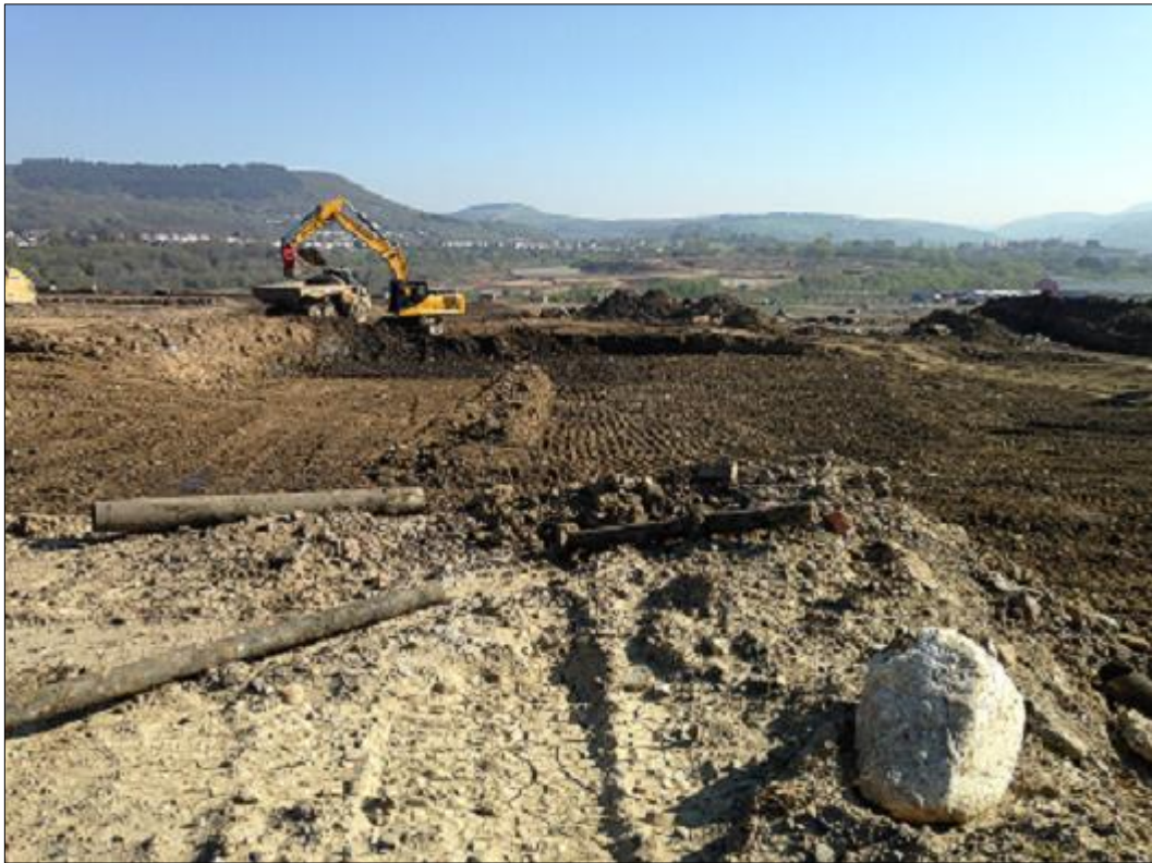
24) View during reclamation looking NE from approximately IP4141 position
