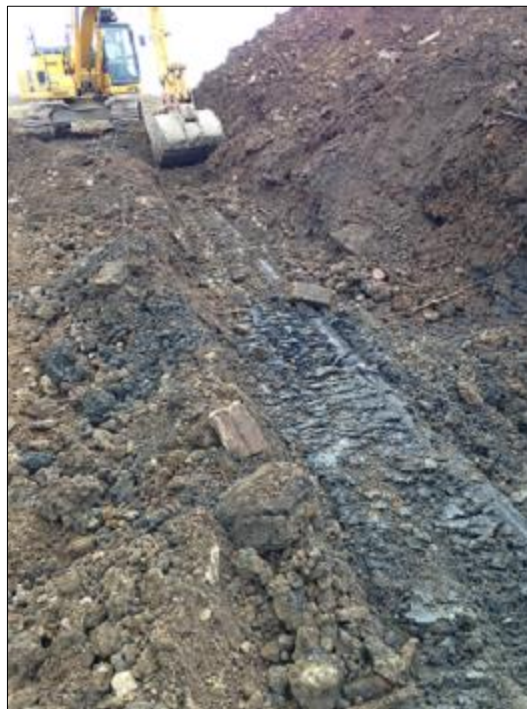
23) Exposure of pipe section prior to removal
