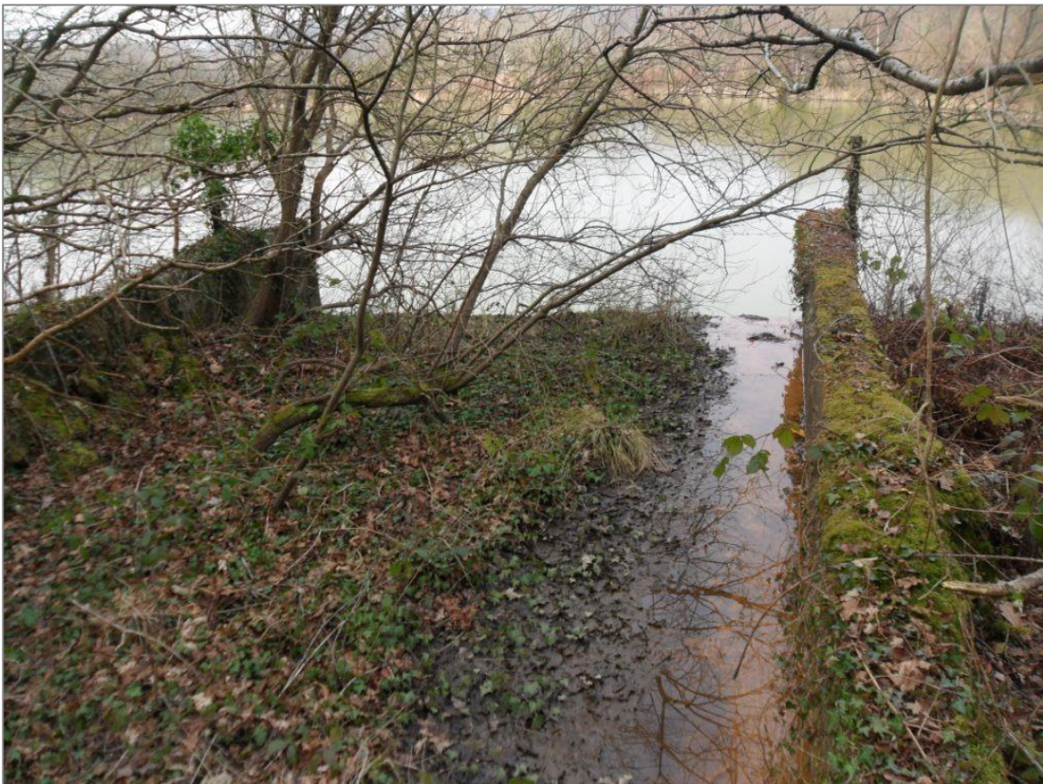
Photograph 22: Brick constructed spillway in to the SSR.
