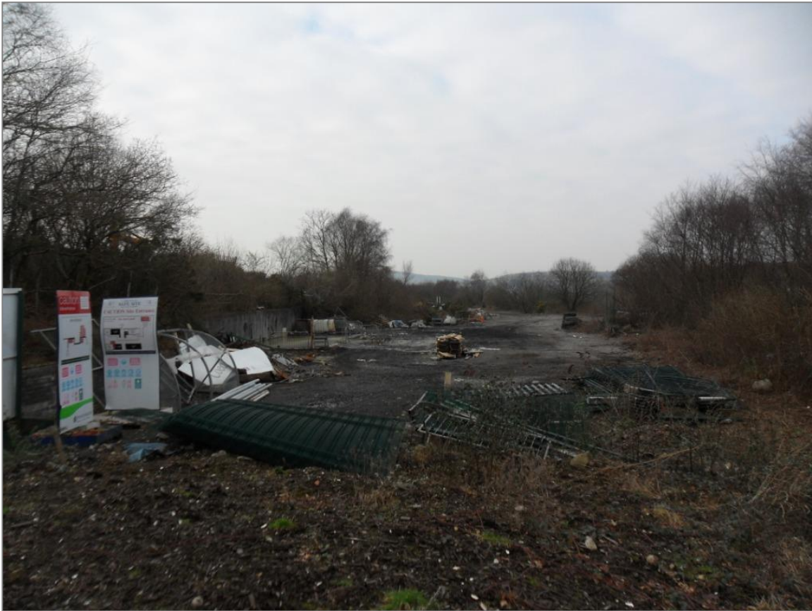
Photograph 15: Photo taken westwards on top of a degraded woodchip pile with miscellaneous anthropogenic inclusions in. Fencing and some broken materials noted on the hardstanding beyond the woodchip.
