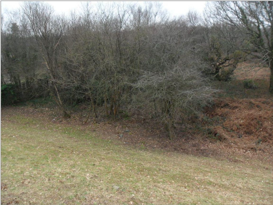
Photograph 5: Grassed bank of the NSR dam wall with dense scrubland from the toe of the slope.
