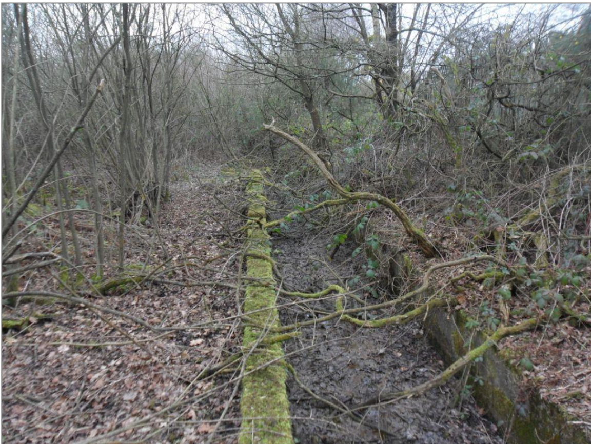
Photograph 10: Relic concrete based drainage channel in dense scrub and semi mature woodland.
