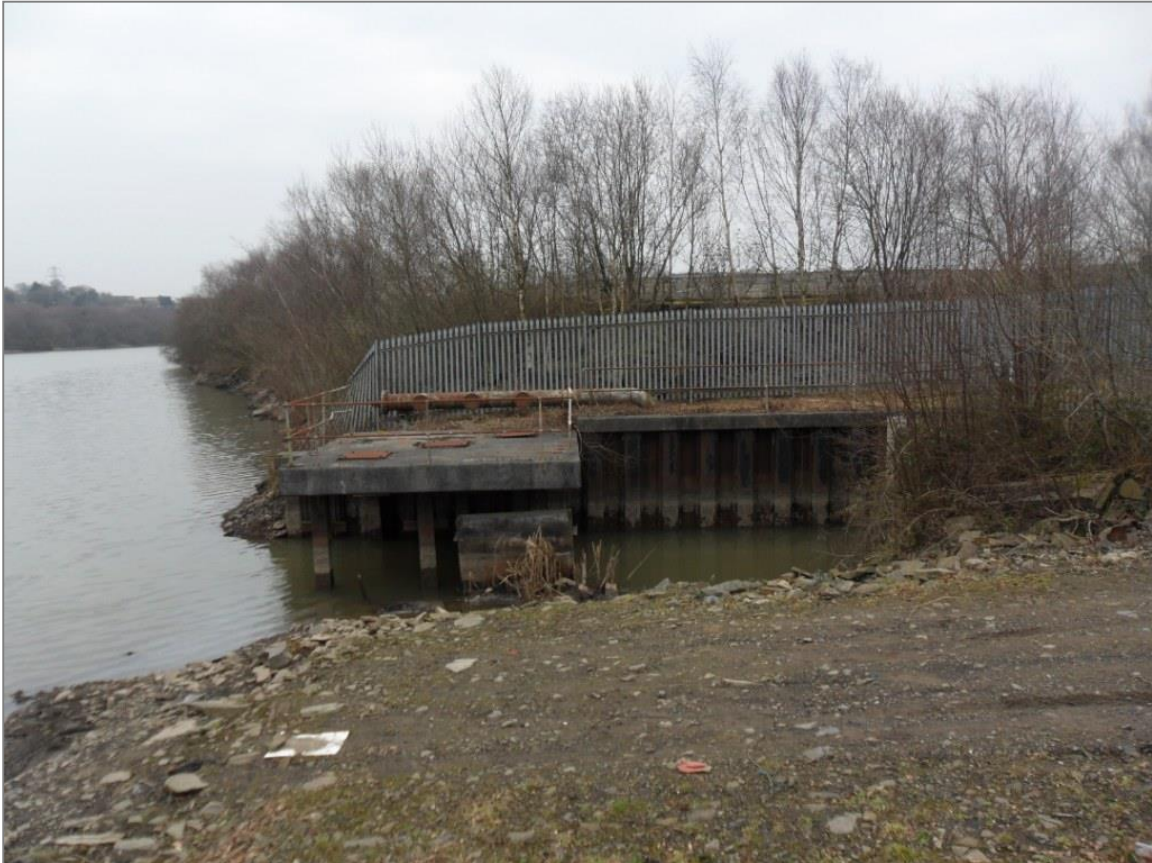
Photograph 3: Sheet piled jetty in the south eastern corner of the NSR. Structure fenced off for access on the eastern edge.
