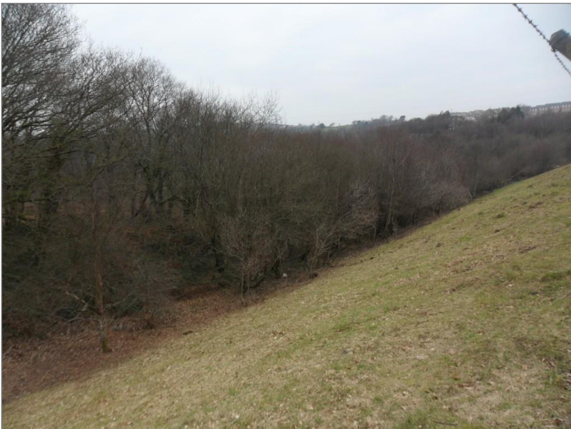
Photograph 6: Grassed bank of the NSR dam wall with dense semi mature woodland with thick scrub from the toe of the slope.
