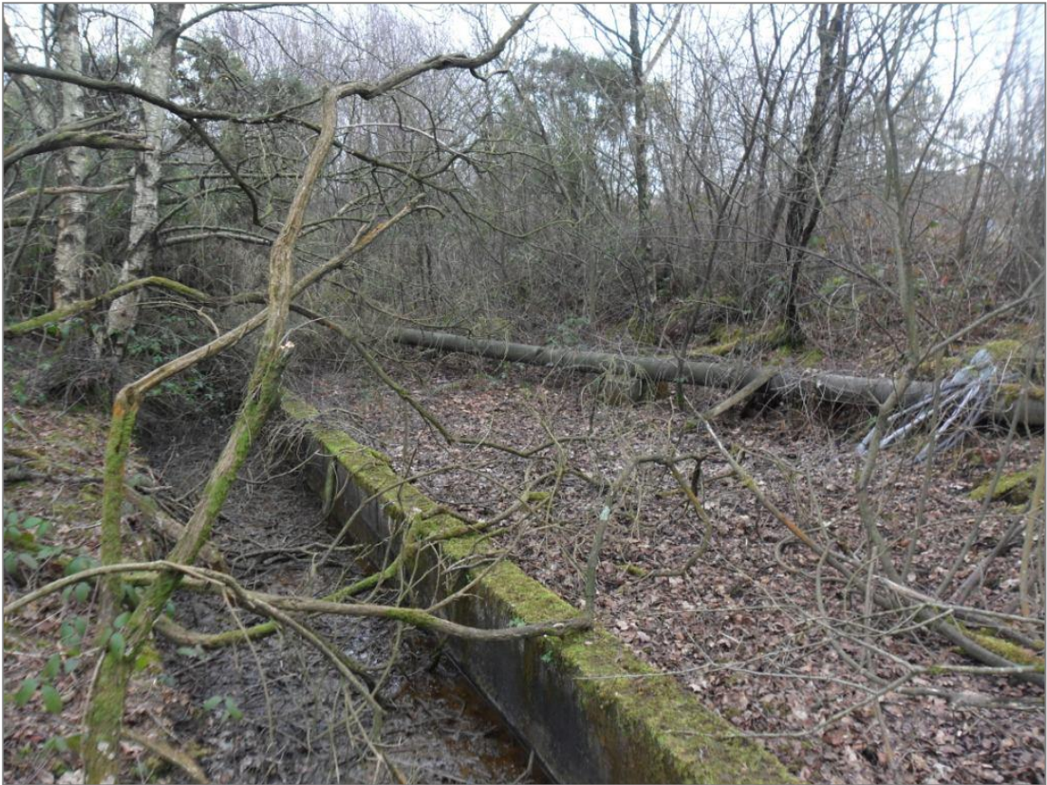
Photograph 11: Relic concrete based drainage channel with steel drainage pipe. Located in dense scrub and semi mature woodland.
