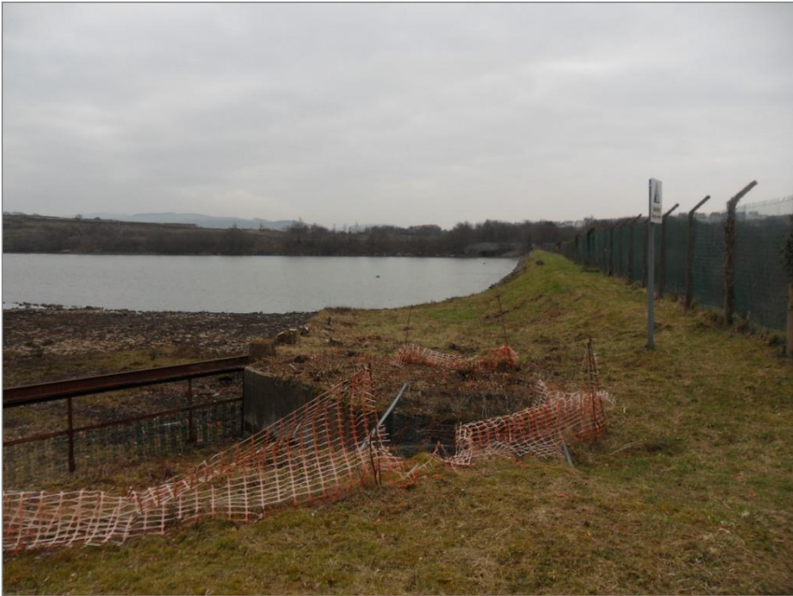
Photograph 7: Photo taken southwards along the NSR grassed dam wall next to the spillway.
