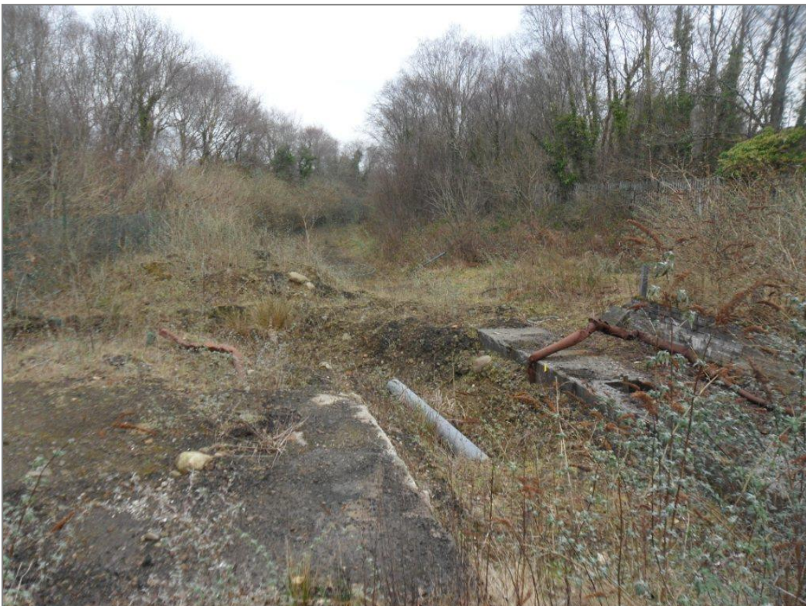
Photograph 14: Concrete culvert and some pipes in an overgrown area of scrub comprising brambles and buddlejia. Some small mounds of track scrapings were noted to be present.
