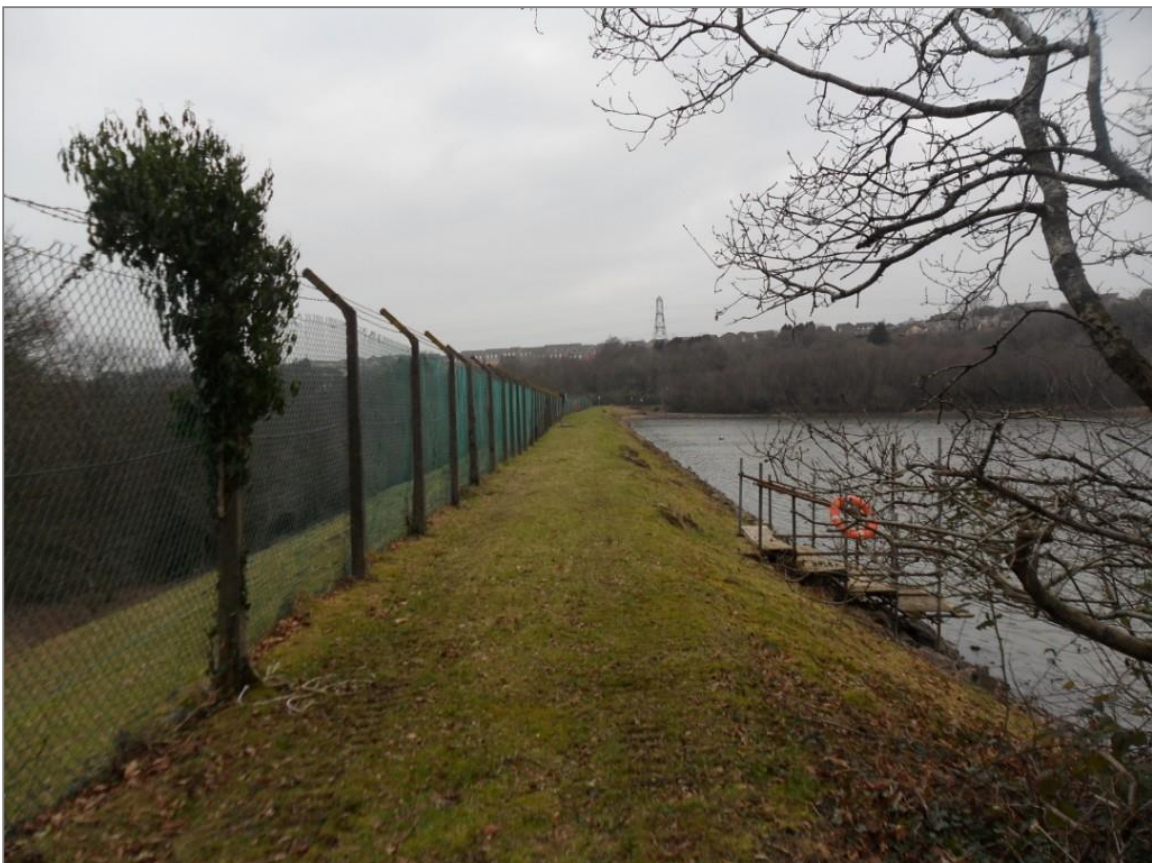
Photograph 4: Photo taken northwards along the NSR grassed dam wall.
