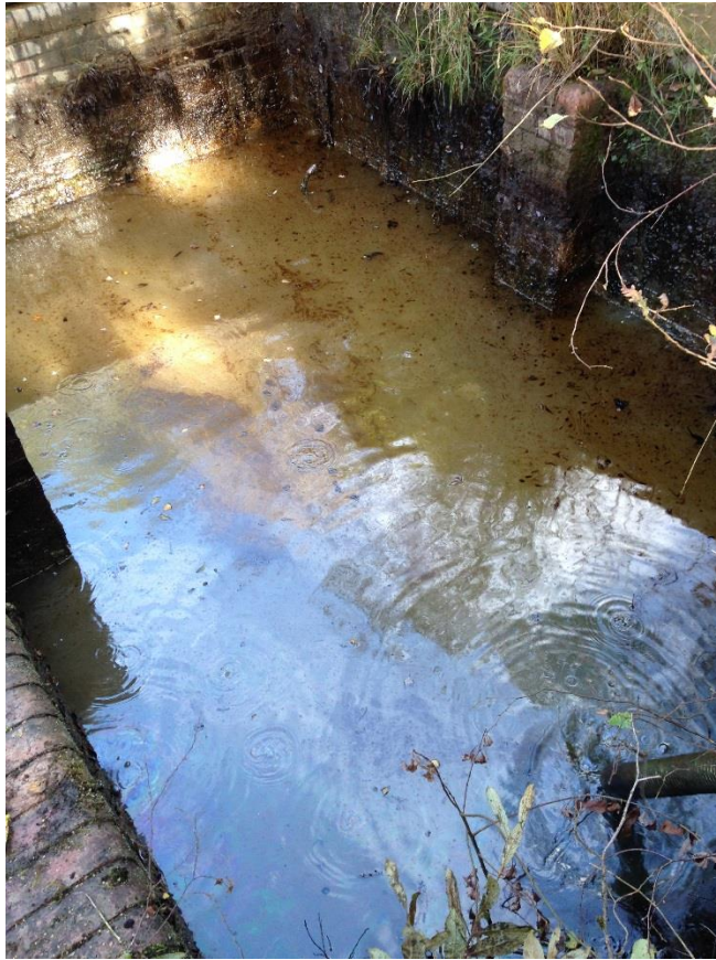
7) Removal of soil water and basal silts
