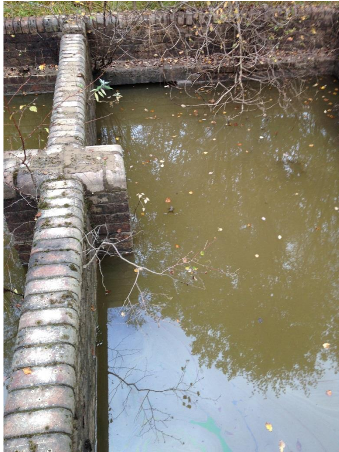
9) Water quality following recharge after recovery
