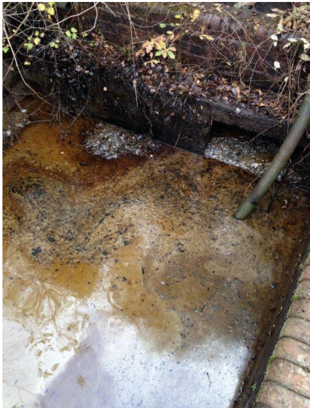
8) Removal of soil water and basal silts
