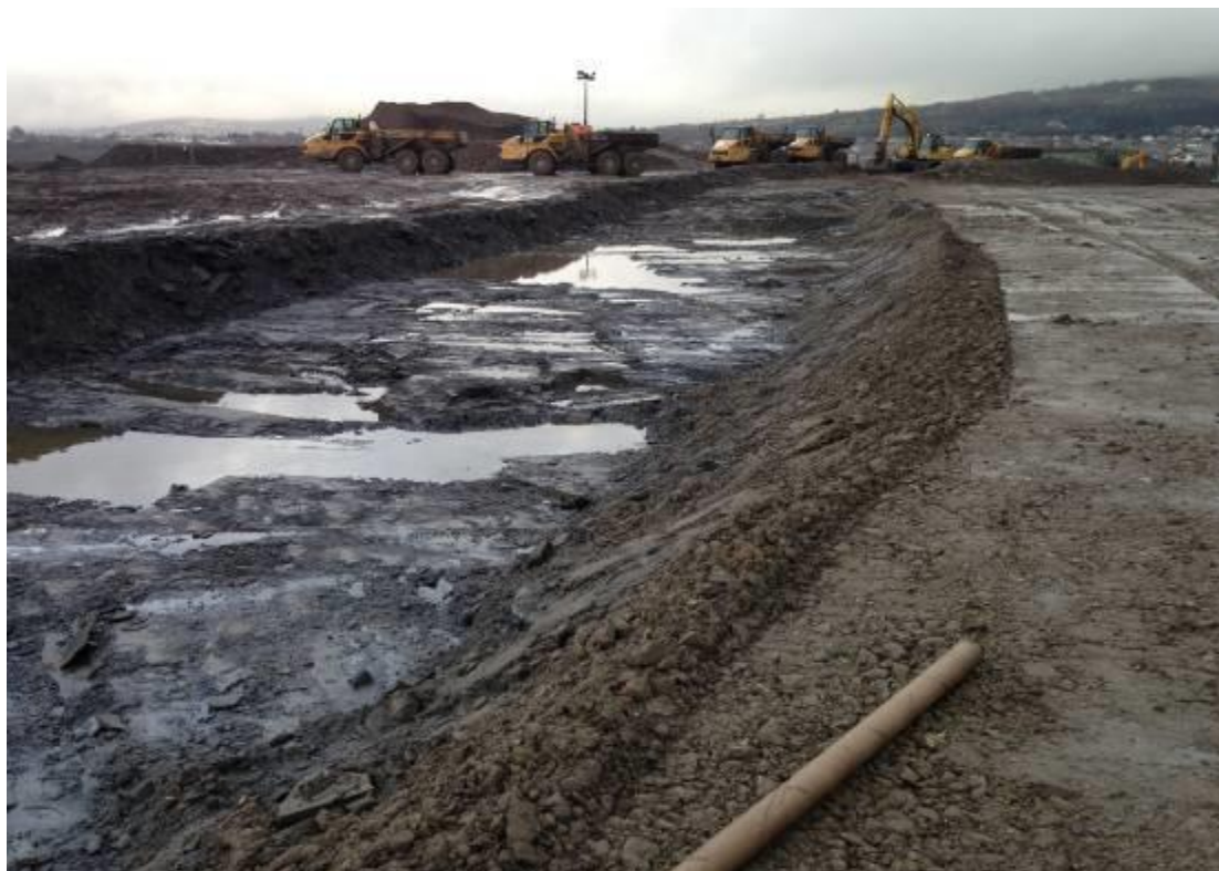
Photograph 7 – Showing the base of excavation on the bedrock on the left and backfilled material on the right.
