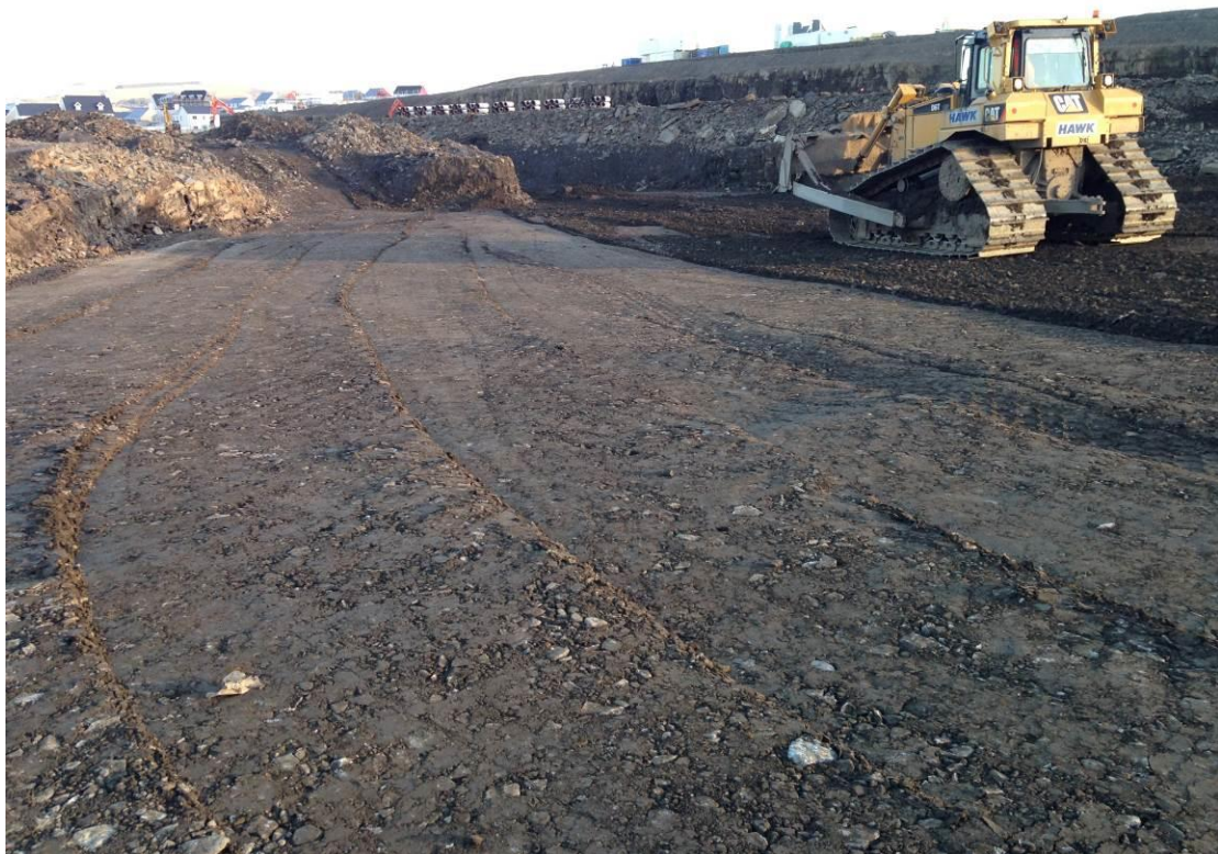
Photograph 14 – Showing the central area, note the material being rolled in to produce a level surface.
