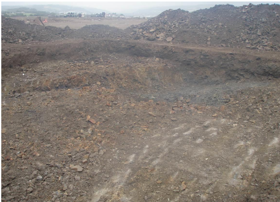
Photograph 10 – Showing IP4080 excavation, note shallow depth to bedrock.
