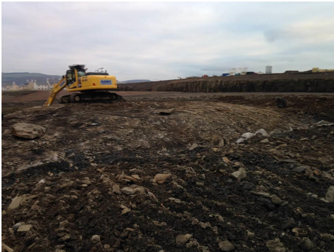
Photograph 11 – Showing the Northern area of MP32 excavated to bedrock
