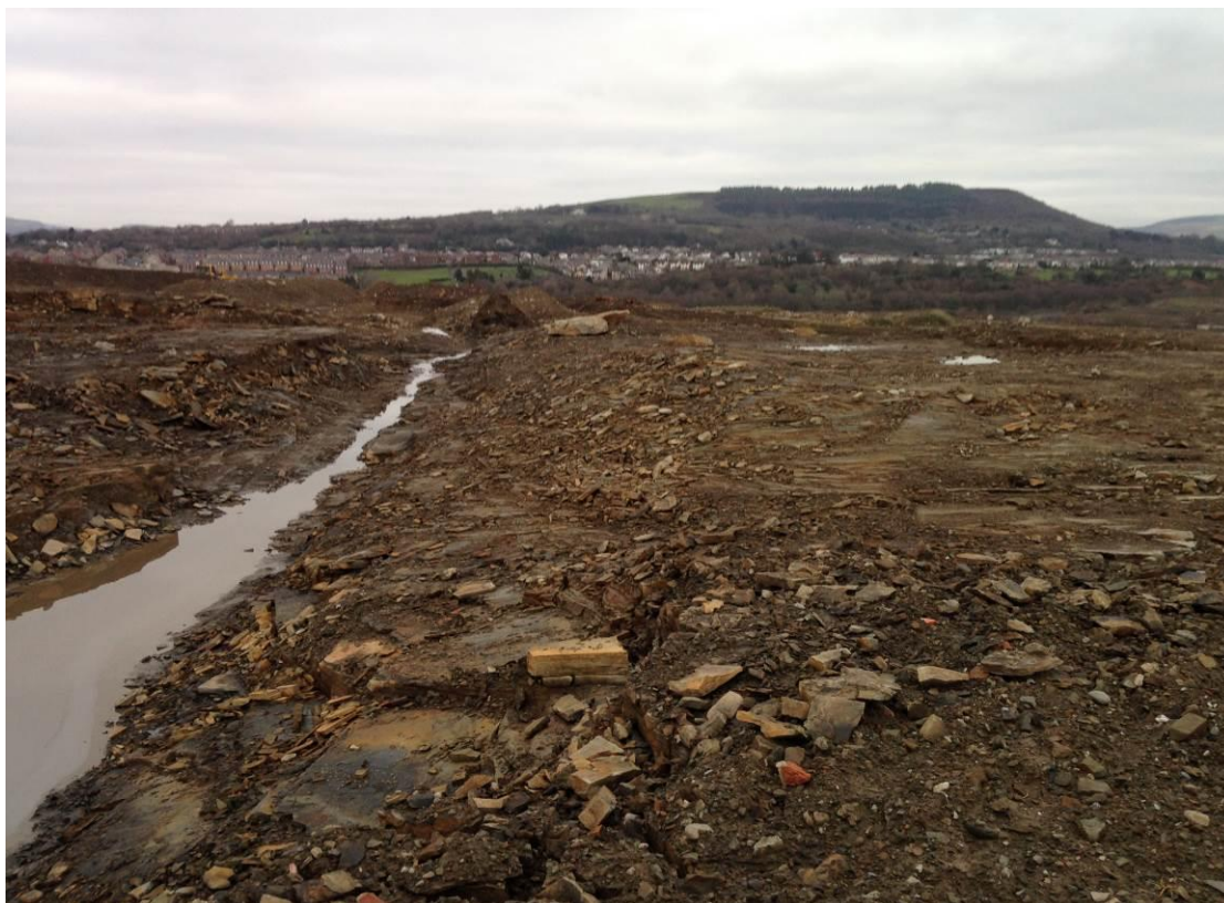
Photograph 12 – Showing the Northern area of MP32 excavated to bedrock with manmade drainage channels
