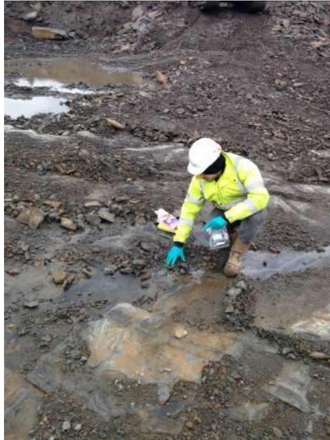
Photograph 1 – Showing the sandstone bedrock after the surface scrape.
