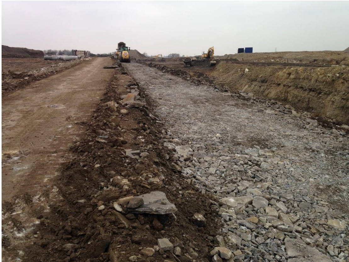
Photograph 13 – Showing the central area, note the material being rolled in to the divots and channels to produce a level surface.
