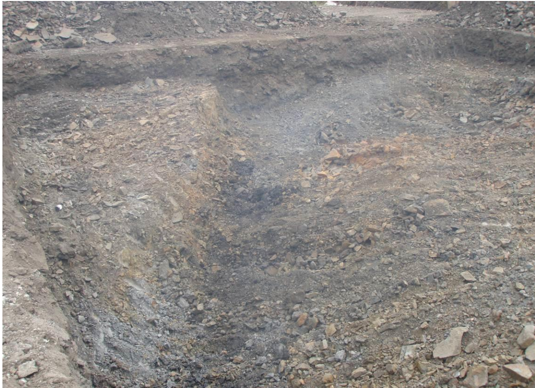
Photograph 9 – Showing the base of excavation IP4080, note the shallow depth to bedrock.
