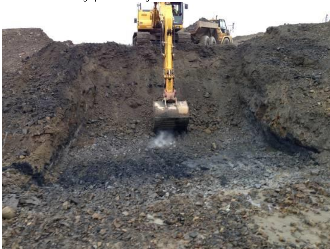
Photograph 6 – Showing the stained Made Ground above the natural bedrock which was removed during the initial work before the validated back fill.
