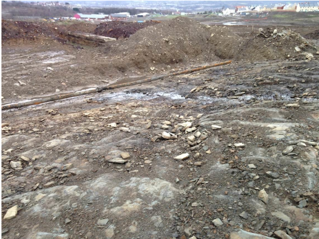
Photograph 15 – showing a north south running pipe located within a manmade recessed channel within bedrock.
