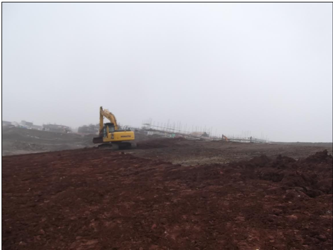
Photograph 6: Placement of shallow imported soils across Monitor Phase 31.
