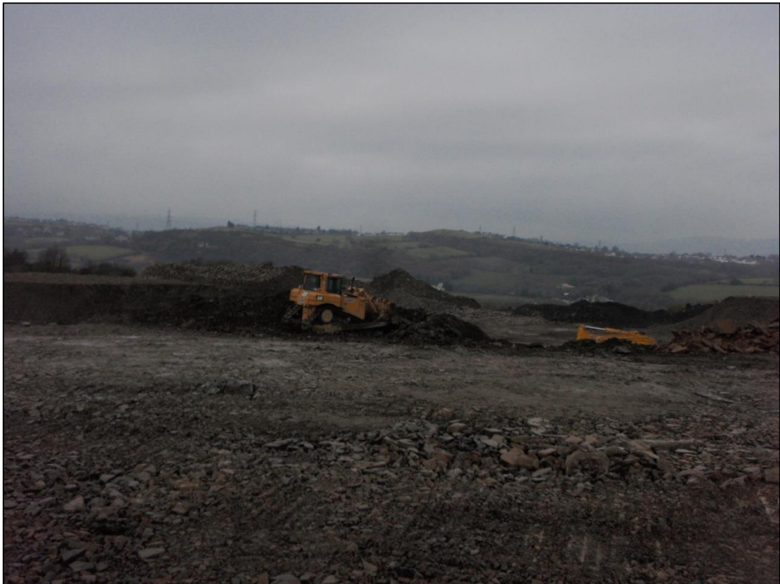
Photographs 5 and 6: Re-profiling of final surface to achieve the desired profile
