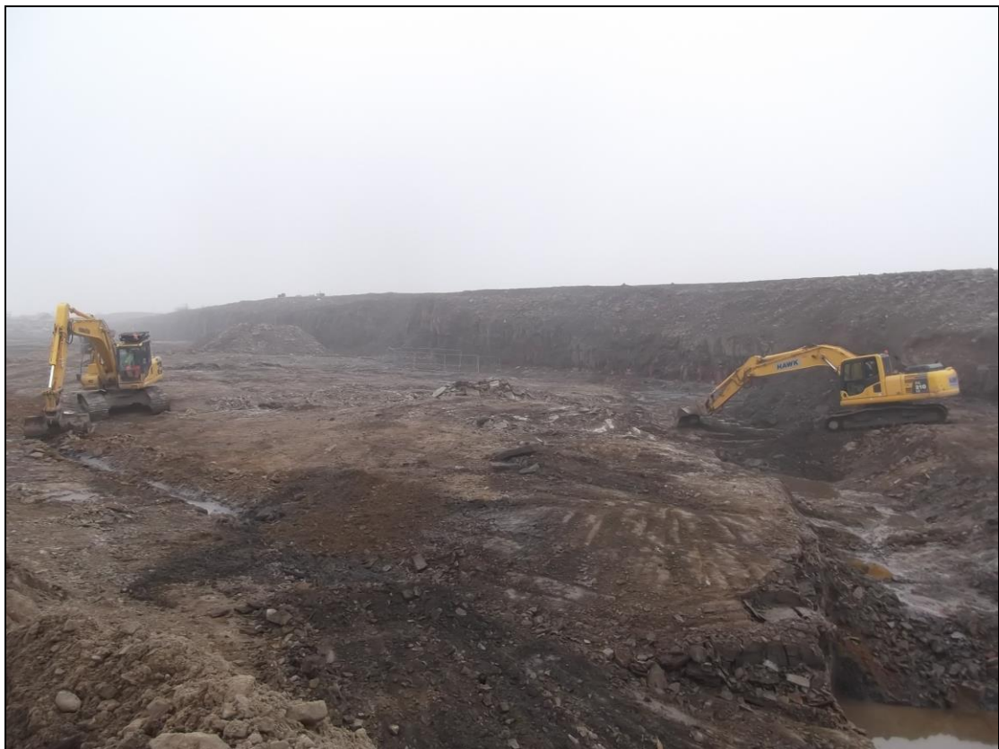
Photograph 3 and 4: Base of Excavation and benching of sandstone bedrock
