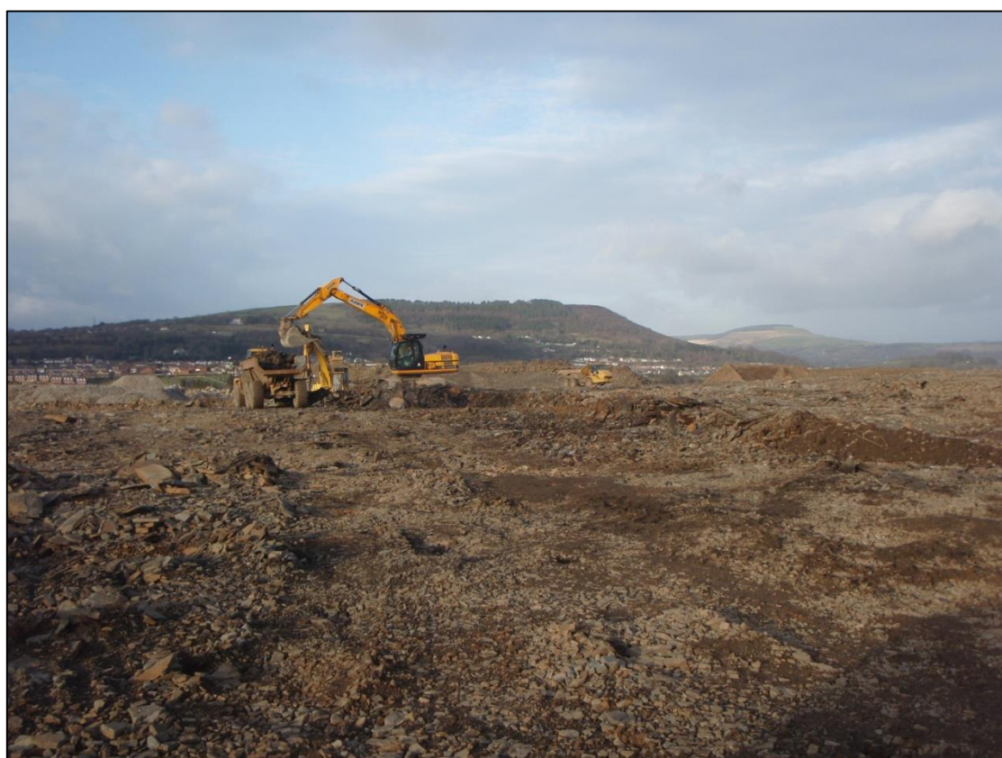
Photographs 1 and 2: Breaking and excavation of existing bedrock
