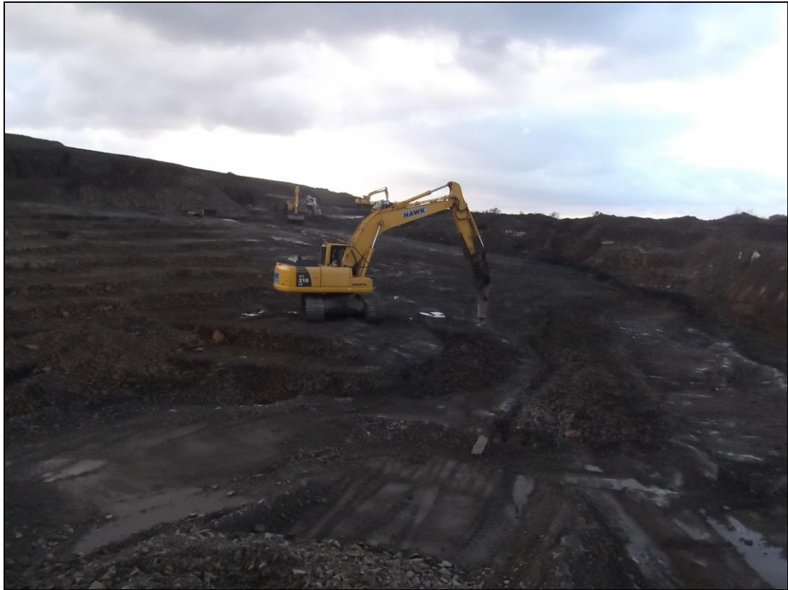
Photograph 3 and 4: Base of Excavation and benching of sandstone bedrock
