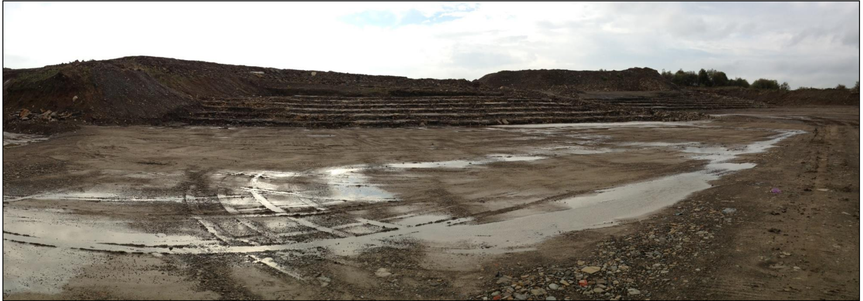
Photograph 6: Final 'stepped' profile along the northern boundary of Monitor Phase 30
