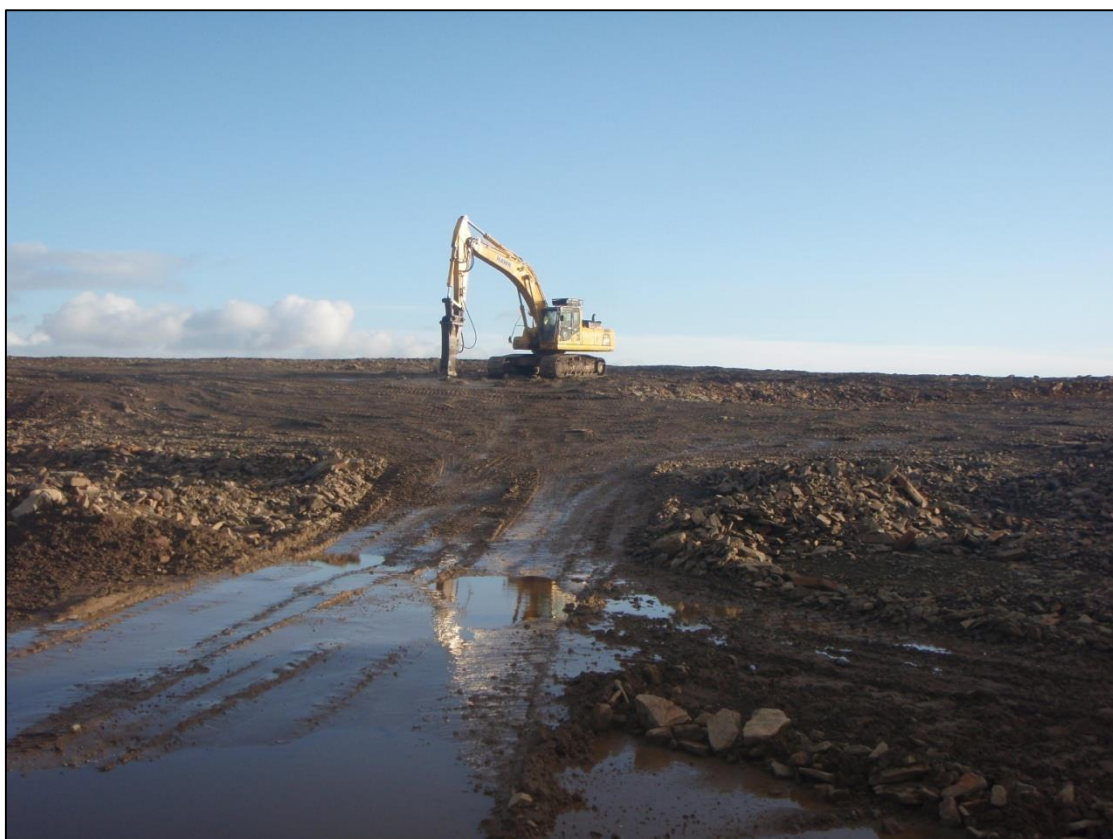
Photographs 1 and 2: Breaking and excavation of existing bedrock
