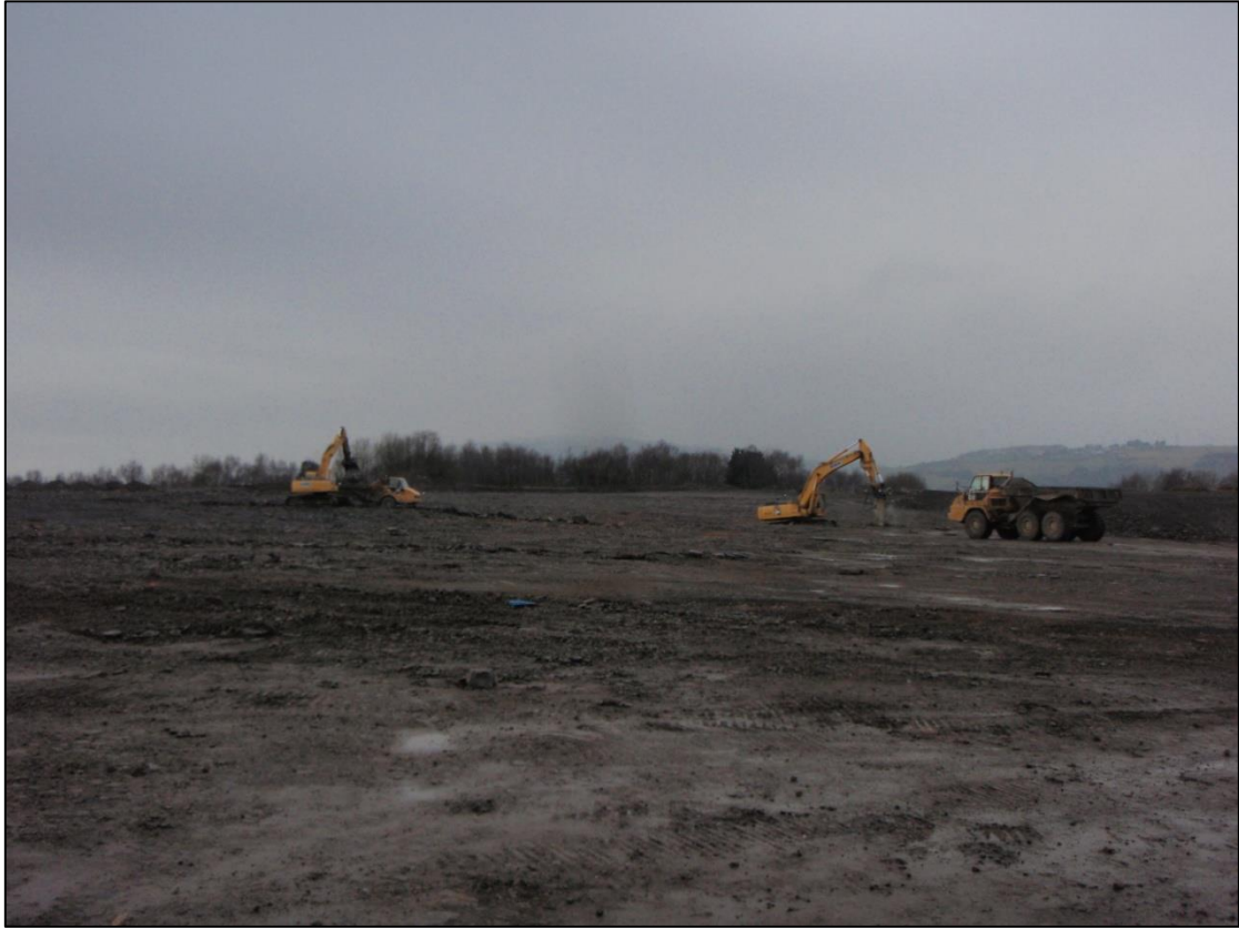
Photographs 5 and 6: Re-profiling of final surface to achieve the desired profile
