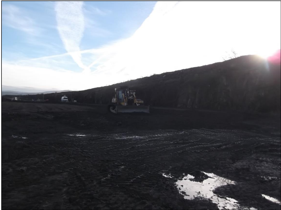
Photograph 5: Backfill of deep fill within excavations
