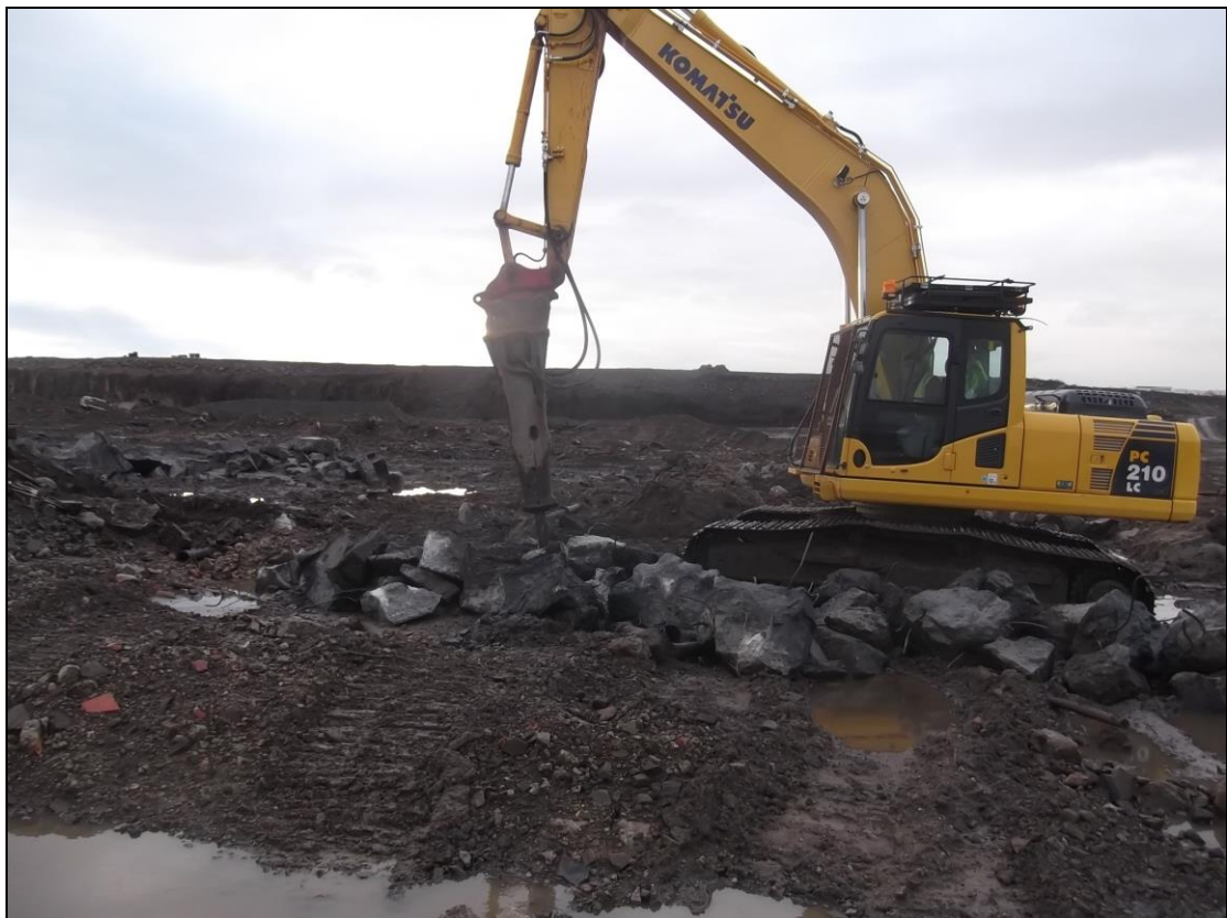
Photograph 1 and 2: Removal of impacted soils and concrete from Monitor Phase 31.
