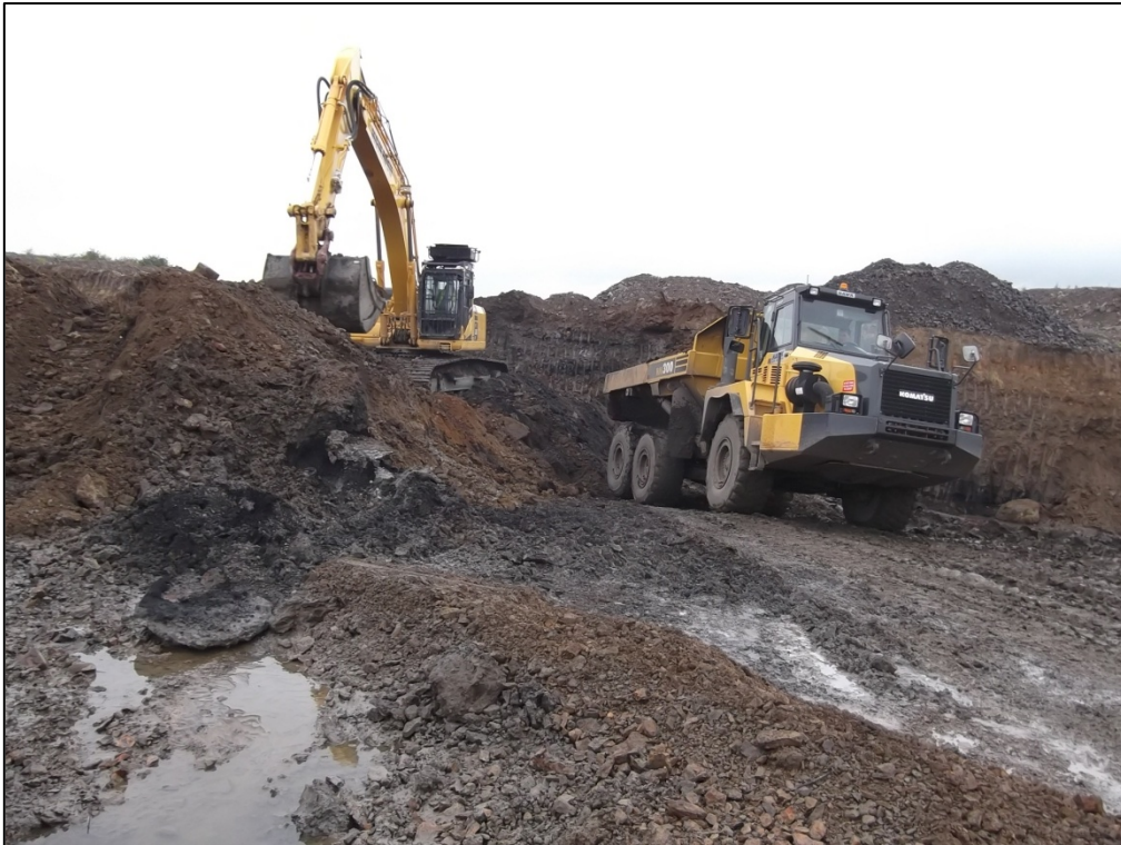
Photograph 1: Excavation of materials from within Monitor Phase 29
