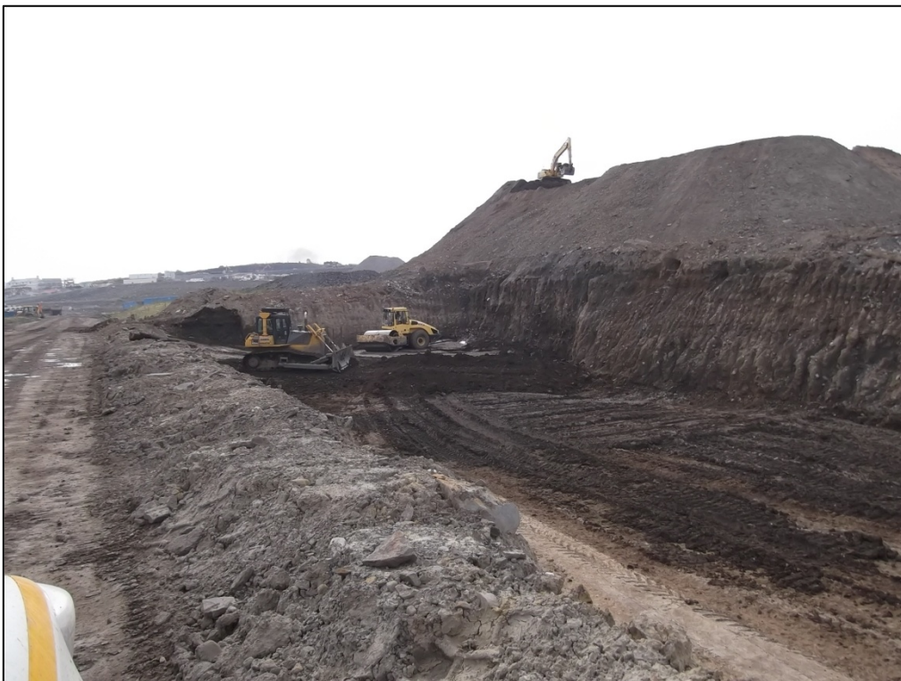
Photographs 2 to 5: Backfill of Monitor Phase 29
