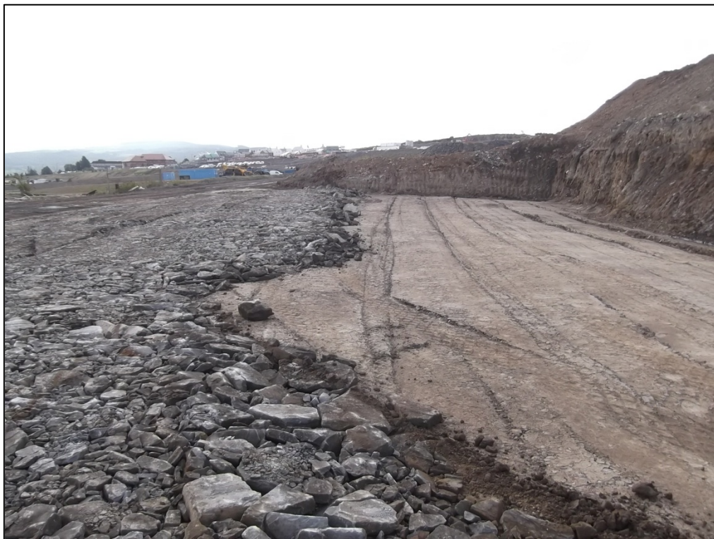
Photograph 6: Upfilling with top 0.5m of suitable fill materials
