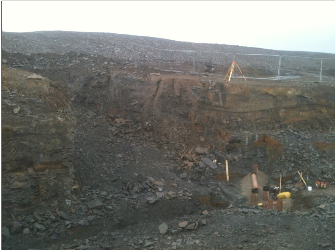
Photographs 5 and 6: Deep excavations for service installation into sandstone bedrock immediately to the north of Monitor Phase 22
