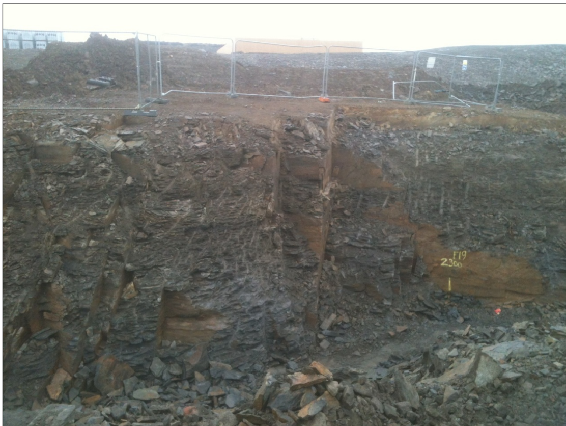
Photographs 5 and 6: Deep excavations for service installation into sandstone bedrock immediately to the north of Monitor Phase 22
