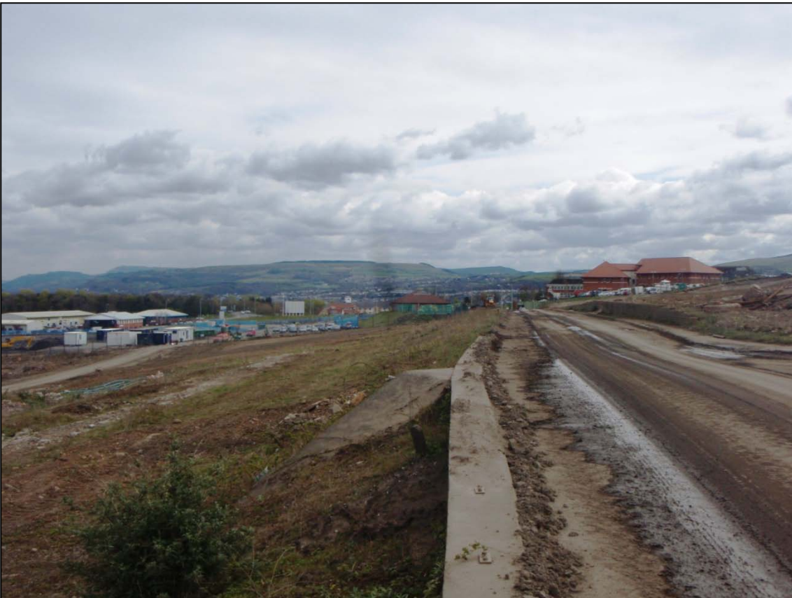
Plate 4 Looking east along an existing road which borders the study area to the south
