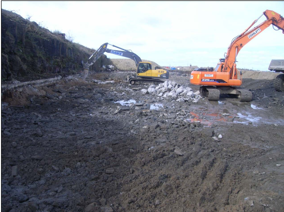
Photograph 5: Middle Terrace obstruction removal in 2011. Exposed rock face evident on the left.
