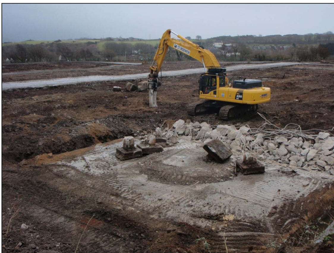
Photograph 2: Obstruction and hardstanding clearance of the upper terrace in 2009
