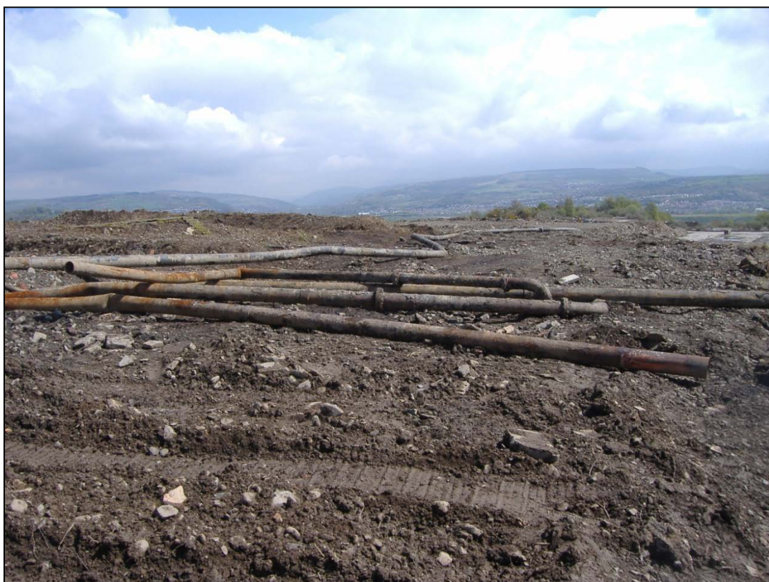
Photograph 4: Pipeline removal from the Cooling towers area 2008
