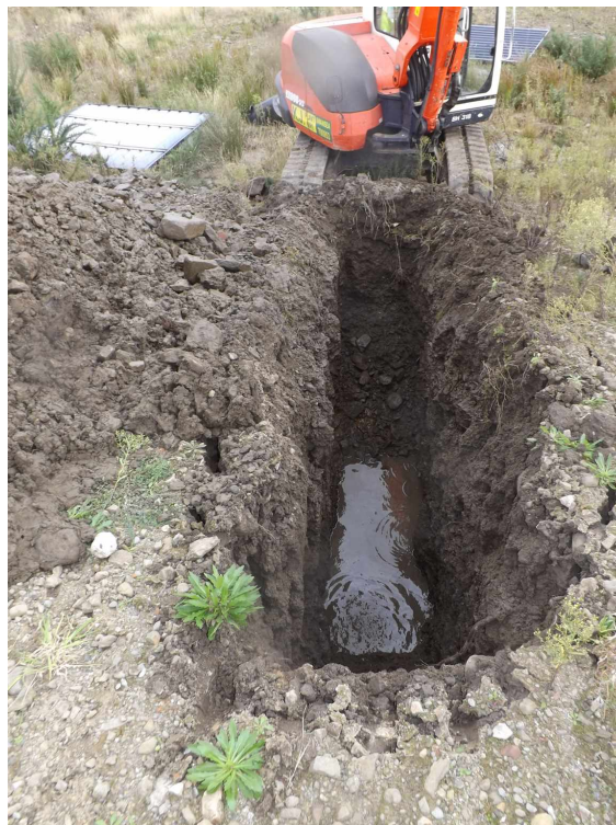
TP49 length and spoil
