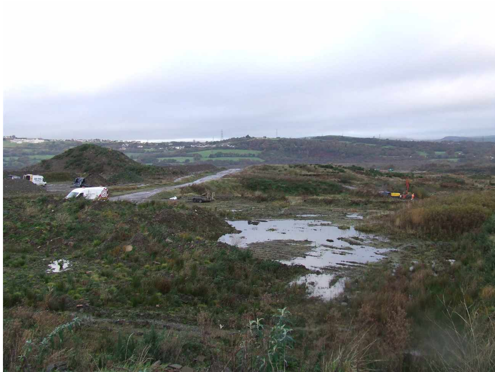
South site facing N facing BH23 & BH22
