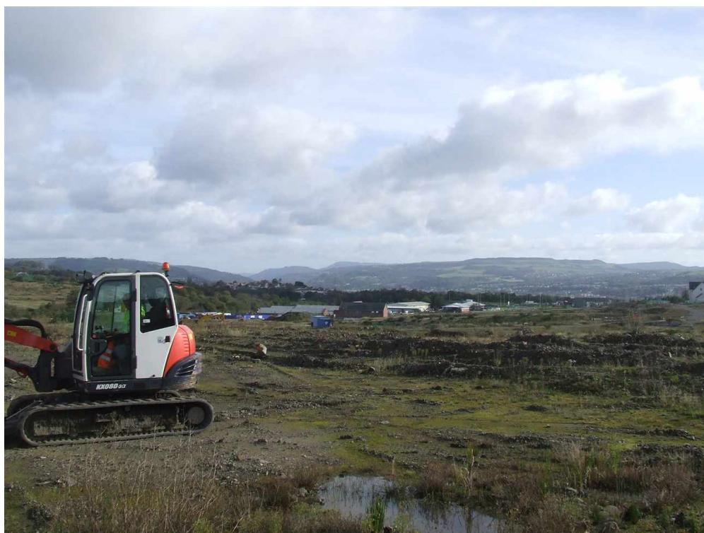
North site facing NE
