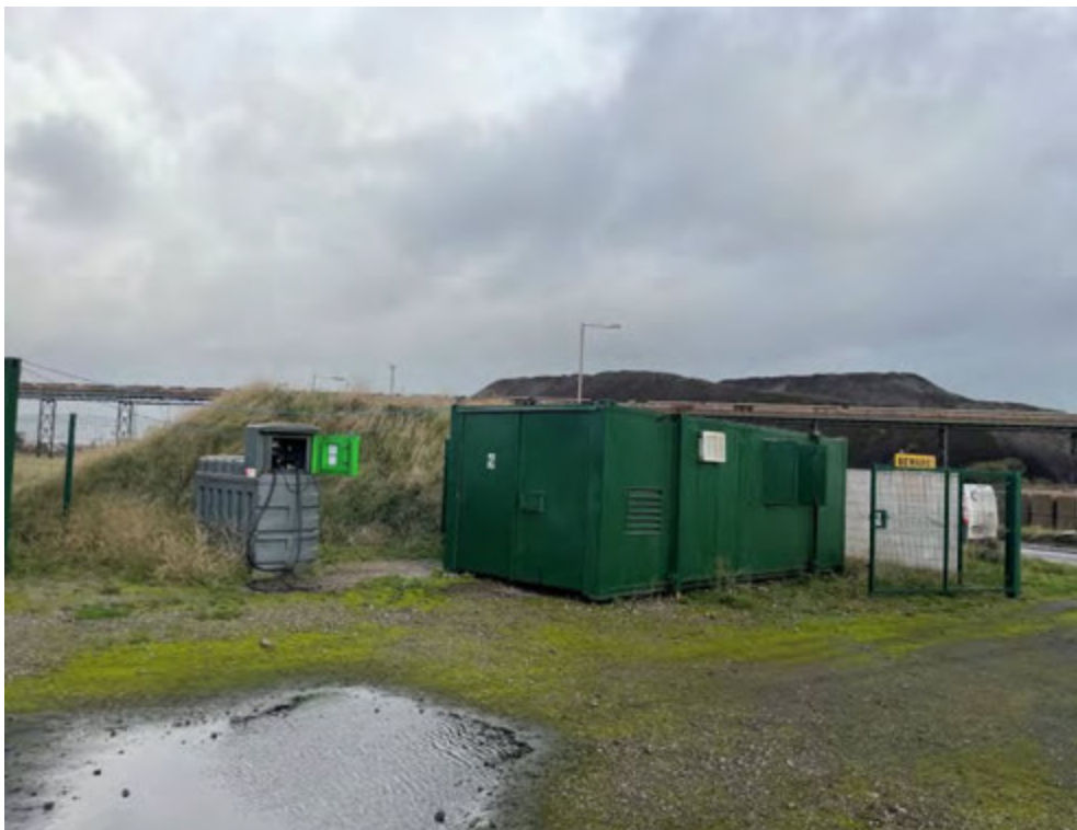
Photograph 2: View of existing containers located at the entrance of the compound, with bunded fuel storage tank, facing north-west.
