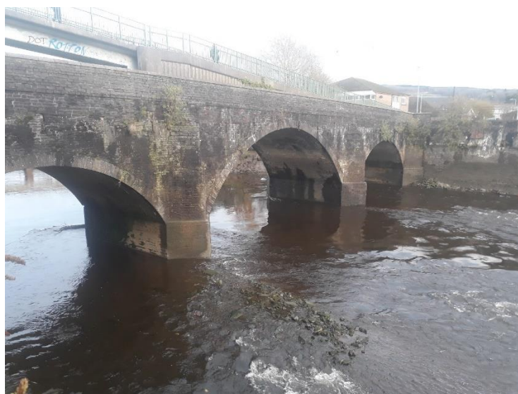
Figure 2 – A465 Neath Masonry Arch
