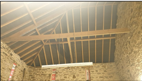
Photo 5 – Underside of Roof Detail, Looking (NW)
