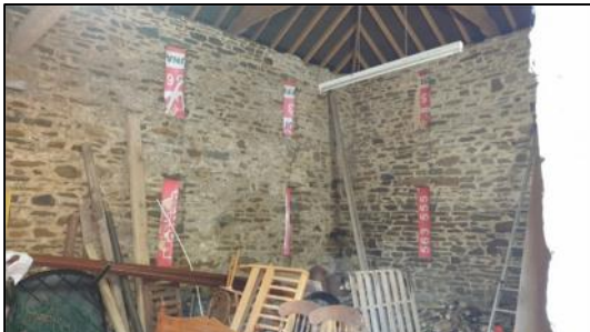
Figure 17 – Well-sealed Windows (NW)
