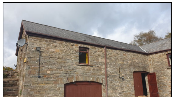
Photo 15 – (S) Section of Barn with Dedicated Window and Double Door – Not Surveyed
