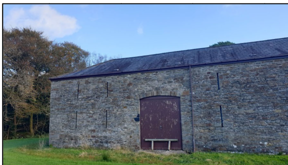
Photo 14 – (W) Aspect of the Building Showing Excellent Condition of Roof Slates and Masonry
