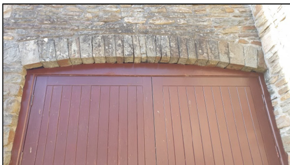
Photo 12 – Small gaps between stones of Semi Circular Arch above (E) Barn Door Visible
