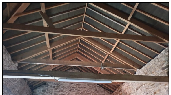
Photo 6 – Underside of Roof Detail, Looking (S)
