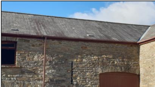
Figure 15 – Slates in Excellent Condition
