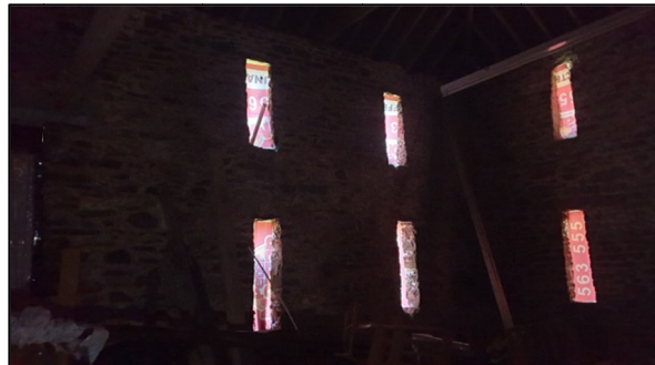
Photo 8 – (NW) Corner of Room when Strip Lighting is Turned off. Some Natural Light can be Seen Entering via the Translucent Plastic Sheets
