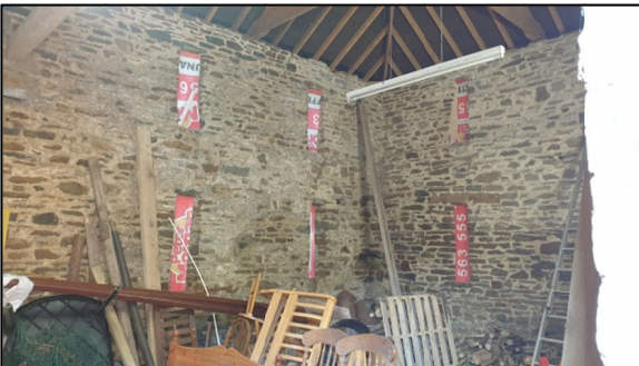
Photo 7 – (NW) Corner of Room when Strip Lighting Turned on. Plastic Sheeting used to Block the Slit Windows is Visible, Tightly Sealing the Windows
