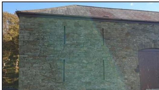
Figure 18 – External view of Sealed Windows (NW)
