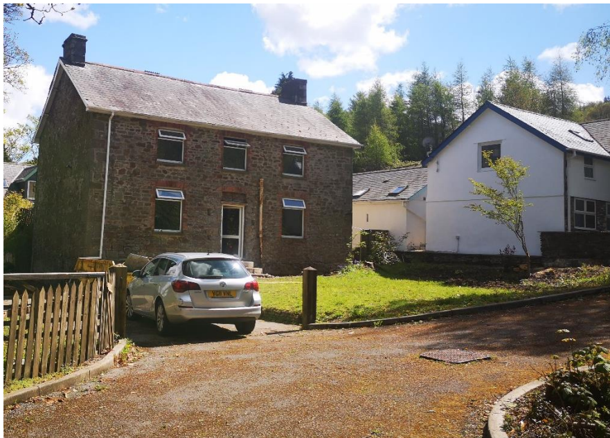
View from Driveway
