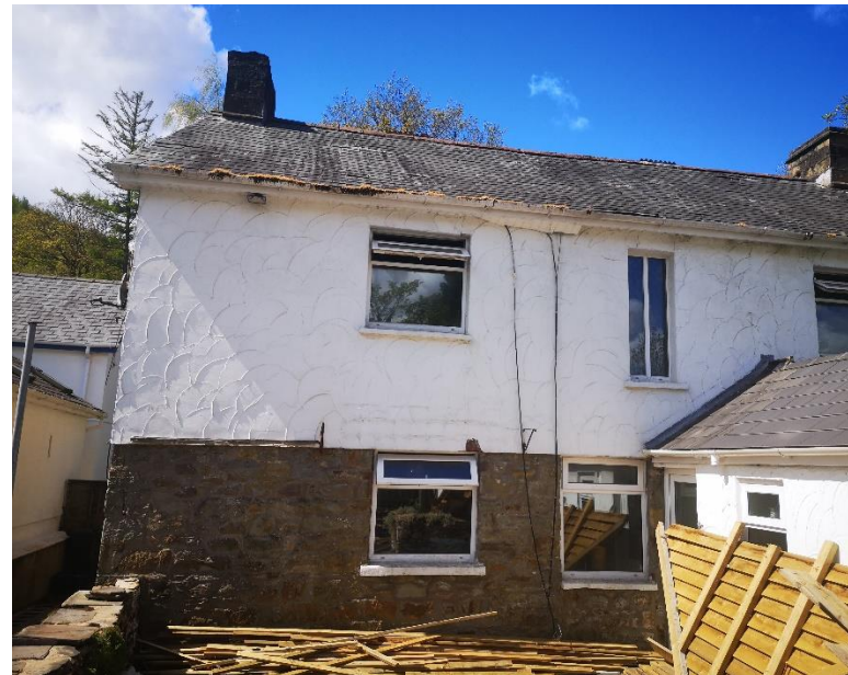
View from rear of property
