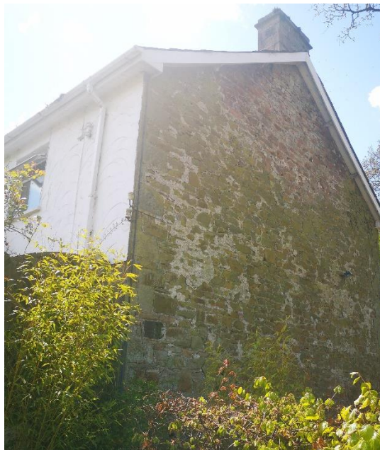
View of the stonework (North facing elevation)
