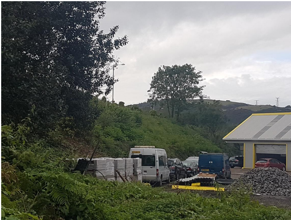
Plate 3 – Western boundary of the site
