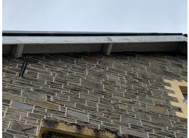
Photo 16: Gap in Timber Soffit of Extension on the North-Western Elevation
