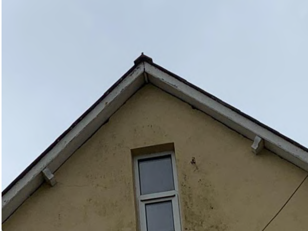
Photo 15: Gap in Timber Soffit of Care Facility on South-Eastern Elevation
