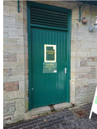
Figure 2, Typical Courtyard Door
