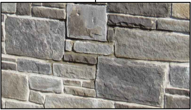
Stone Cladding: Blue Pennant Stone – Semi Coursed
