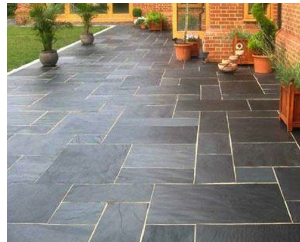
Paving to Driveway & External Paths
