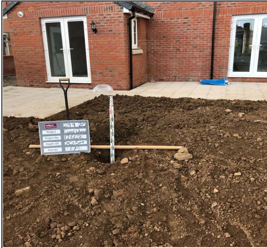
Plot 17 Capping Depth Check
