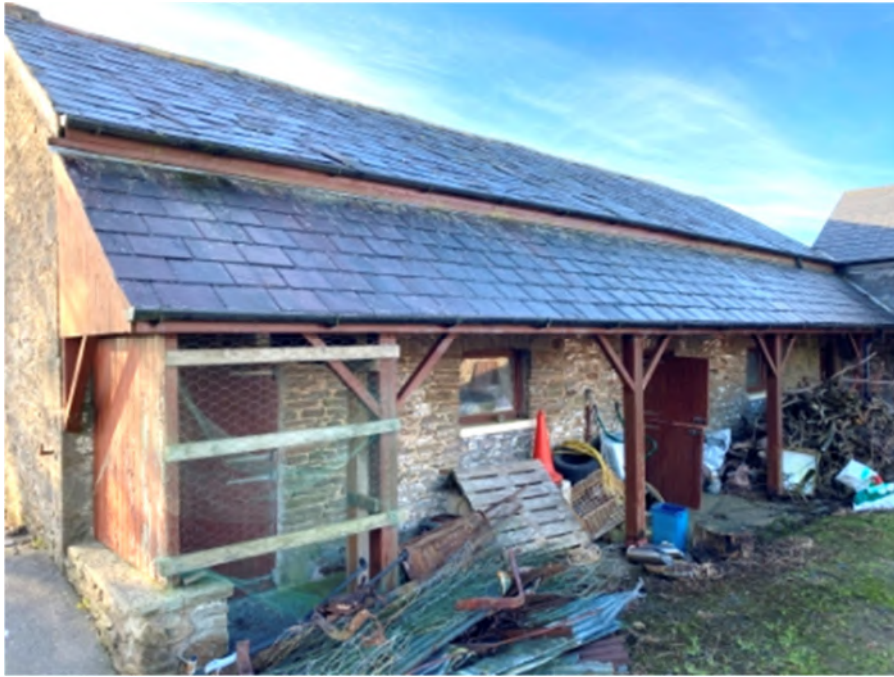
Photograph 53: View of north elevation canopy structure.
