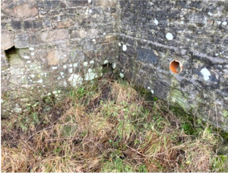
Photograph 11: View of drainage pipes discharging through west gable elevation.
