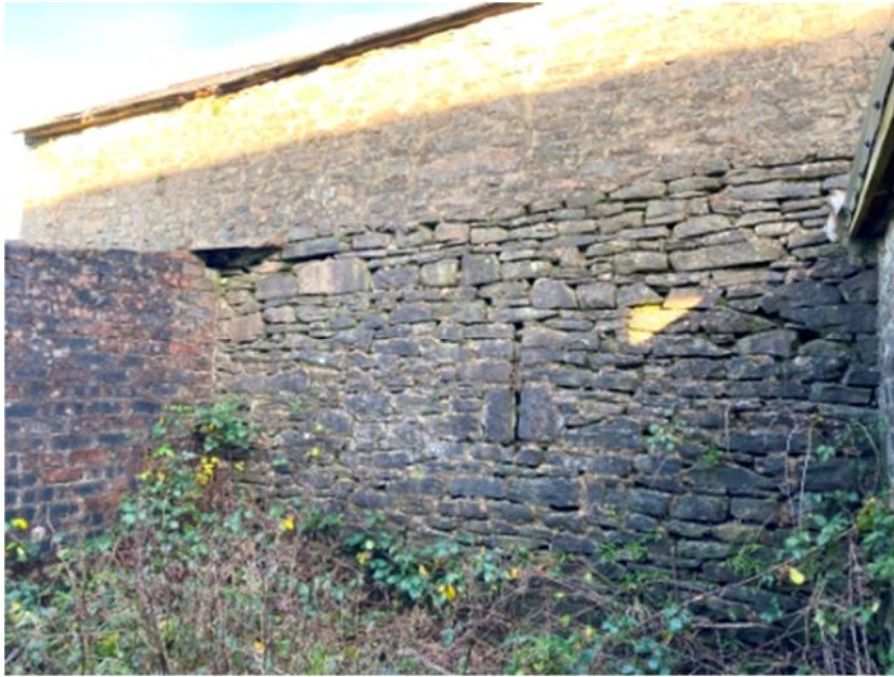
Photograph 29 : View of outer face of barn southern elevation from inside cow shed area.
