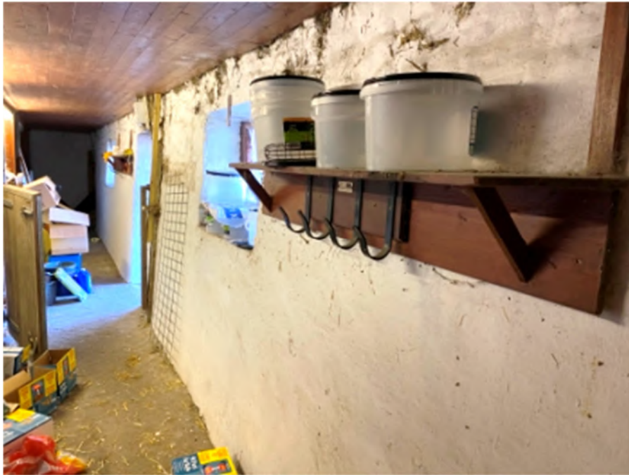
Photograph 47: Second view along the length of the barn north elevation wall with significant outwards lean. No cracking is noted within the wall construction.
