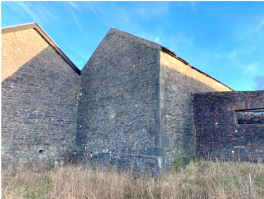
Photograph 8: View of barn west gable elevation and part cow shed elevation.
