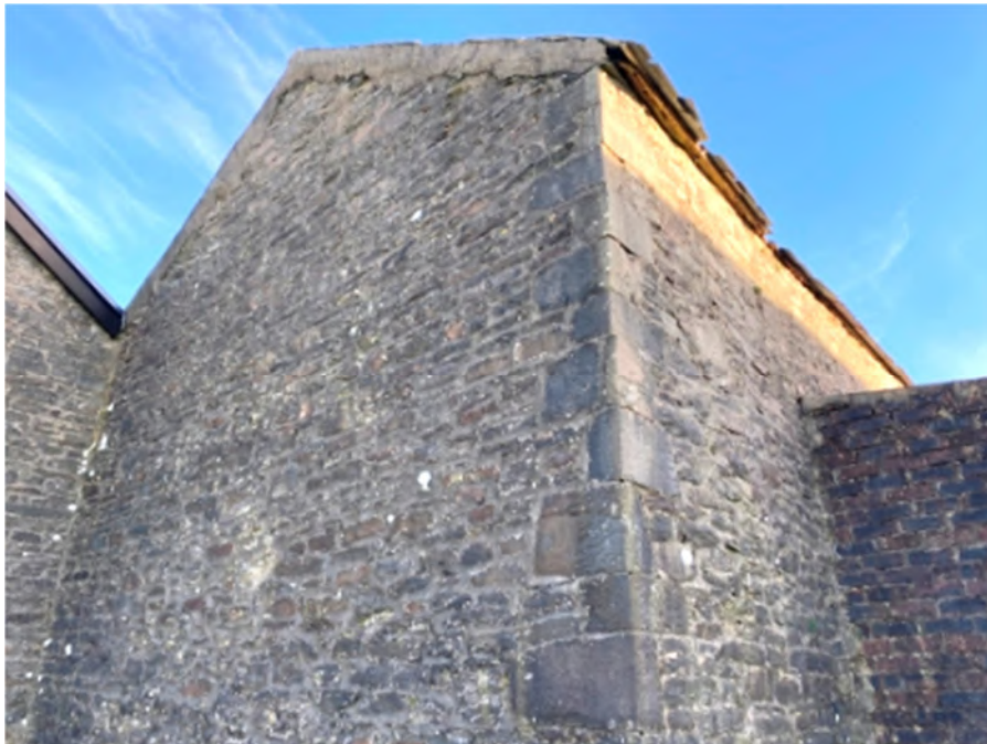
Photograph 10: View at junction of stone barn west gable elevation.
