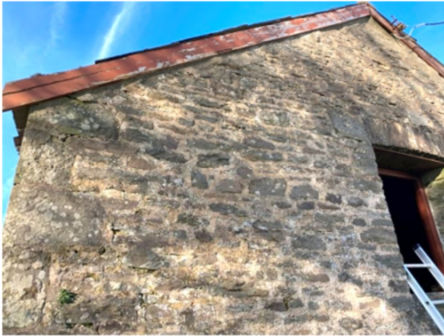
Photograph 33: View of barn east elevation. Stonework is in good condition with no cracking.
