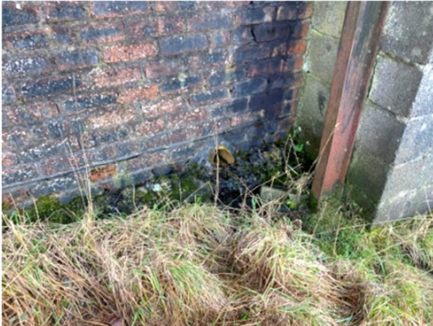
Photograph 12: View of drainage pipe discharging through cow shed west elevation.
