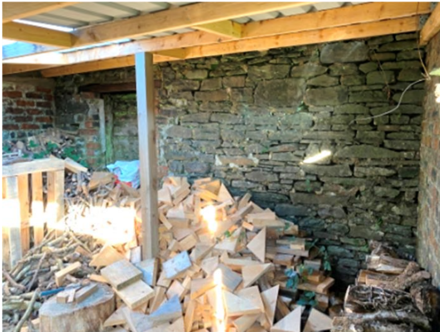
Photograph 30 : Second view of barn south elevation from inside cow shed.
