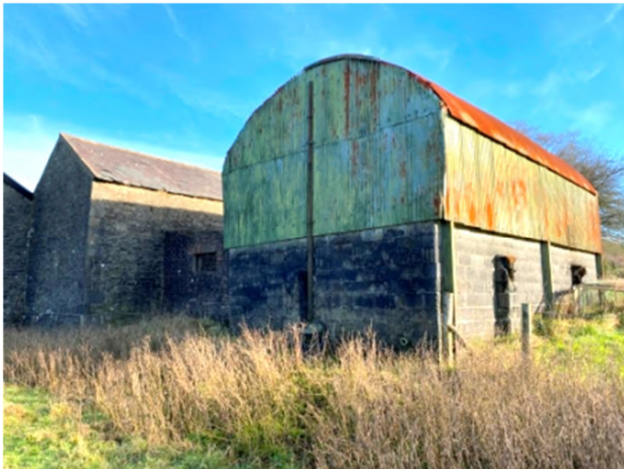
Photograph 6: View from south west corner showing Dutch barn and gable elevation of barn building.
