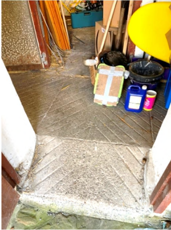
Photograph 45: Barn has a concrete ground bearing slab construction.
