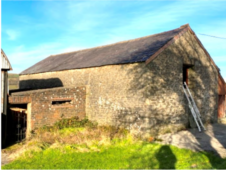
Photograph 3: View of barn south elevation. No openings in this elevation.
