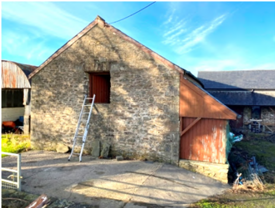
Photograph 2: View of eastern gable elevation of barn building with single opening allowing access to first floor level.
