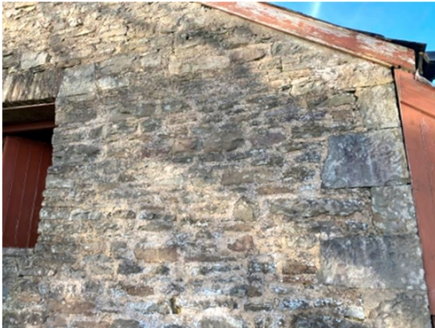
Photograph 34: Second view of barn east elevation. Stonework in good condition.
