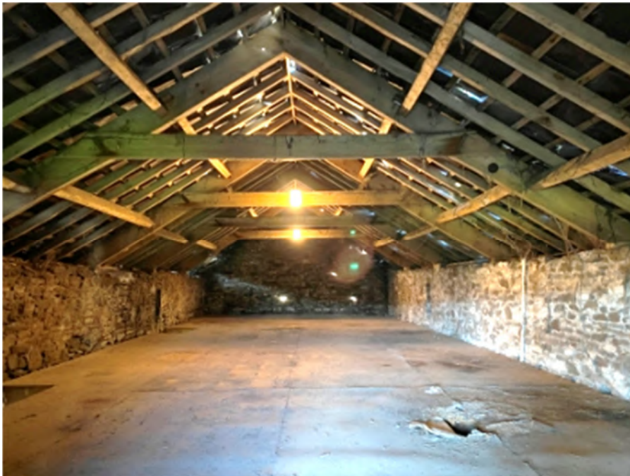
Photograph 38: View of barn roof structure consisting of timber rafters, purlins and A-frame trusses.
