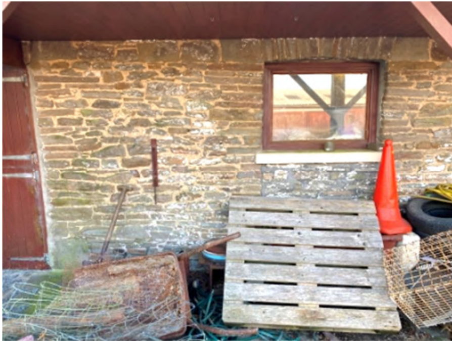
Photograph 35 : Part view of barn north elevation (courtyard). No cracking noted externally.
