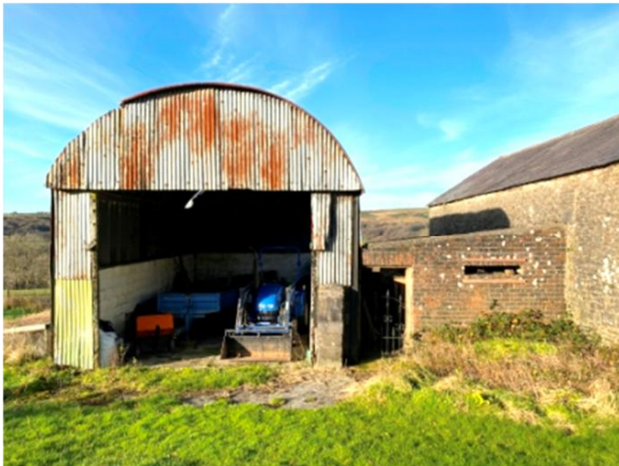
Photograph 4: View of east elevations of Dutch barn and cow shed structure which butts up against the main barn building.
