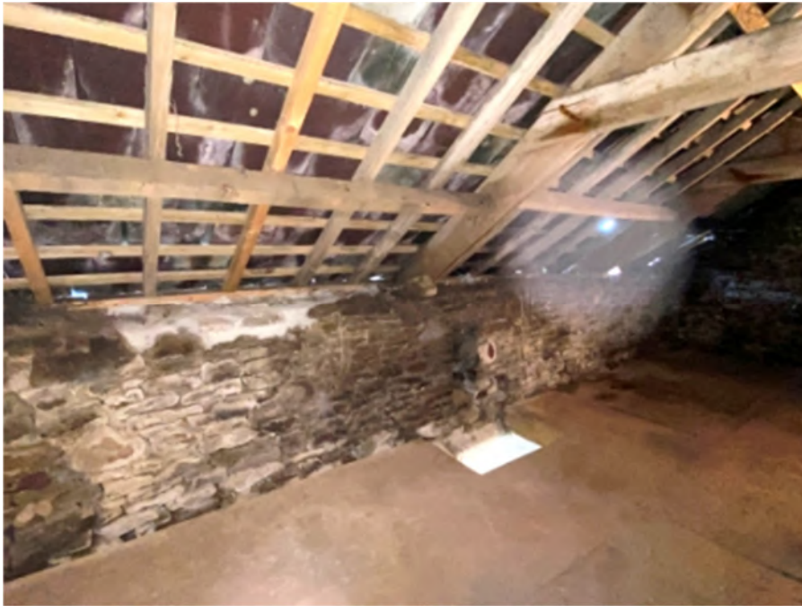
Photograph 41 : All stone walls at first floor level appeared stable with no sign of cracking.
