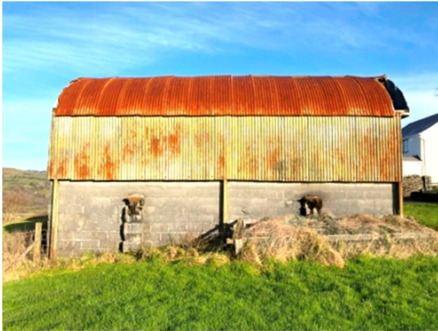
Photograph 5: View of Dutch barn south elevation.
