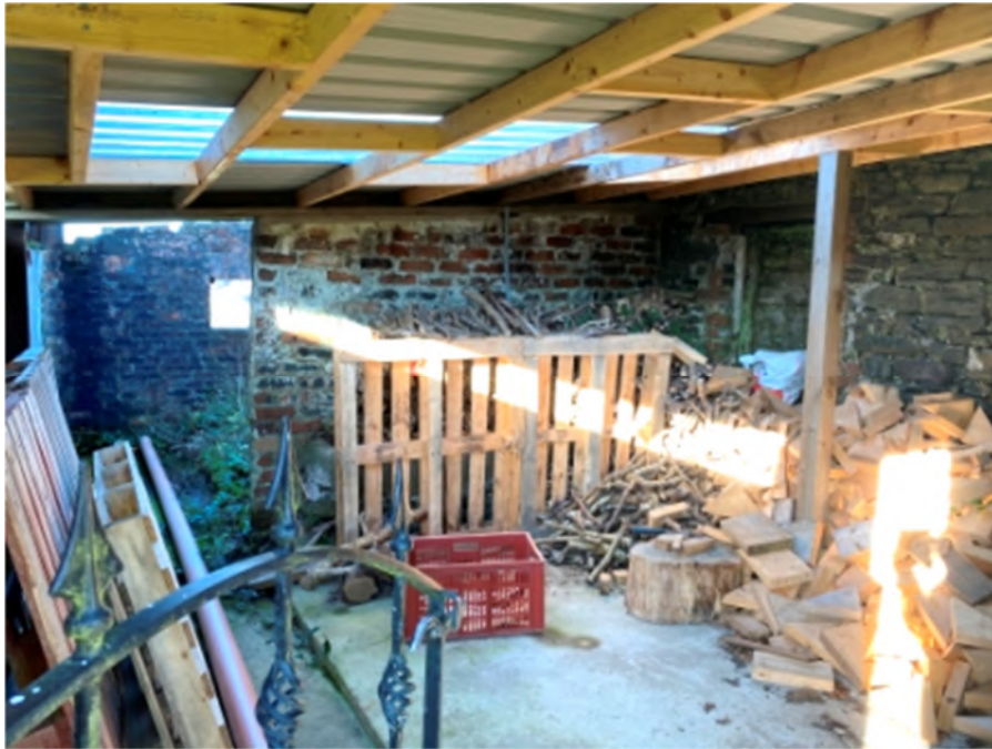
Photograph 27: Internal view of lightweight timber roof structure and profiled metal sheet cladding over cow shed.
