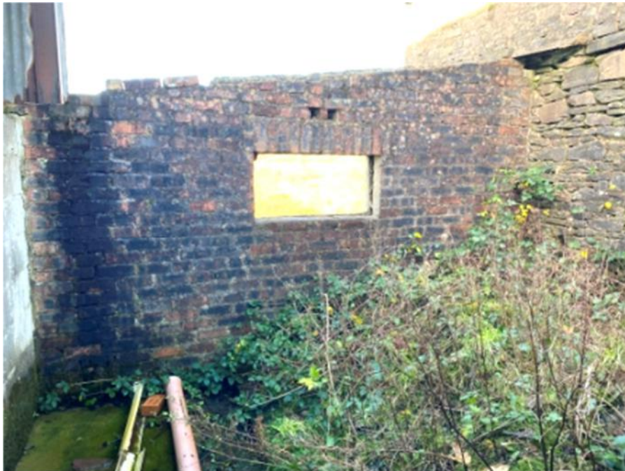
Photograph 28: Internal view of cow shed west elevation brick wall. No window or roof covering.
