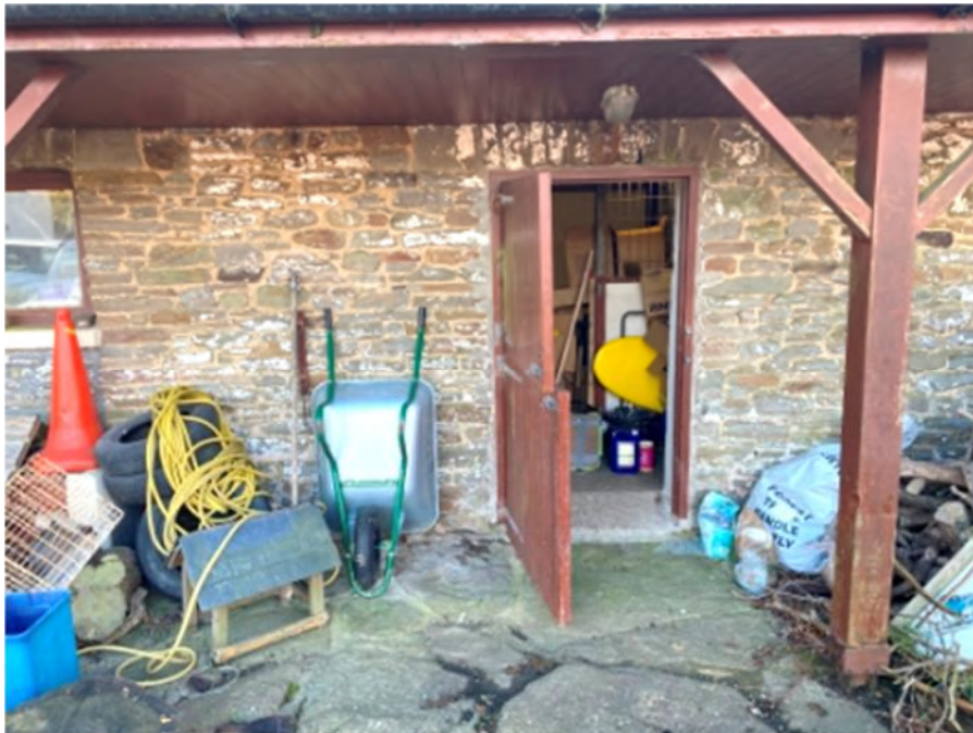
Photograph 36 : Part view of barn north elevation (courtyard). No cracking noted.
