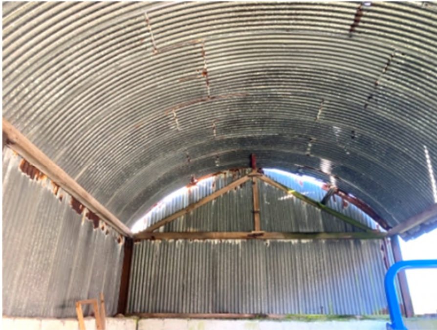
Photograph 21: Internal view of Dutch barn. Timber structure supports corrugated steel sheeting, above blockwork walls. Roof relies on diaphragm action of metal sheeting with no roof support members.
