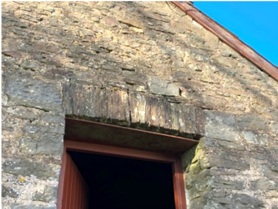
Photograph 32 : View of stone soldier course over first floor opening in barn east gable elevation.
