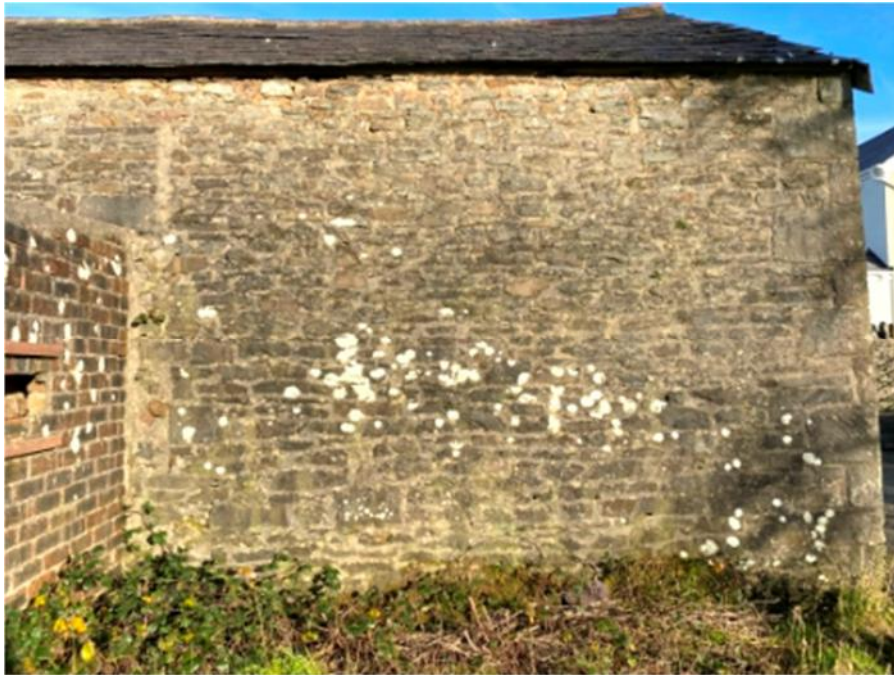
Photograph 31 : View of barn south elevation at south east corner. All stonework is in good condition.
