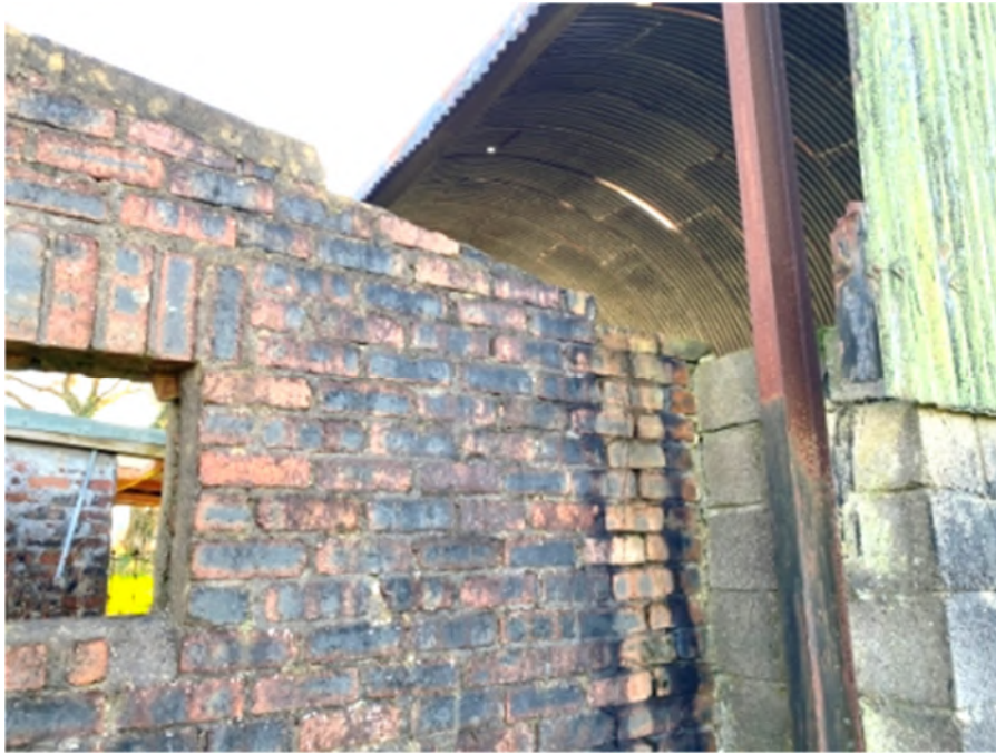
Photograph 13: View of junction between cow shed and Dutch barn on west elevation.
