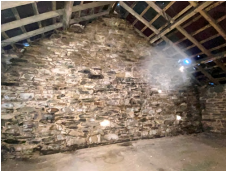
Photograph 42 : Internal view of west gable elevation wall. Wall is in a stable condition.
