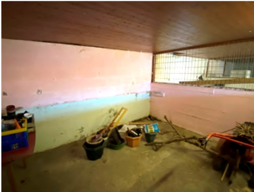
Photograph 48: Internal view of south elevation barn wall shows an inner skin of concrete blockwork. No cracking or structural movement is noted to the blockwork construction.
