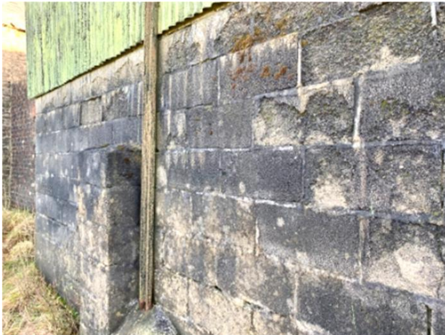
Photograph 14: View of blockwork construction on west gable elevation of Dutch barn.
