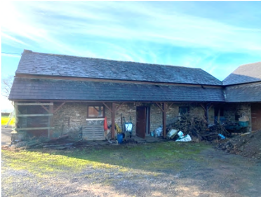
Photograph 1: View of courtyard north elevation of barn at Cilmaengwyn Uchaf Farm with mono-pitch canopy roof structure.
