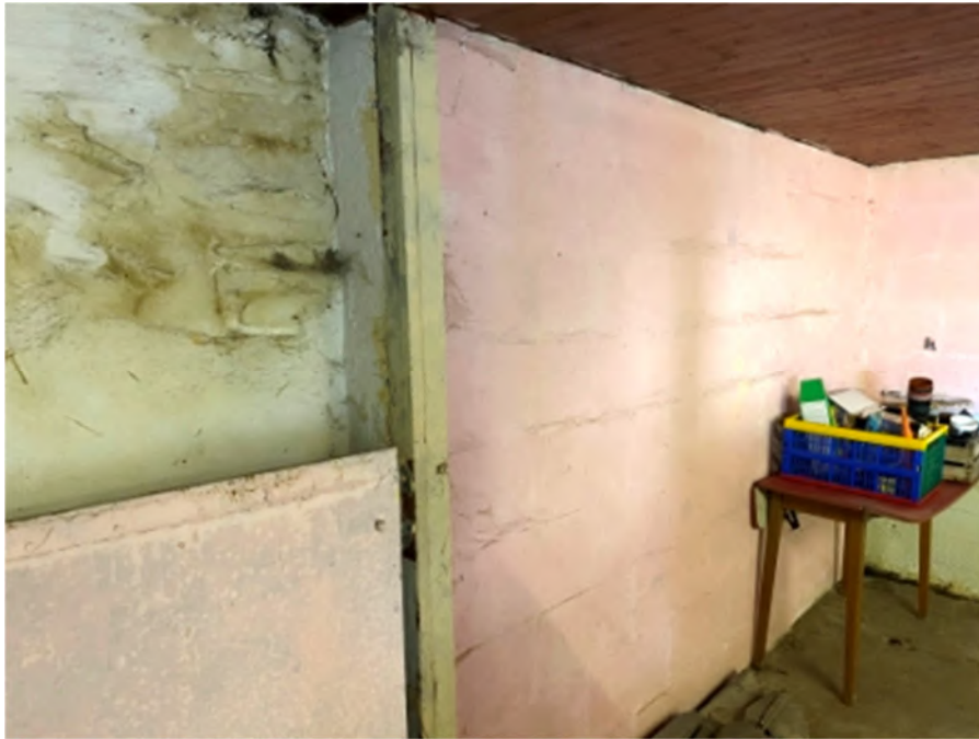
Photograph 51: View of inner block skin which exists along the south, east and west elevations.
