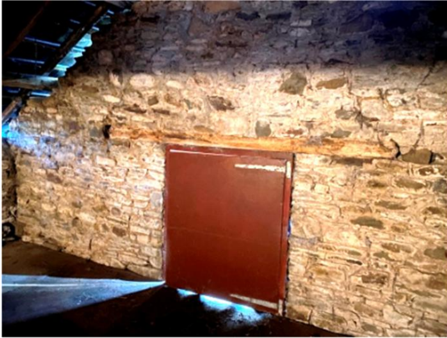
Photograph 39 : Internal view of barn east elevation. No cracking or structural movement noted.
