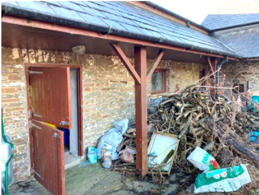
Photograph 52: Timber posts with diagonal bracing support a mono pitch timber canopy structure along the north courtyard elevation.
