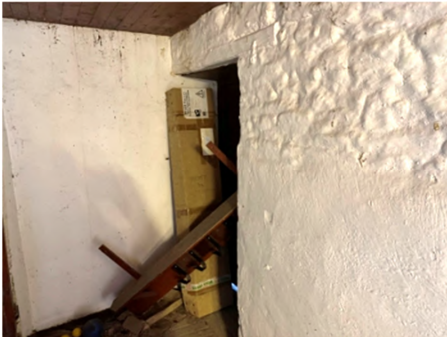
Photograph 50 : Single door opening exists in the north west corner, allowing access into the next adjacent barn building.
