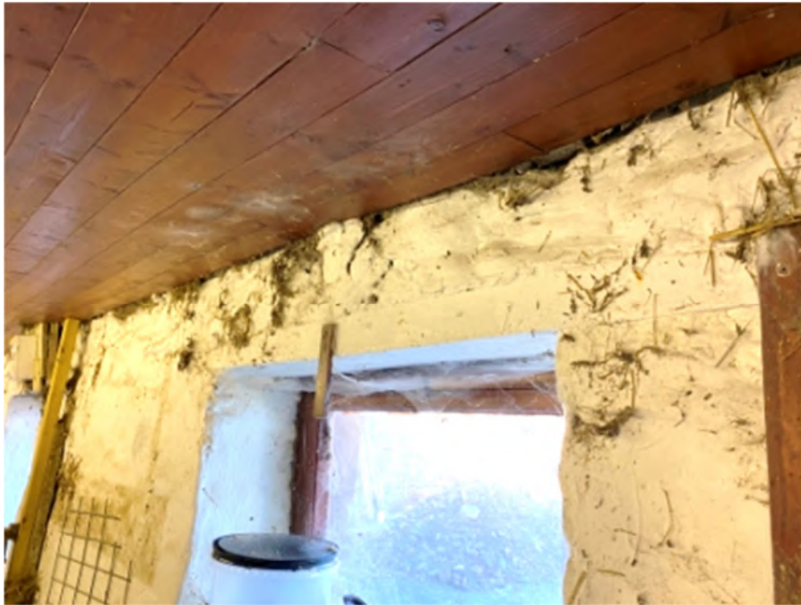
Photograph 49 : Inner timber lintels along the north elevation appear in good condition.
