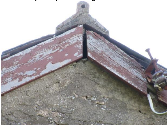
Plate 11: Gaps between wall and roof feature
