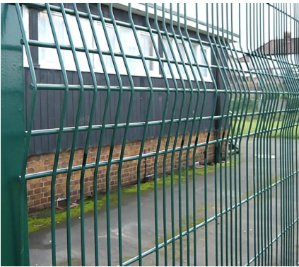
External refrigeration plant cage (Adjacent to Customer Parking) - Paladin fencing
