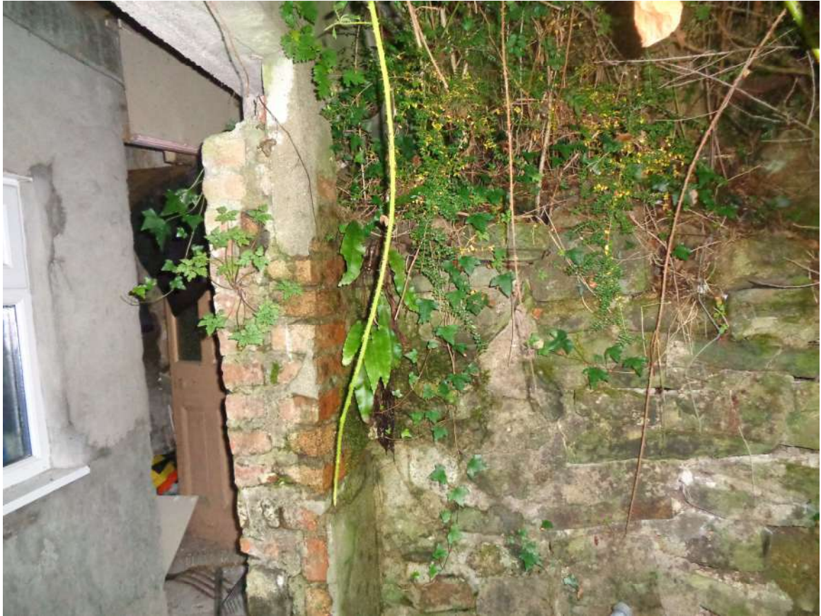
Photograph 3 – Rear elevation facing retaining wall.
