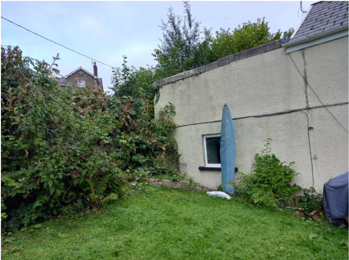
Photograph 1 – Front Elevation (viewed from front garden).
