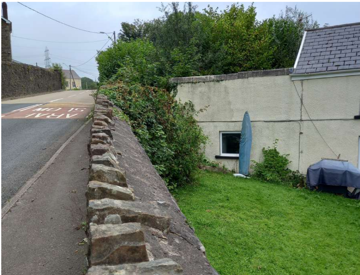
Photograph 2 – Front Elevation (viewed from public footway).
