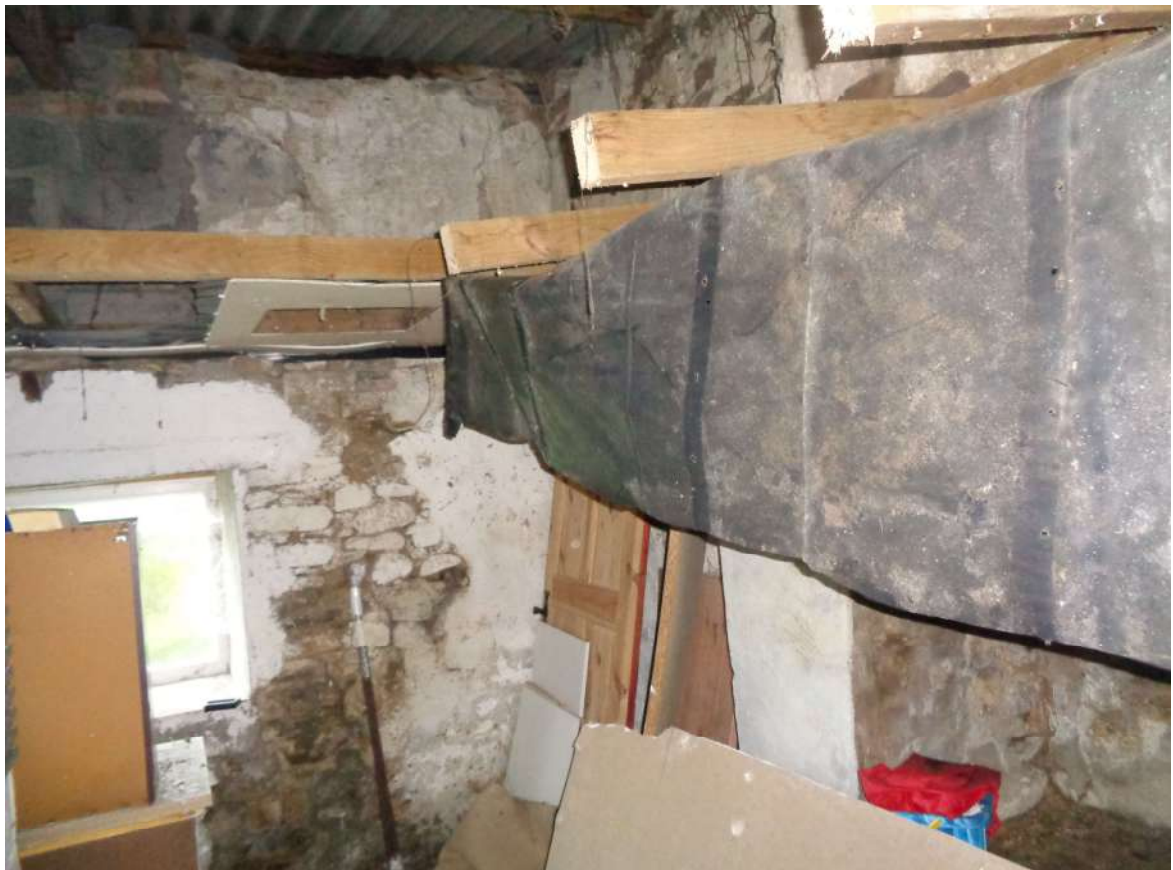
Photograph 4 – Internal view facing side and front wall.
