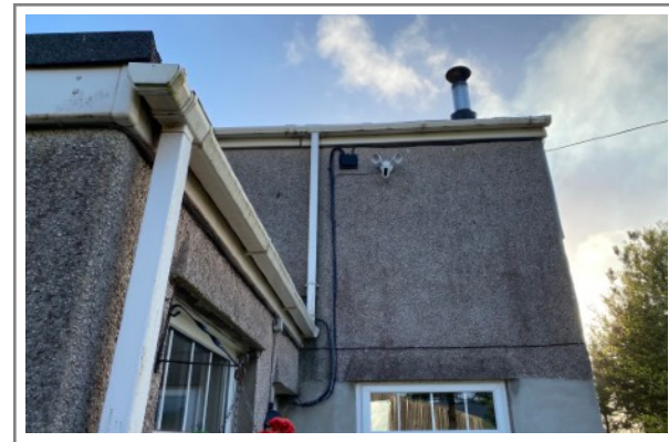
Photo 7: Main east facing elevation with no gaps for bat access behind fascia boards
