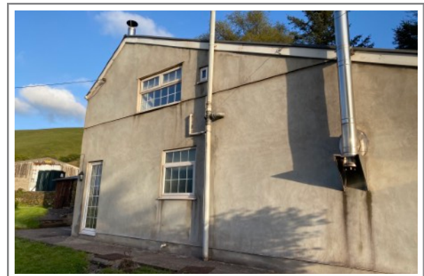
Photo 4: North facing elevation
