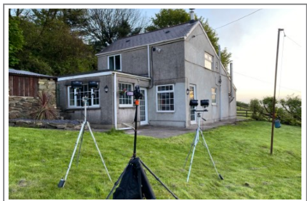
Photo 10: Infra red camera set up
