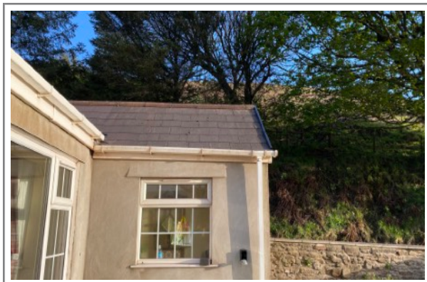
Photo 3: North and west elevations with mature trees to the south
