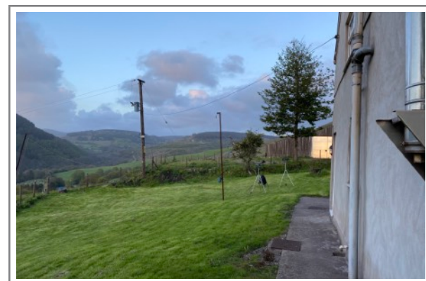
Photo 9: View of the north facing elevation looking east towards Cwm Dyffryn
