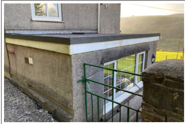
Photo 5: Flat roof over the kitchen at the east side of the property
