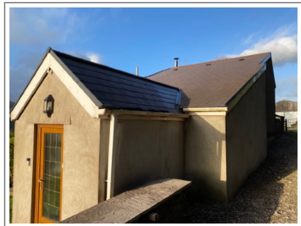
Photo 2: South and west elevations
