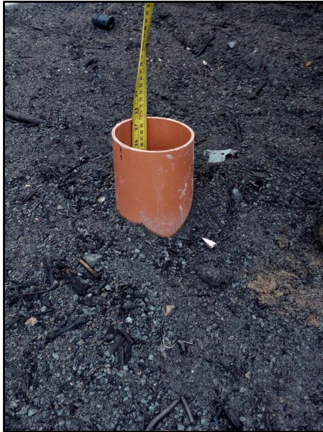
Plate 01 & 02. Capping Soils and Barrier at >600mm bgl.
