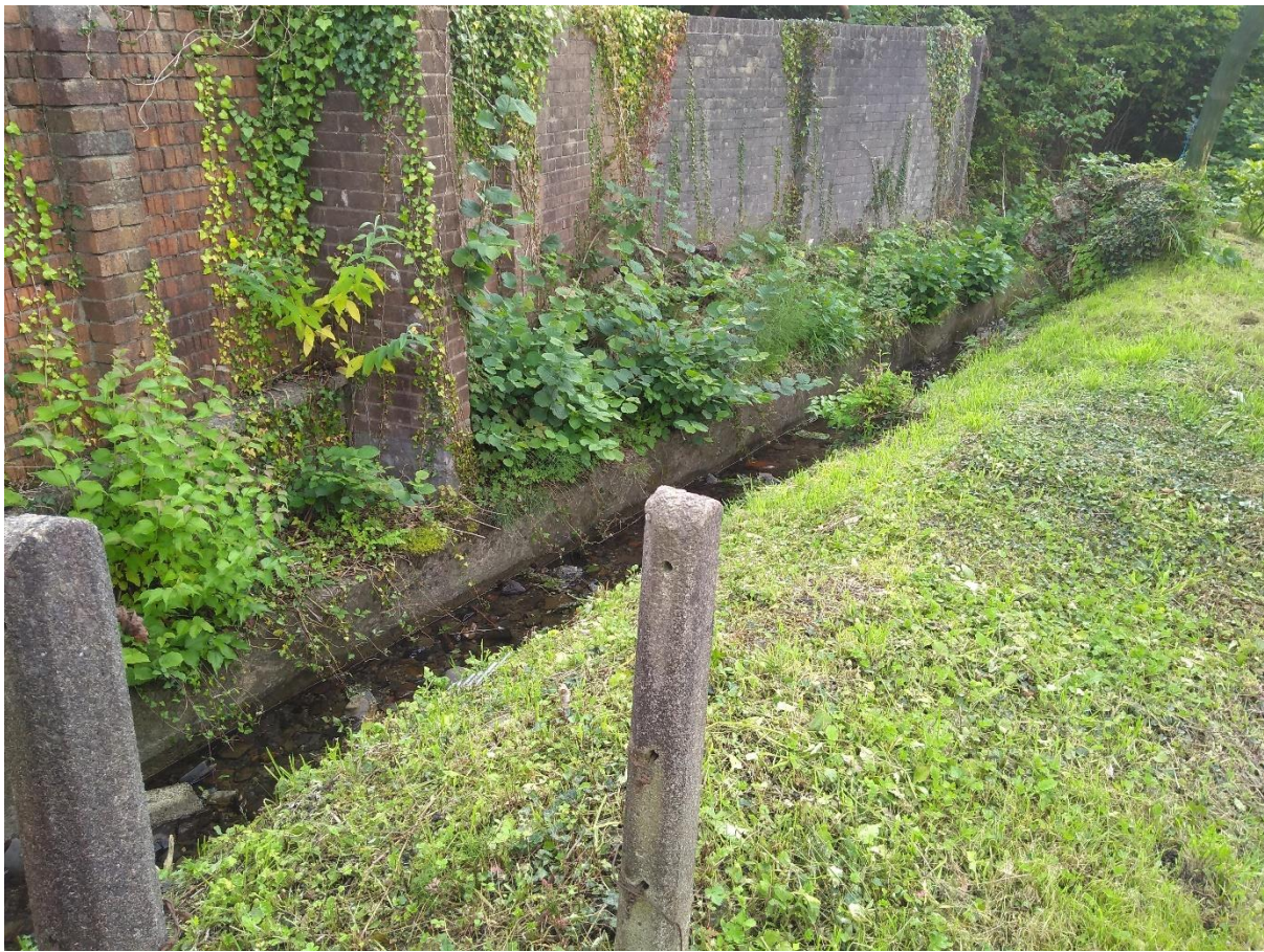
Picture 2 – Open culvert adjacent to the parkland.
