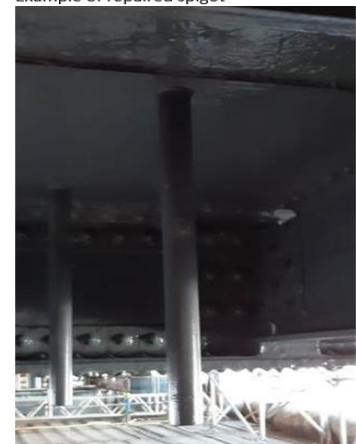
Example of repaired spigot
