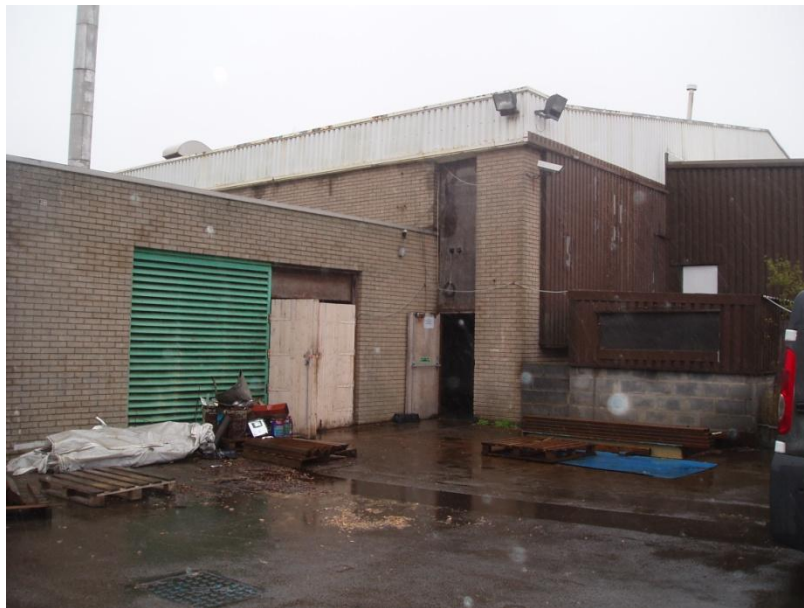
The two buildings looking from the south
