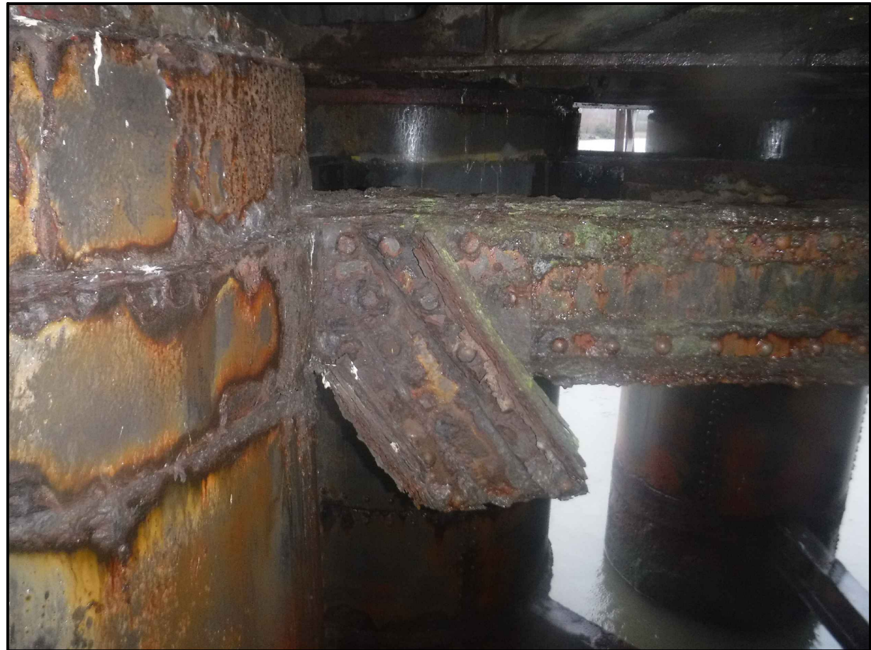
CUT BRACING IN CLUSTER PIER ARRANGEMENT
