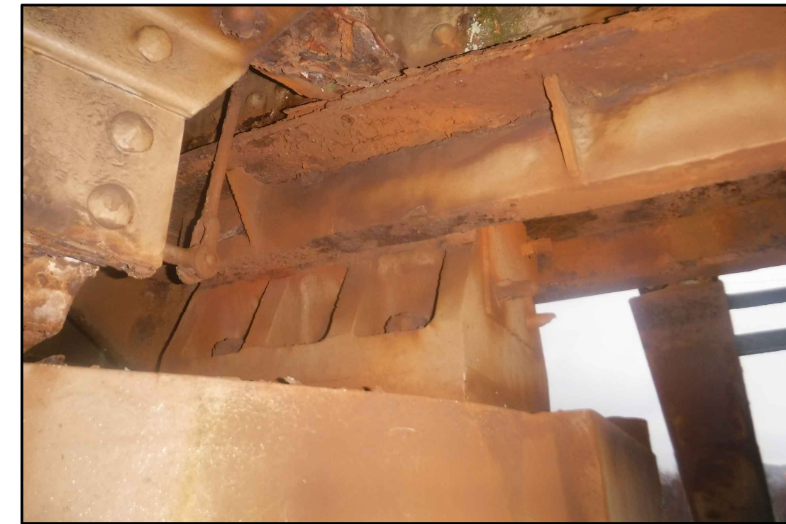
- PHOTO 1 - SHOWING SLIDING BLOCK
