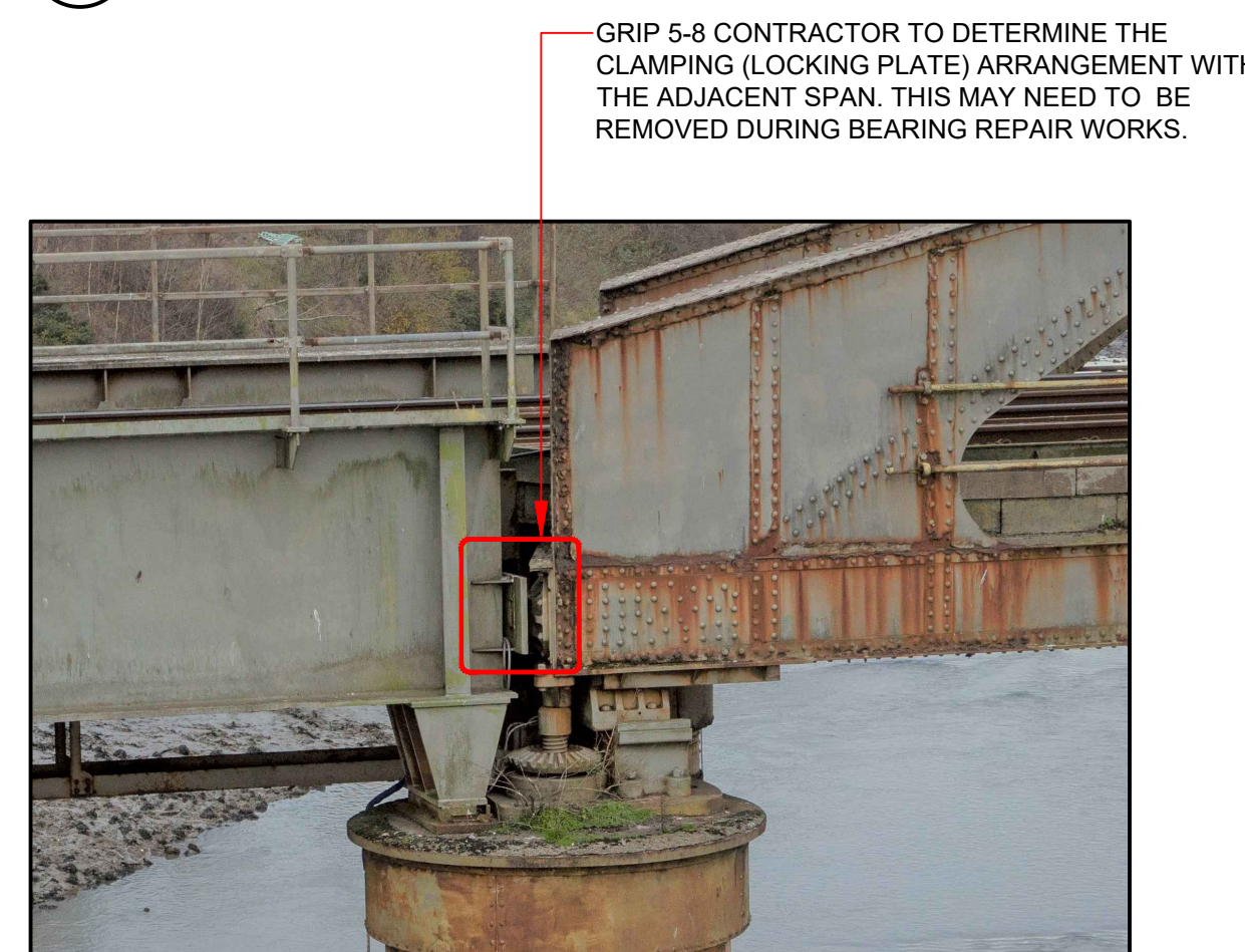
- PHOTO 2 - ELEVATION OF SWING SPAN BEARING
