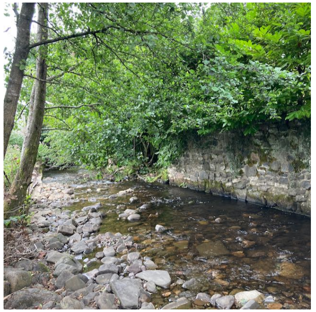
Figure 4. Stone wall to the north, on the western bank.
