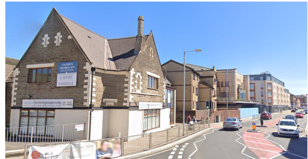
View of the site looking South down Talbot Road.
