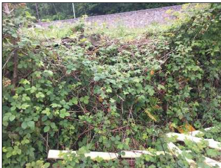
Fig. 7. Section of stone wall behind Bramble cover
