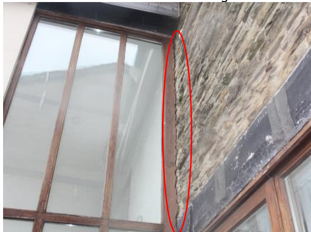
Photo 28: Gap Between the Timber Feature and External Wall on Commercial Building
