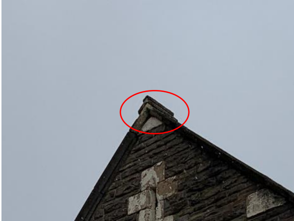
Photo 13: Lifted Ridge Tile Adjacent to South Western Gable End
