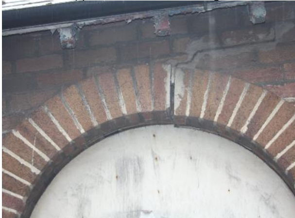
Photo 21: Slipped Arch on Outbuilding
