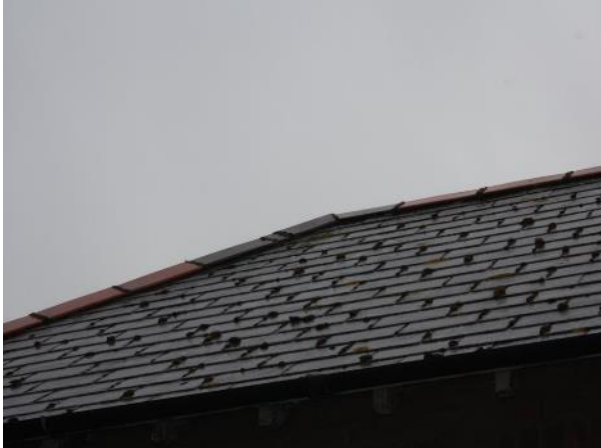
Photo 15: Lifted Hip Tiles on South Eastern Elevation of Outbuilding
