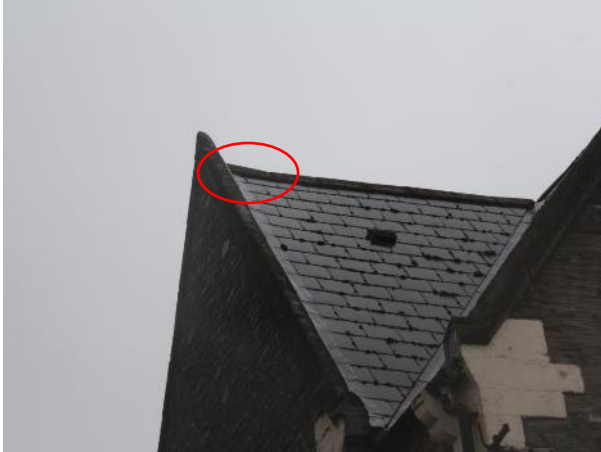
Photo 15: Lifted Hip Tiles on South Eastern Elevation of Outbuilding
