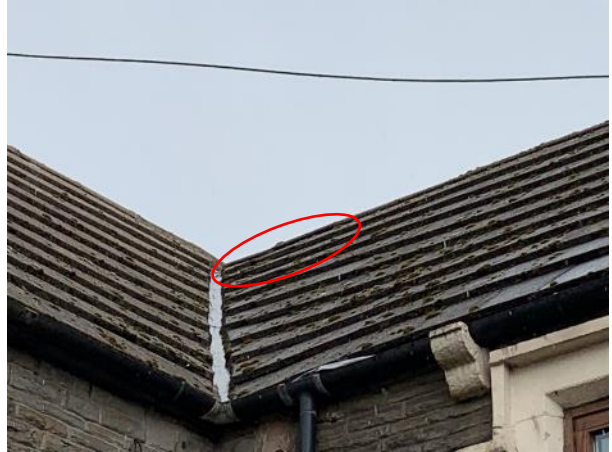
Photo 14: Slipped Tile on Outbuilding
