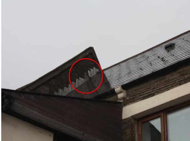
Photo 19: Lifted Lead Flashing on External Wall
