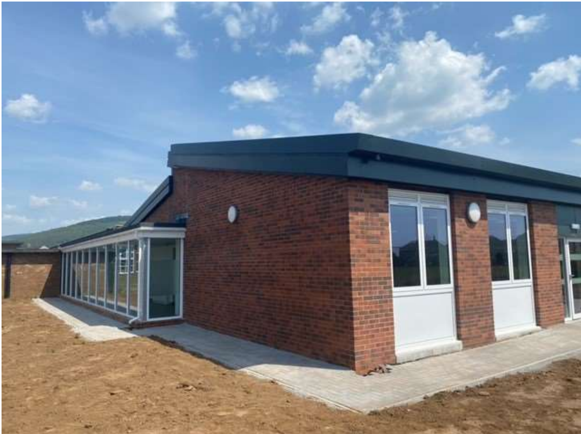
Corner of South West Elevation
